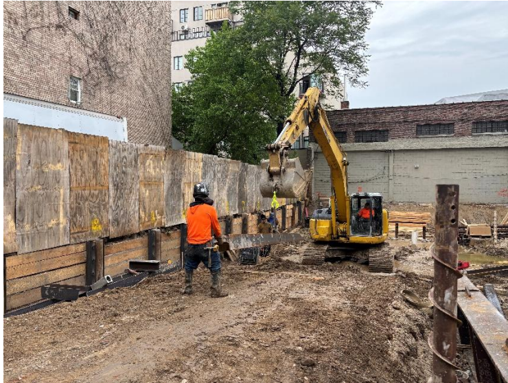
Photo 1: View of contractors placing and welding steel beams, facing north.
