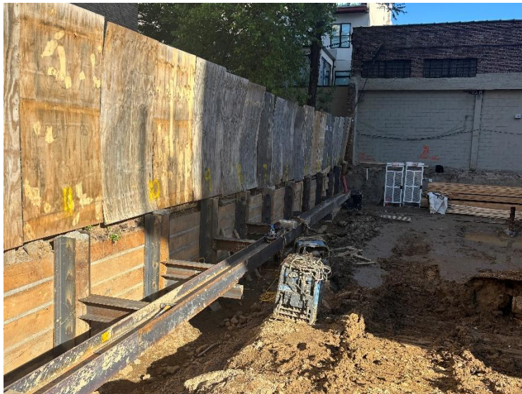
Photo 2: View of contractors welding steel beams, facing north.
