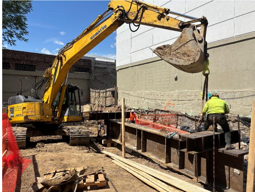
Photo 1: View of contractors setting up load test, facing north.
