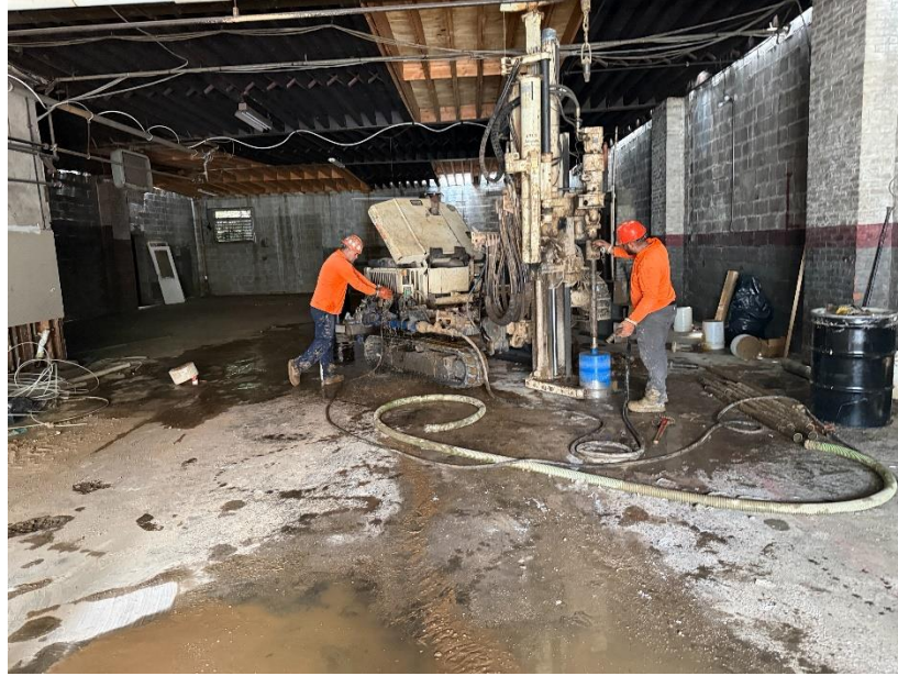
Photo 1: View of AARCO advancing a soil boring for SVE monitoring point VP-04 (facing south).
