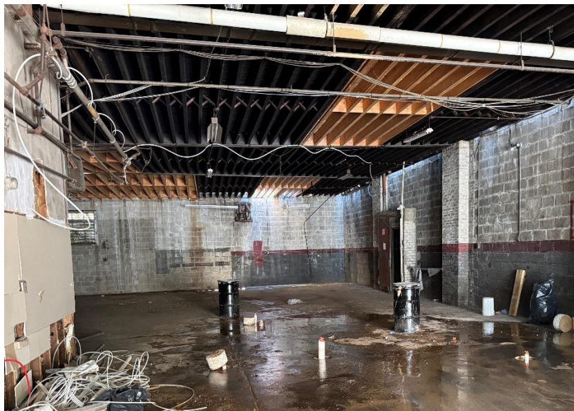
Photo 2: General view of the site (facing south).
