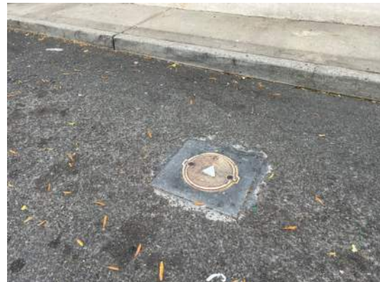
VIEW OF A MONITORING WELL NOTED ON SITE AT 456-460 BUSHWICK AVENUE
