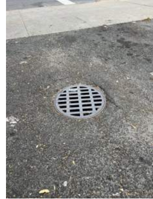
VIEW OF A DRYWELL NOTED ON SITE AT 456-460 BUSHWICK AVENUE
