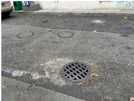
VIEW OF A DRYWELL NOTED ON SITE AT 456-460 BUSHWICK AVENUE (2)
