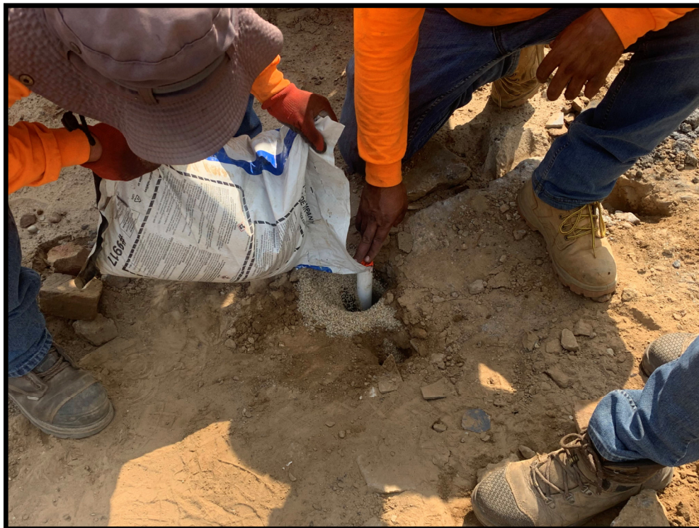
View of #2 sand being used to fill the annular space of the temporary groundwater monitoring well boring.
