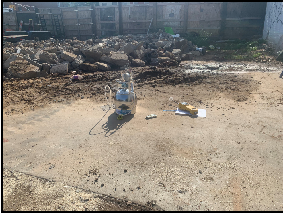
View of soil vapor sample SV-2 being collected.
