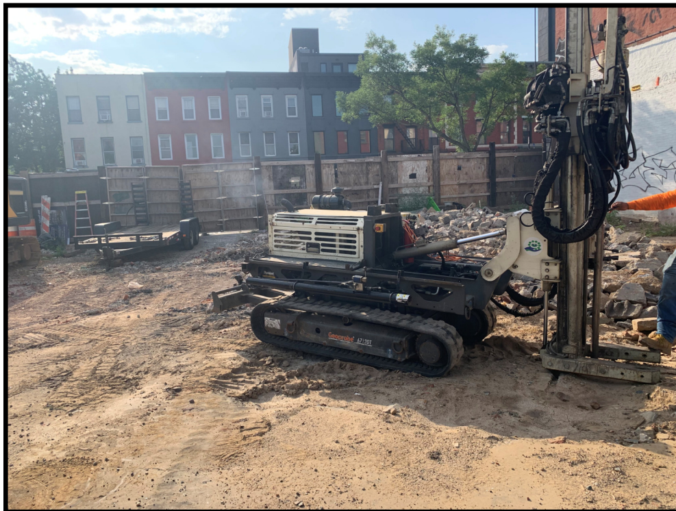
View of drilling being conducted by PGES at the Site.
