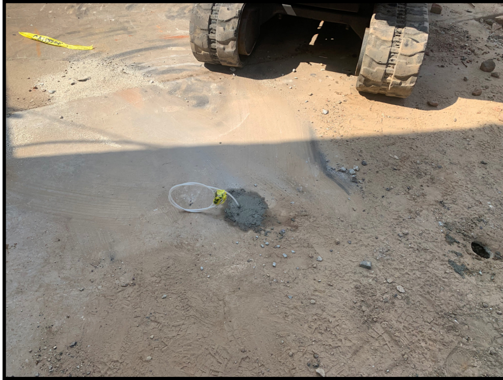
View of the soil vapor point after being finished with bentonite to ground surface.
