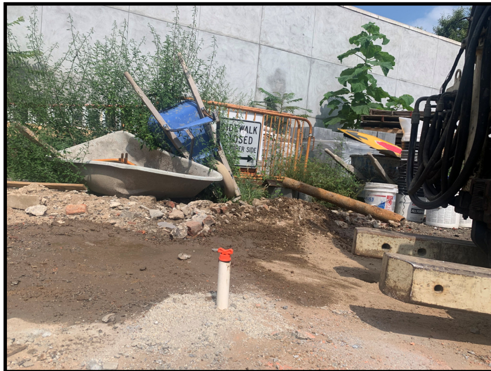
View of temporary groundwater monitoring well TW-2 after being installed.
