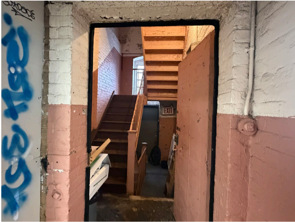
Photograph 5: View of the basement doorway leading to the stairwell. Date: October 17, 2025
