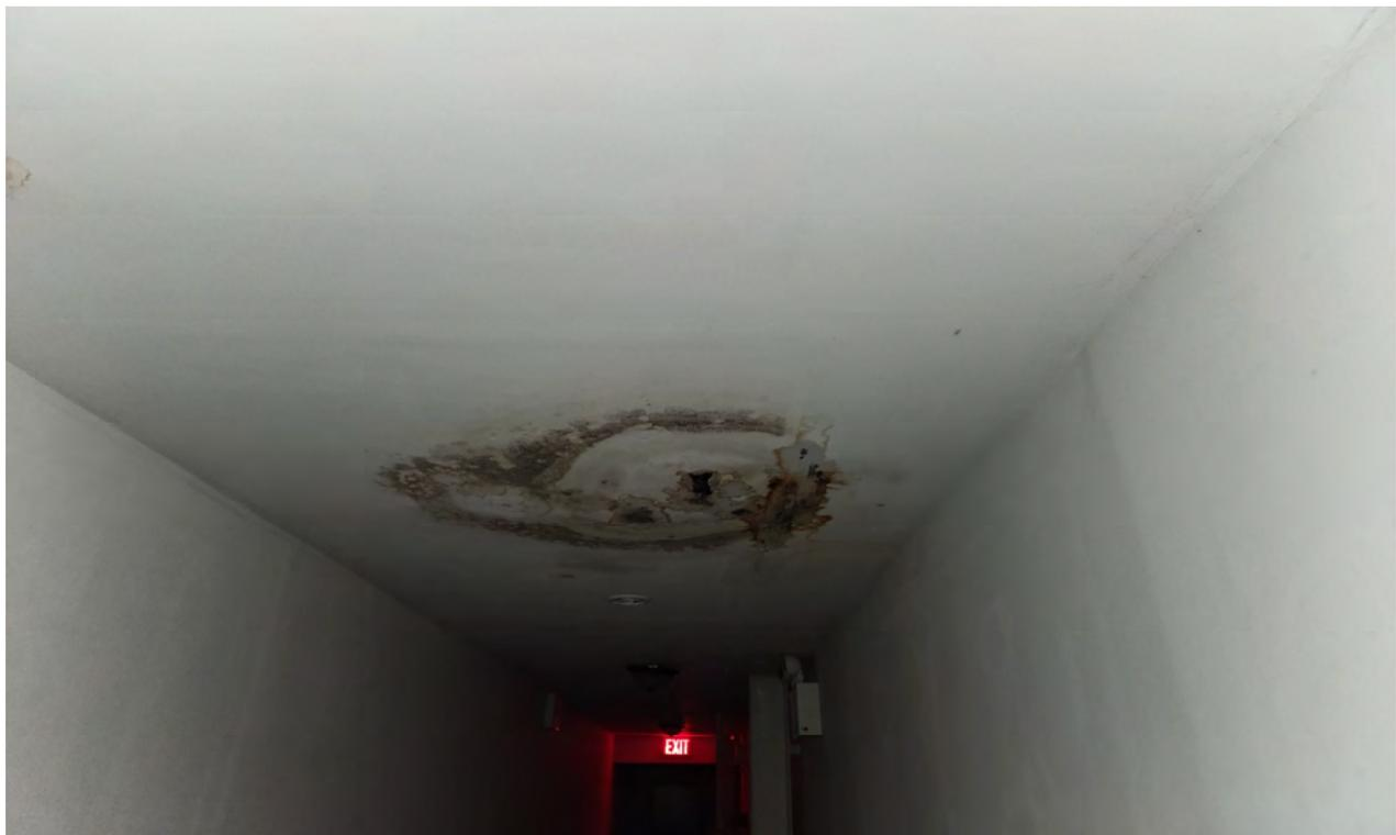
**View of water-staining on the 2<sup>nd</sup> floor ceiling.**
