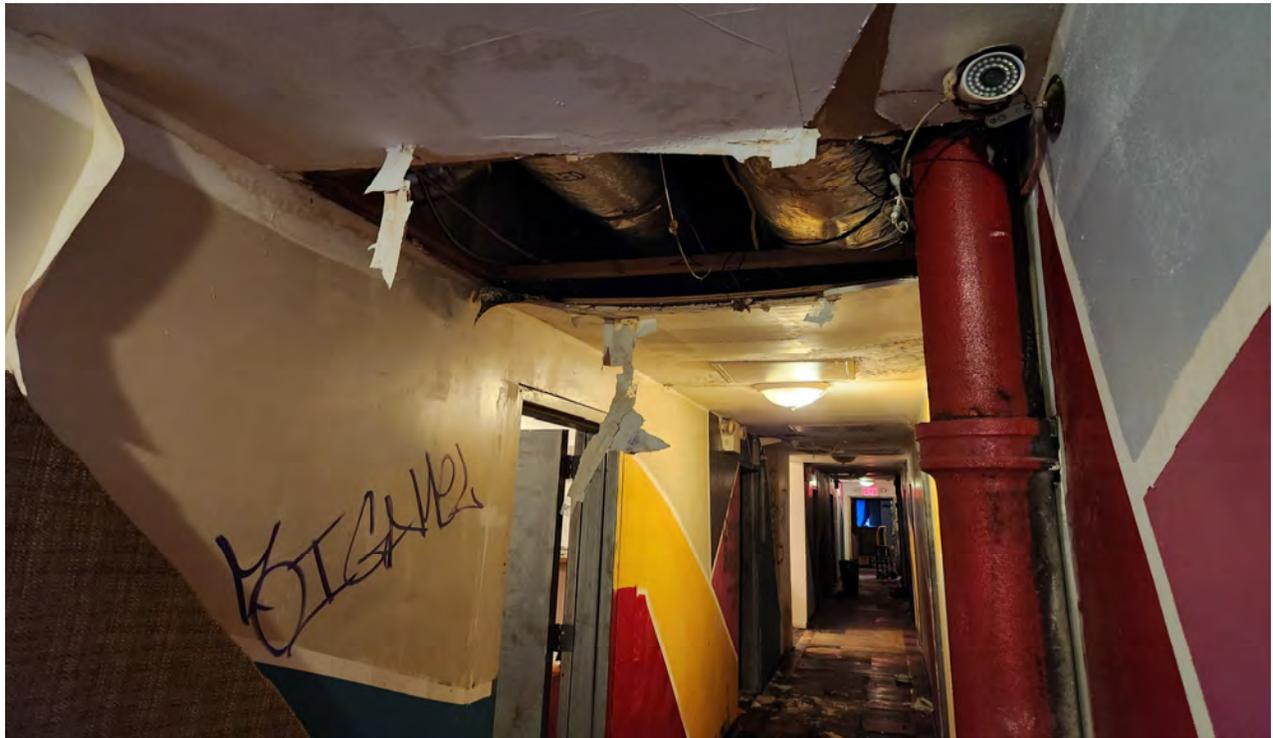
**View of water damaged sheetrock (2<sup>nd</sup> floor ceiling).**
