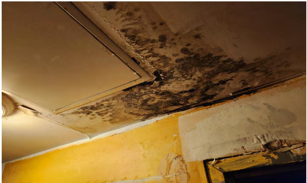
**View of water damage and visible mold growth (2<sup>nd</sup> floor ceiling).**
