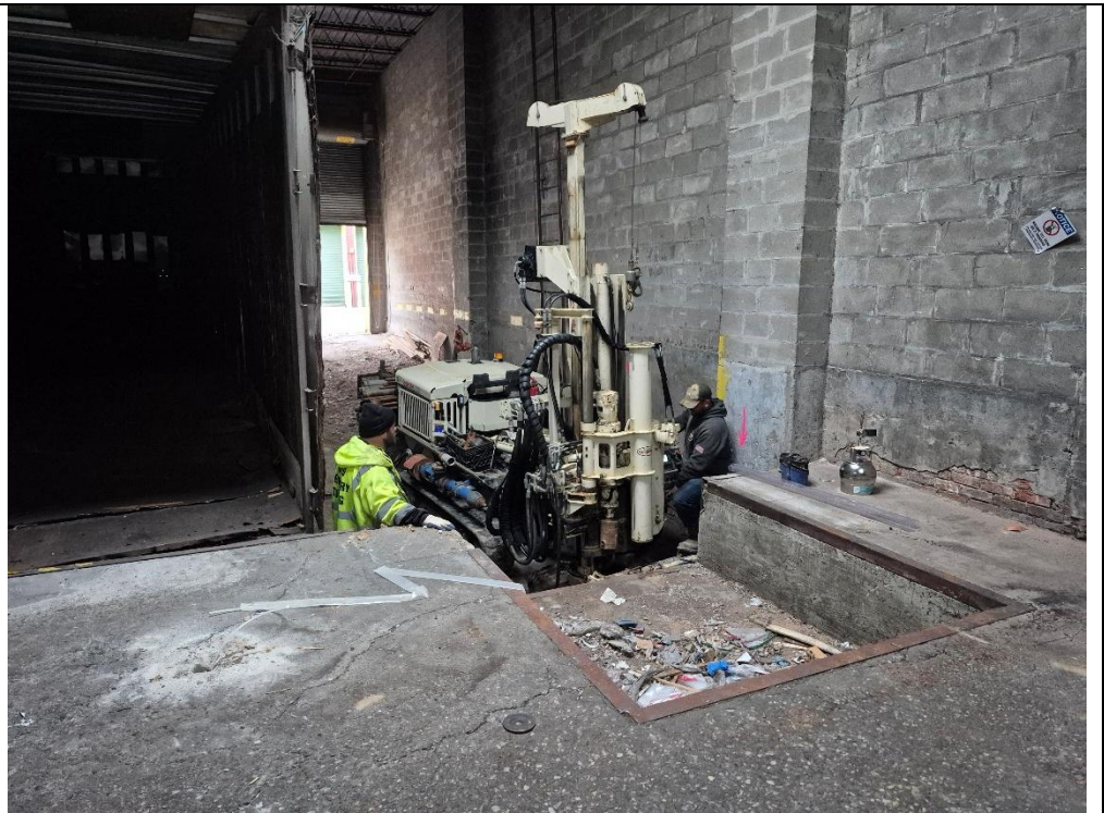
Photo 1: View of soil boring installation utilizing Geoprobe 7822DT.
