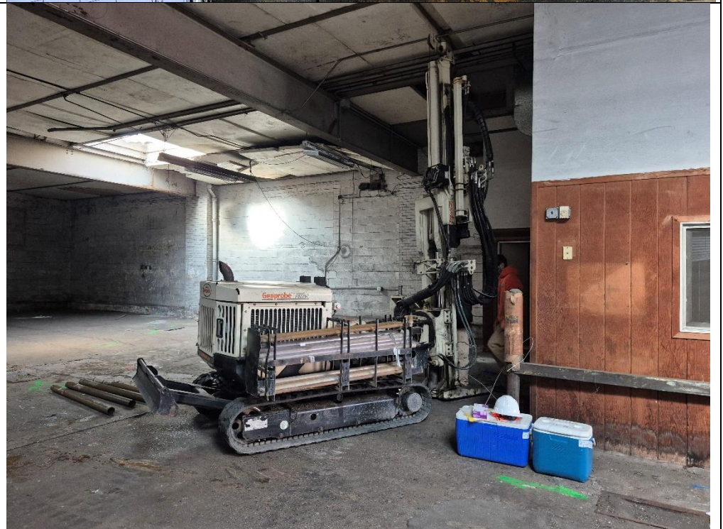
Photo 2: View of drilling utilizing Geoprobe 7822DT.
