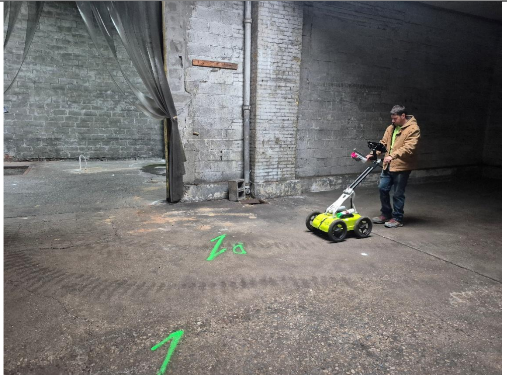
Photo 1: View of the GPR being performed.
