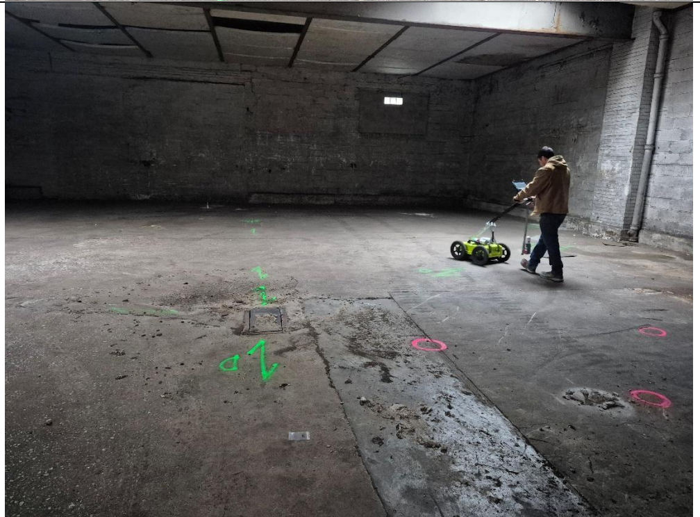
Photo 2: View of GPR being performed and marked out floor drains and utilities.
