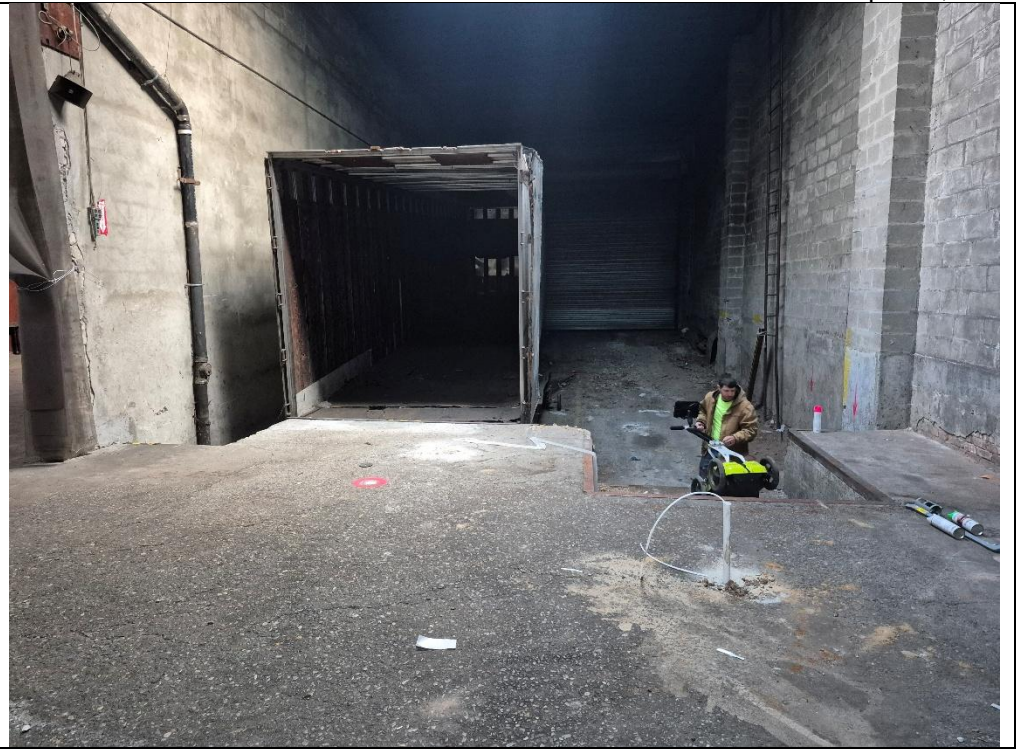
Photo 3: View of empty trailer in loading bay with MW-3 in foreground.
