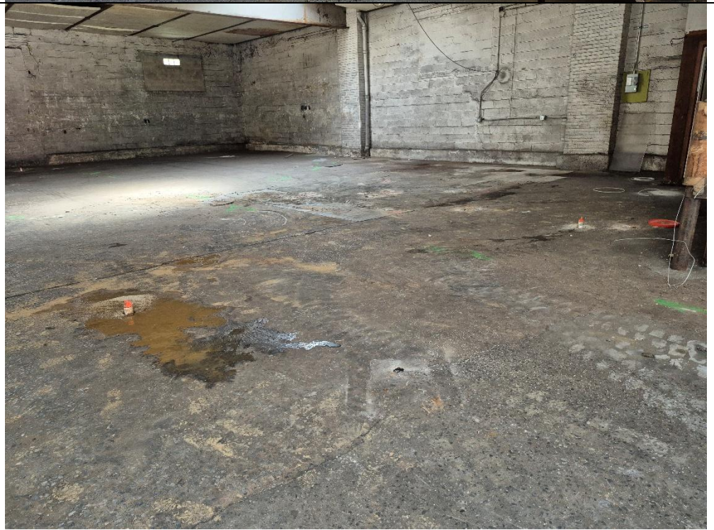
Photo 4: View of installed MW-6 and MW-7.
