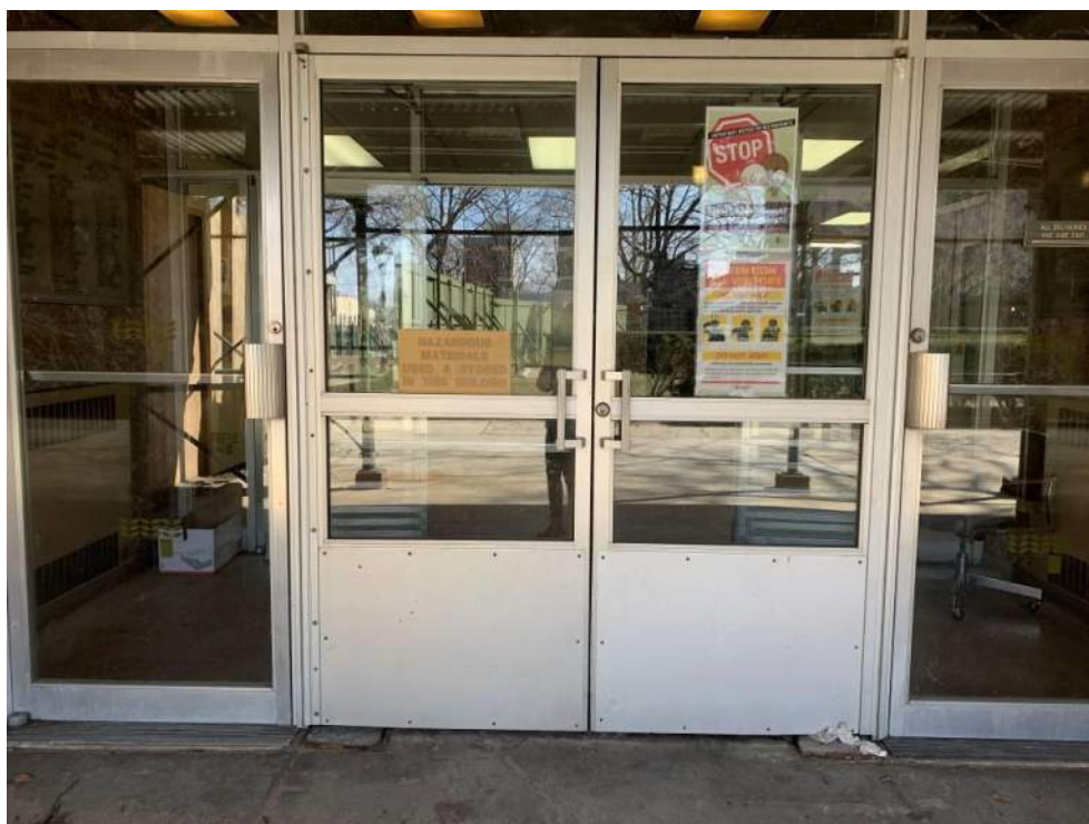
Photograph 18: View of entrance to the Masin building from courtyard (facing east).
