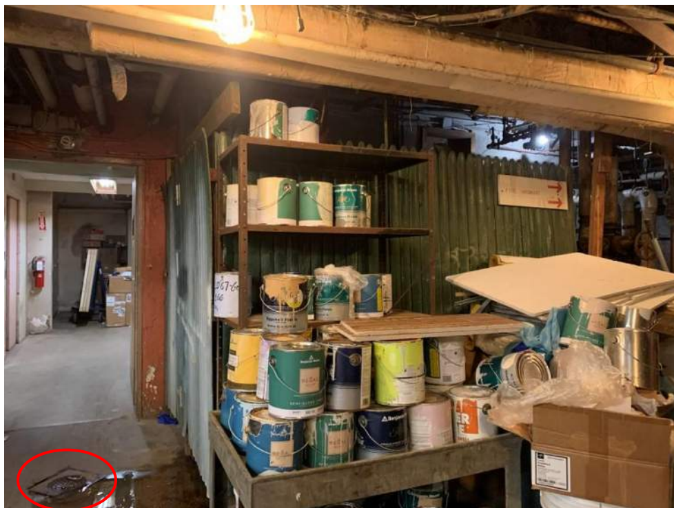
Photograph 9: View of paint storage and floor drain in maintenance area of Blumberg building cellar (facing northeast).
