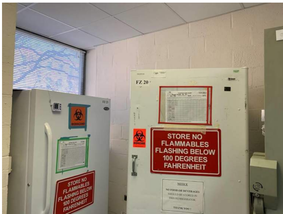
Photograph 28: View of biological freezers in freezer storage room on third floor of the Masin building (facing northwest).
