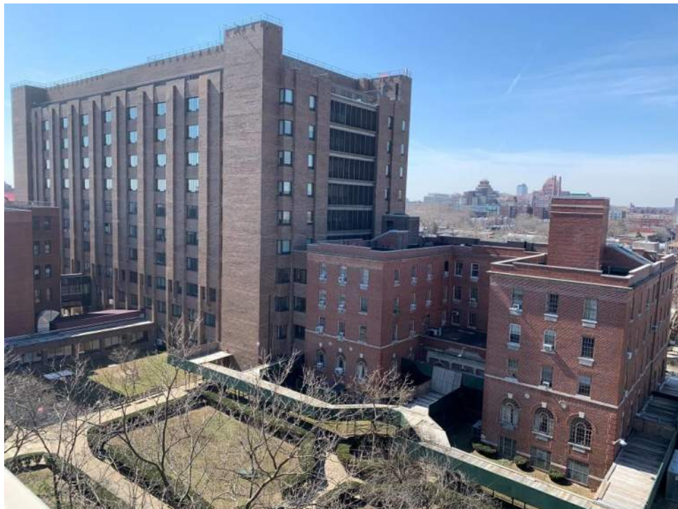
Photograph 33: View of courtyard and Leviton building from roof of the Masin building (facing west).
