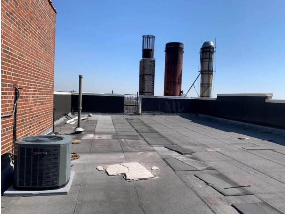
Photograph 15: View of flue gas stacks and steam column from roof of Blumberg building (facing east).
