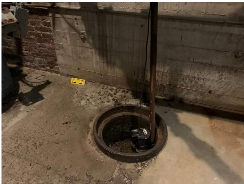
Photograph 36: View of sump in the boiler room of the Leviton cellar (facing east).
