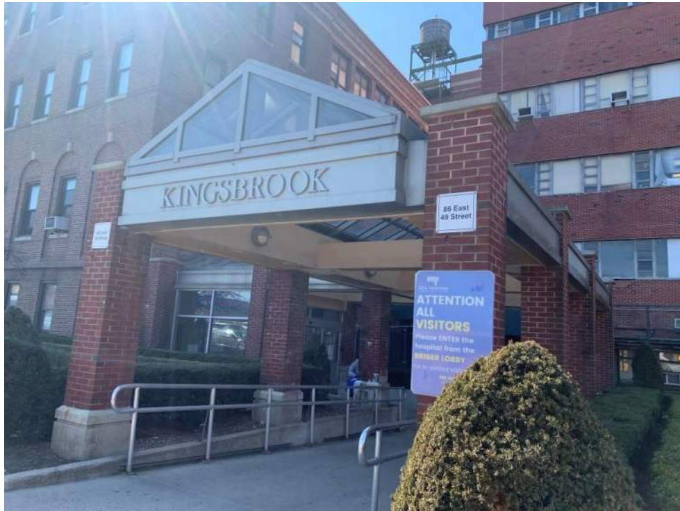
Photograph 1: Entrance to the LeFrak building on East 49 th Street (facing southwest).
