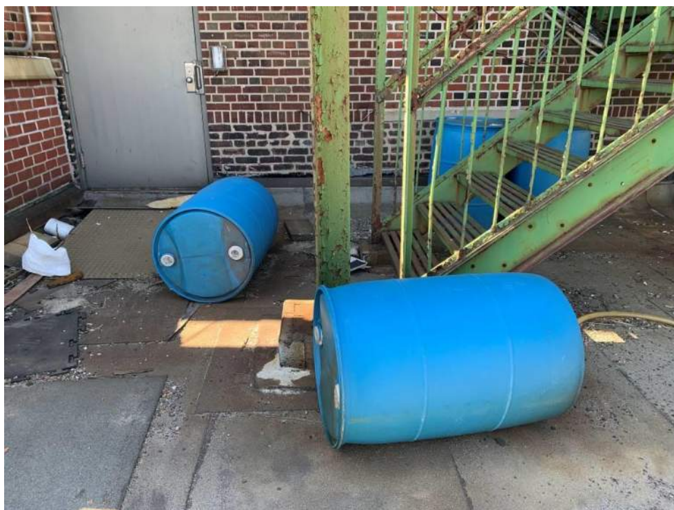
Photograph 6: View of plastic 55-gallon drums on the roof of the LeFrak building (facing west).
