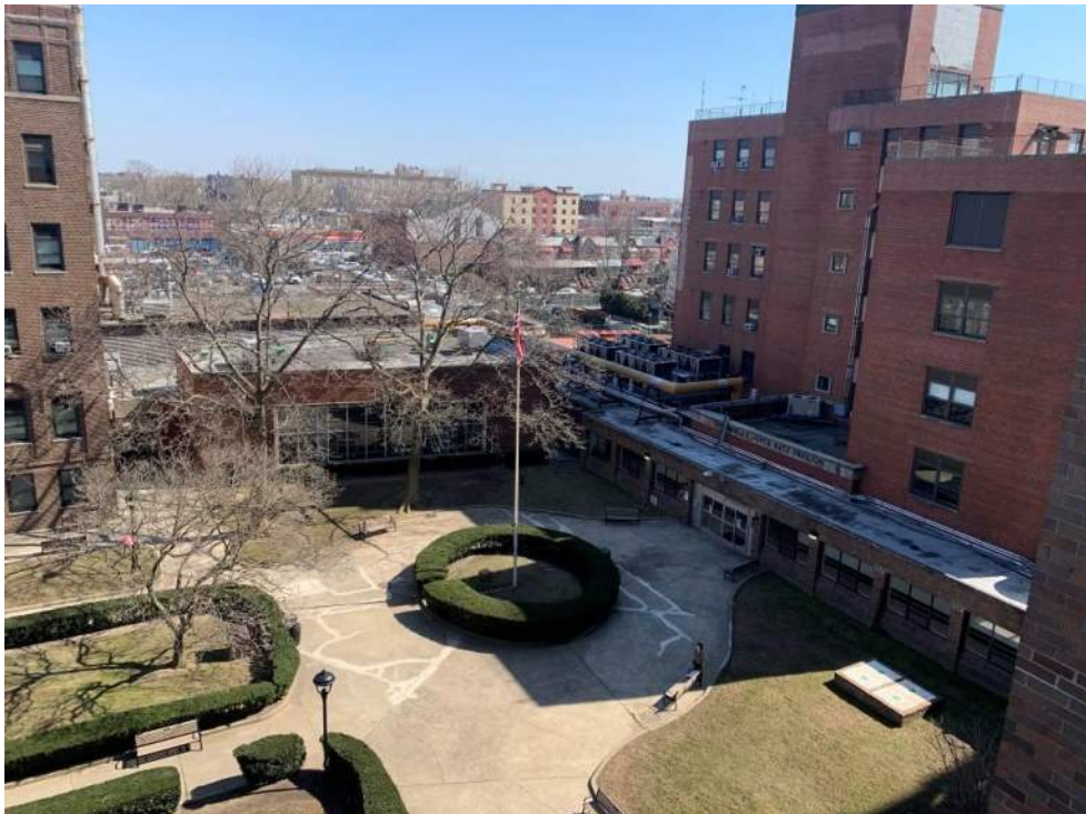
Photograph 40: General view of southern boundary of the Subject Property (facing west).
