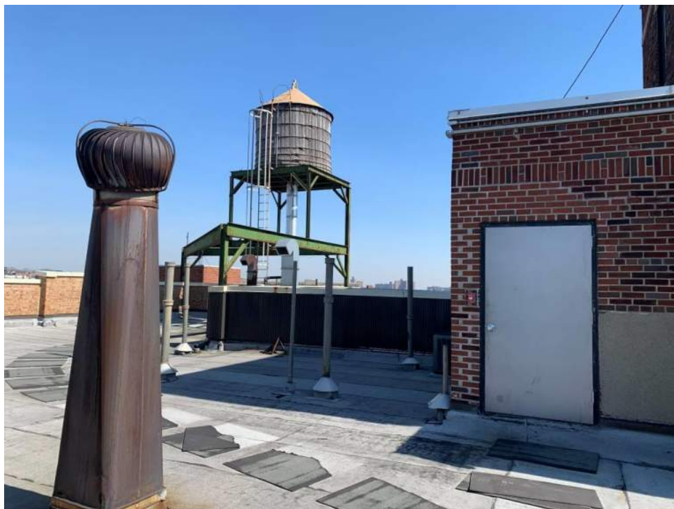
Photograph 14: View of water tank on roof of Blumberg building (facing northeast).
