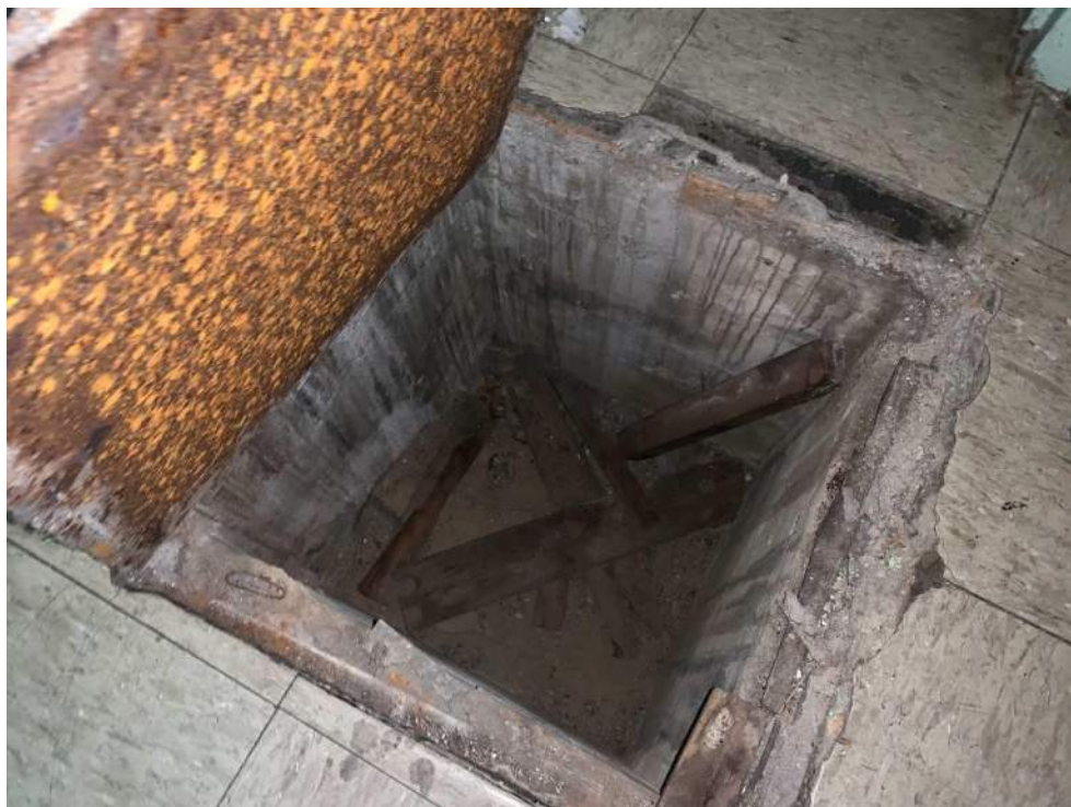
Photograph 34: View of sump pit in cellar of the Leviton building (facing west).
