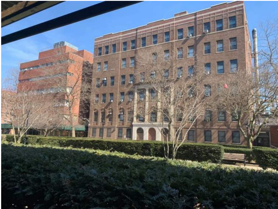
Photograph 7: View of the Blumberg and Masin buildings from courtyard (facing northeast).
