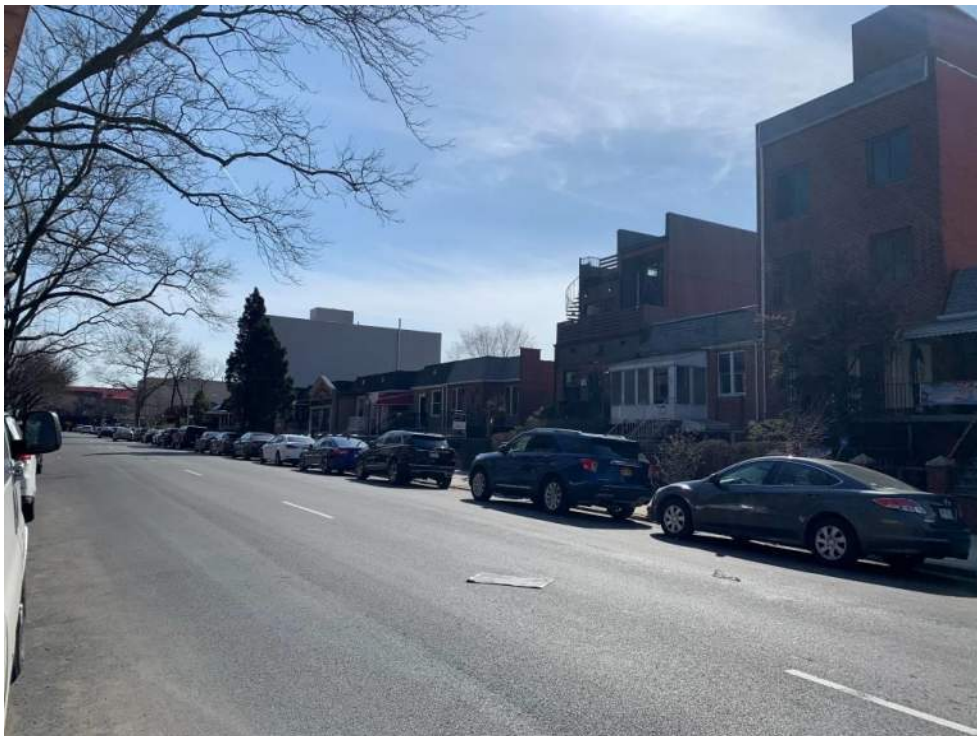
Photograph 46: View of western-adjointing multi-family residential buildings on Schenectady Avenue (facing southwest).
