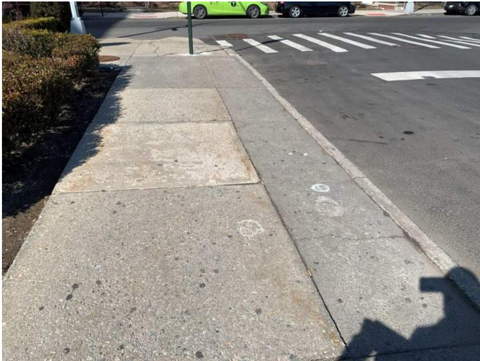
Photograph 43: View of patched concrete in potential borehole locations on sidewalk near the LeFrak building entrance (facing north).
