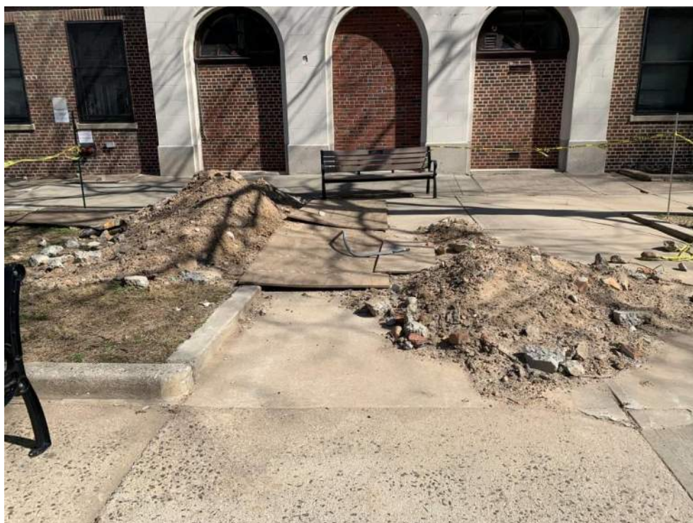
Photograph 38: View of stockpiled soil in the courtyard outside of the Blumberg building (facing east).
