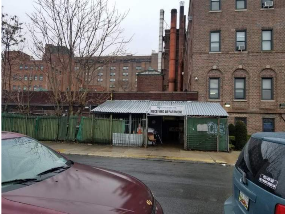
Photograph 29: View of the LeFrak Building (right), the southeastern adjoining building which contains three steam boilers from the eastern side of East 49 th Street (left, facing west).
