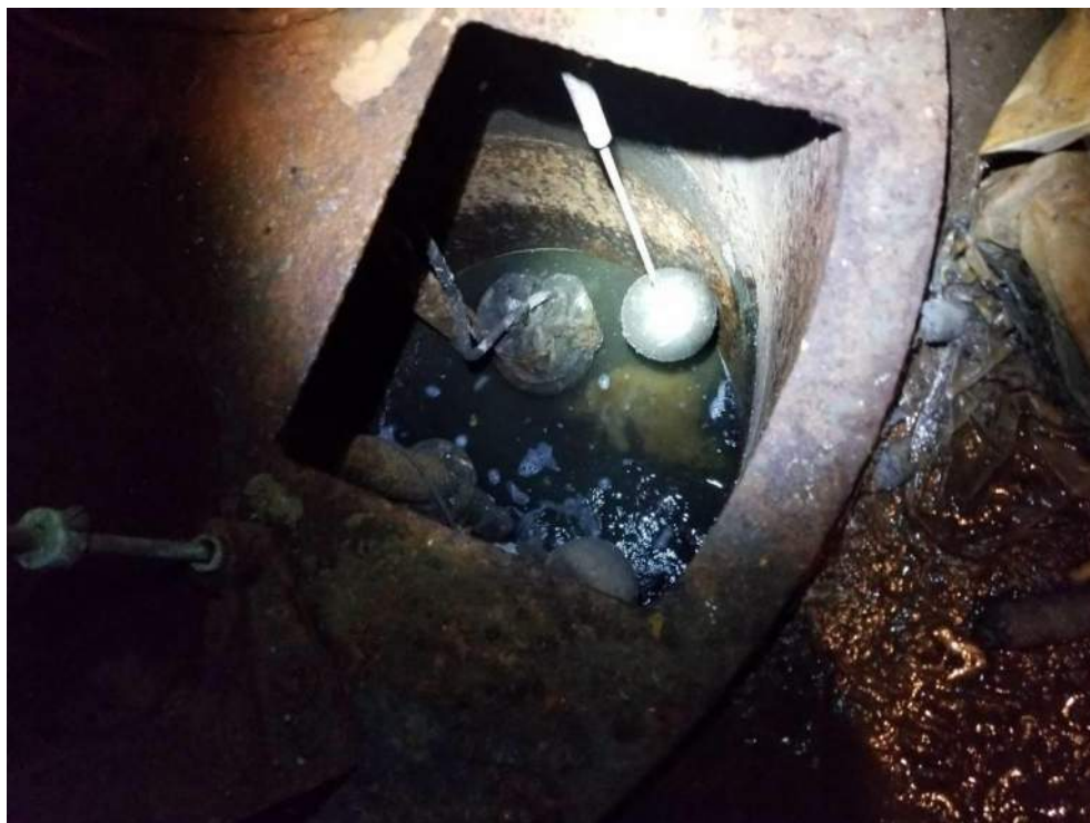
Photograph 20: View of sump pump in the former boiler room in the cellar of the Masin building (facing south).
