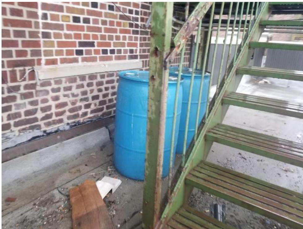
Photograph 27: View of two unlabeled plastic 55-gallon drums on the roof of the LeFrak building (facing north).
