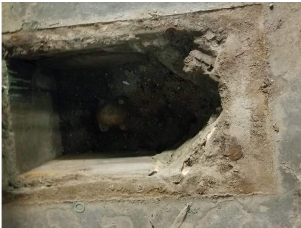
Photograph 23: View of sewer cleanout pit in the cellar of the Blumberg building (facing south).
