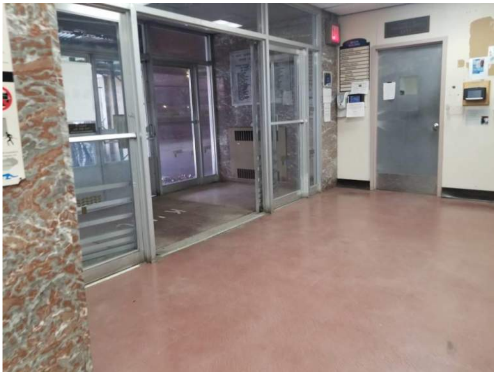
Photograph 17: Entrance foyer on the ground floor of the Masin building (facing northwest).
