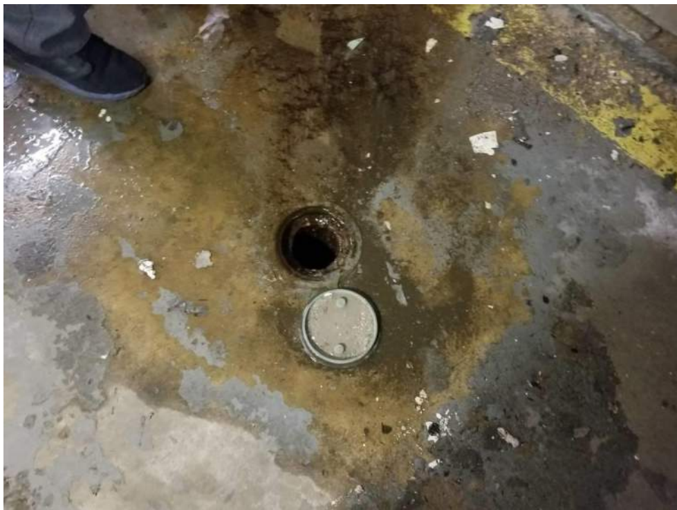
Photograph 15: View of a maintenance shop in the cellar of the Masin building (facing east).
