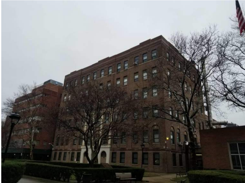
Photograph 3: View of the Blumberg building from the southern adjoining courtyard (facing northeast).
