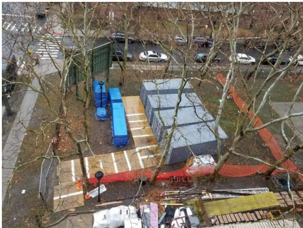
Photograph 11: View of façade restoration construction material storage adjoining the Leviton building to the north (facing north).
