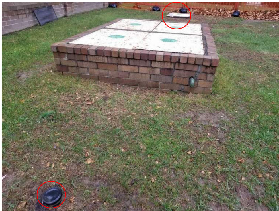
Photograph 35: View of 40,000 gallon No. 6 Fuel Oil underground storage tank (UST) vault and fill port and access hatch on southern adjoining property in courtyard (facing west).
