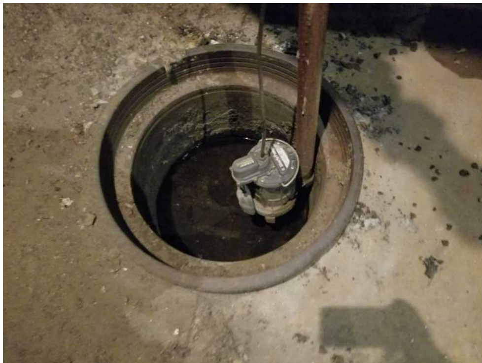
Photograph 9: View of sump in the boiler room of the Leviton cellar (facing east).
