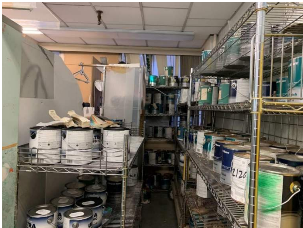
Photograph 18: View of paint storage room in cellar of the Masin building (facing south).
