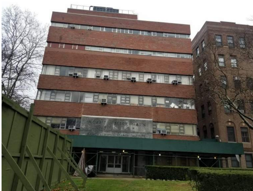
Photograph 2: View of the Masin building from the courtyard (facing east)
