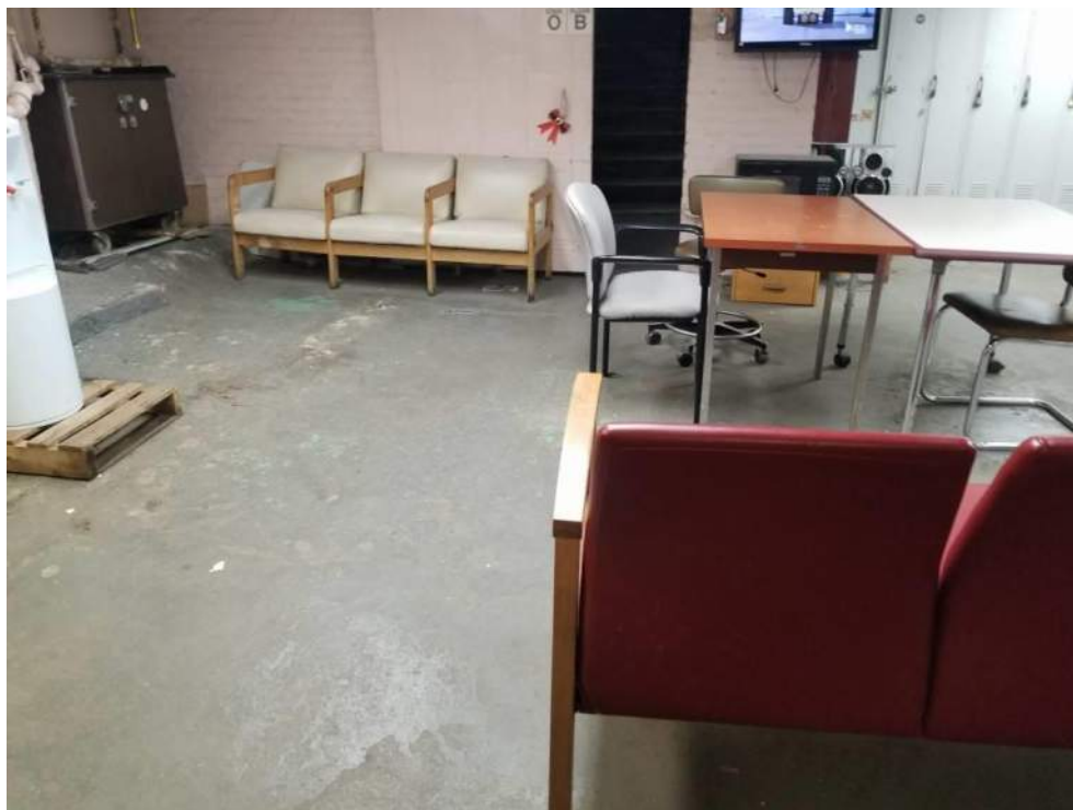
Photograph 28: View of a staff break room in the cellar of the LeFrak building (facing south).
