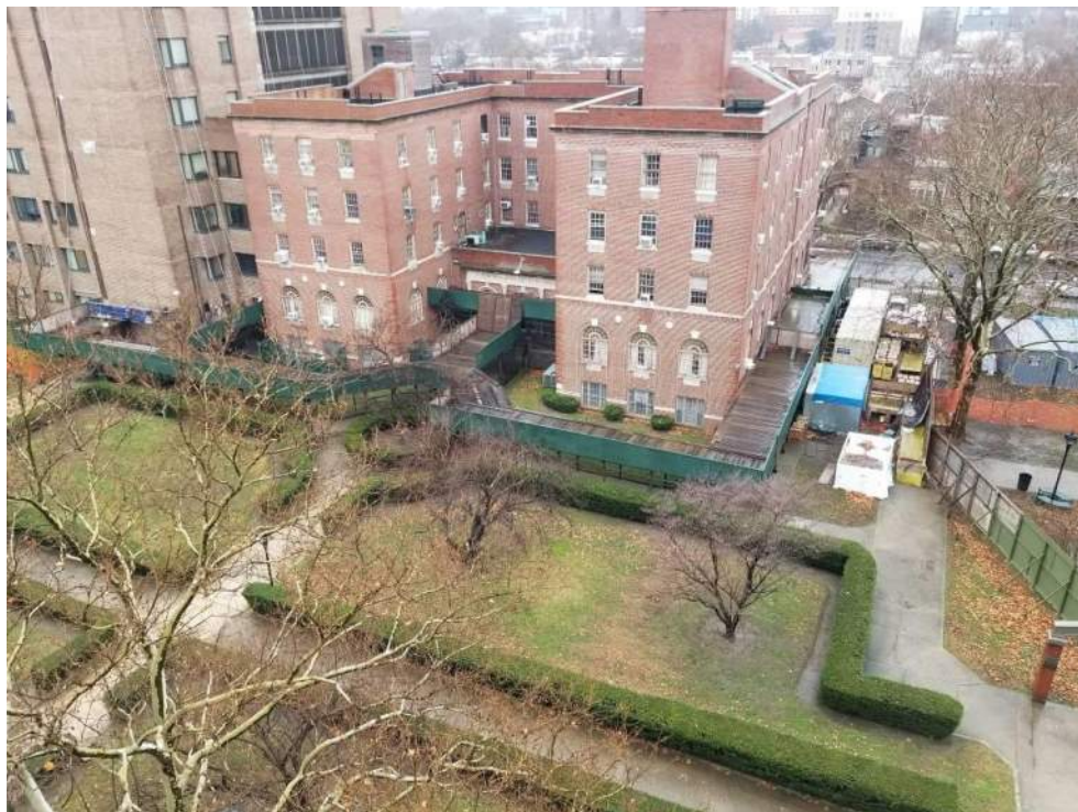
Photograph 1: View of the Leviton building and courtyard from the roof of the Masin building (facing southwest)
