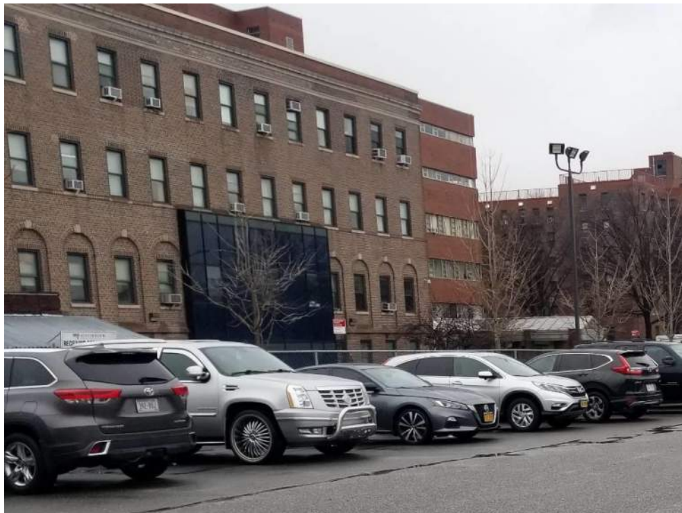
Photograph 4: View of the LeFrak Building from the parking lot across East 49 th Street (facing northwest).
