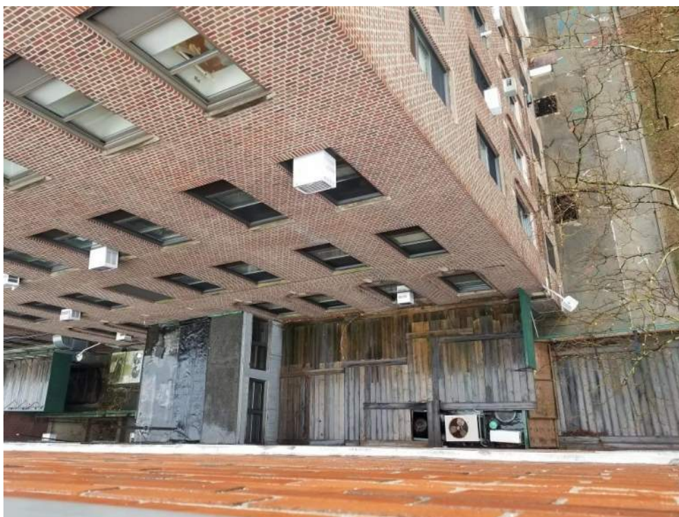
Photograph 32: View of southern Subject Property boundary between the Leviton building and Rutland Nursing Home (facing south).
