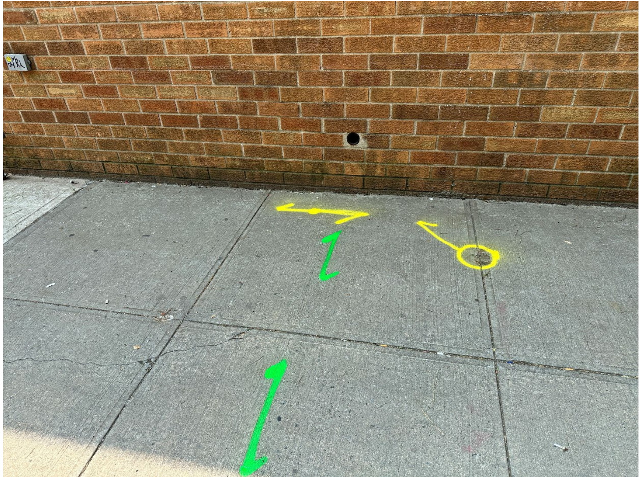
Photo 5 - Sewer line connecting from the street to the side of the building. A vent is visible in the photo which the sewer line was traced out leading directly to.
