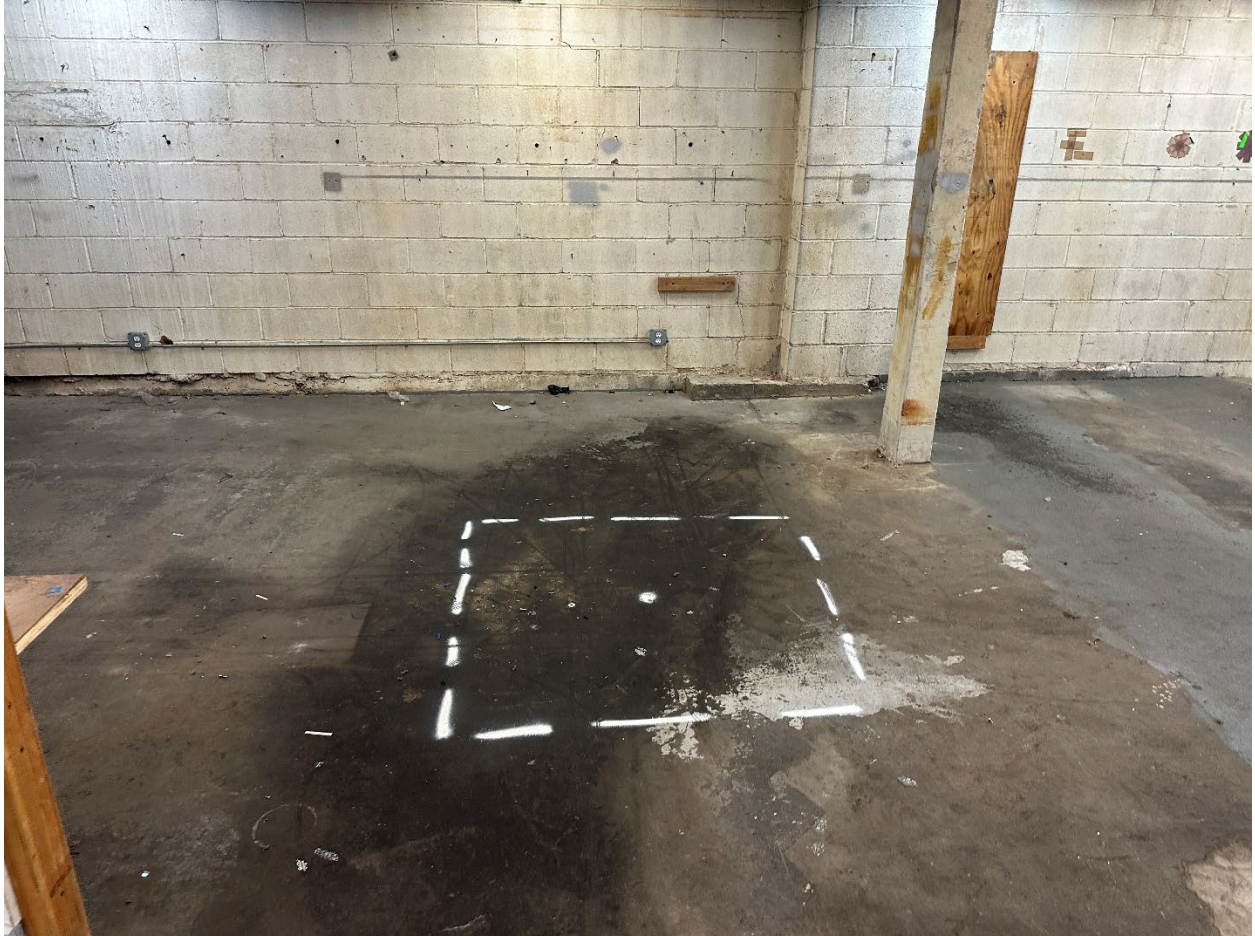
Photo 1 – SB-1 cleared of all utilities and safe for drilling. A 4x4 box was marked to perform drilling and give options.
