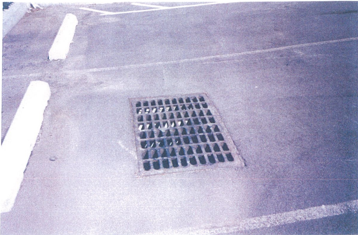
VIEW OF TYPICAL OPEN-GRATE SUBSURFACE DRAINAGE STRUCTURE
