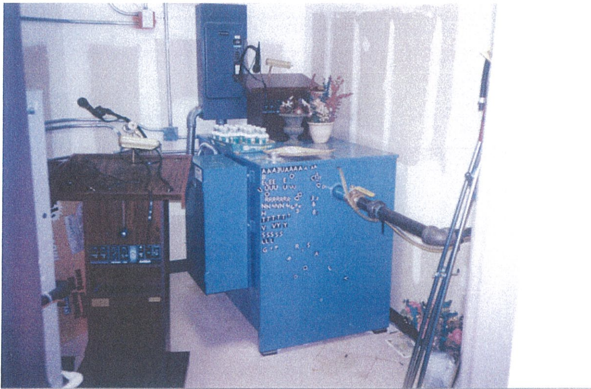
VIEW OF ELEVATOR MOTOR UNIT
