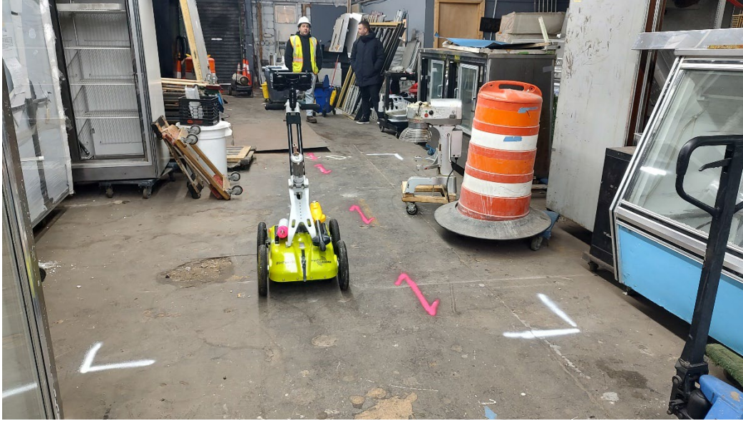
Photo 1 & 2 – View of the area cleared within property #1035 for the collocated locations. the pink marking indicated the detected drainage line leading to the covered cleanout pit seen here.
