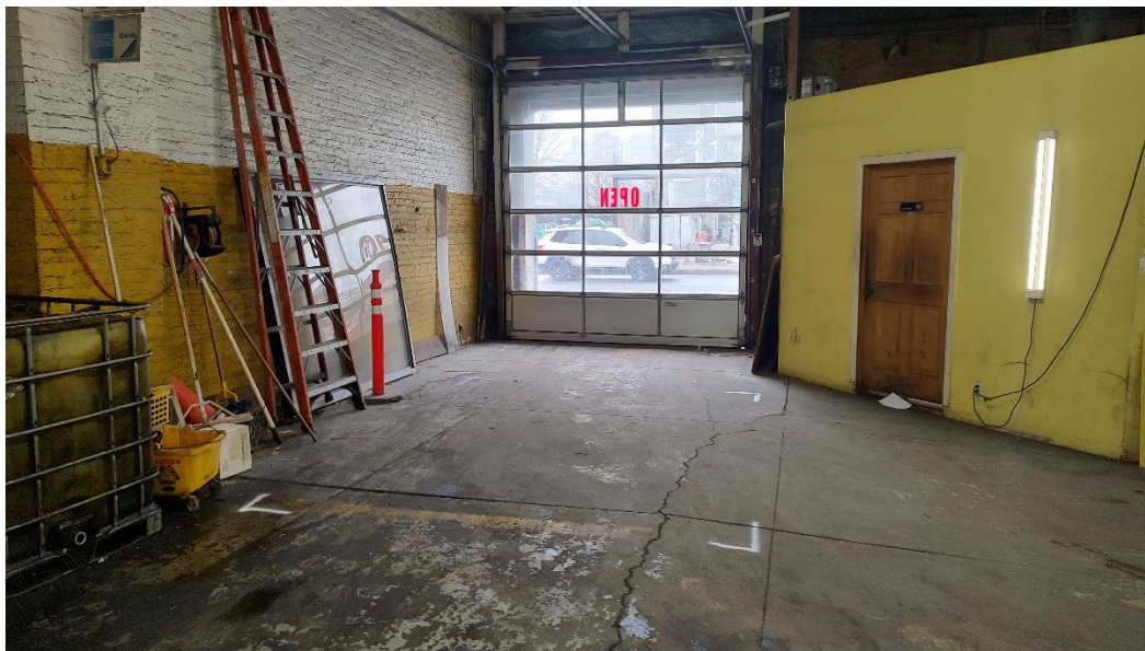
Photo 3 – One of the locations cleared inside the mechanic's shop, showing no detections.
