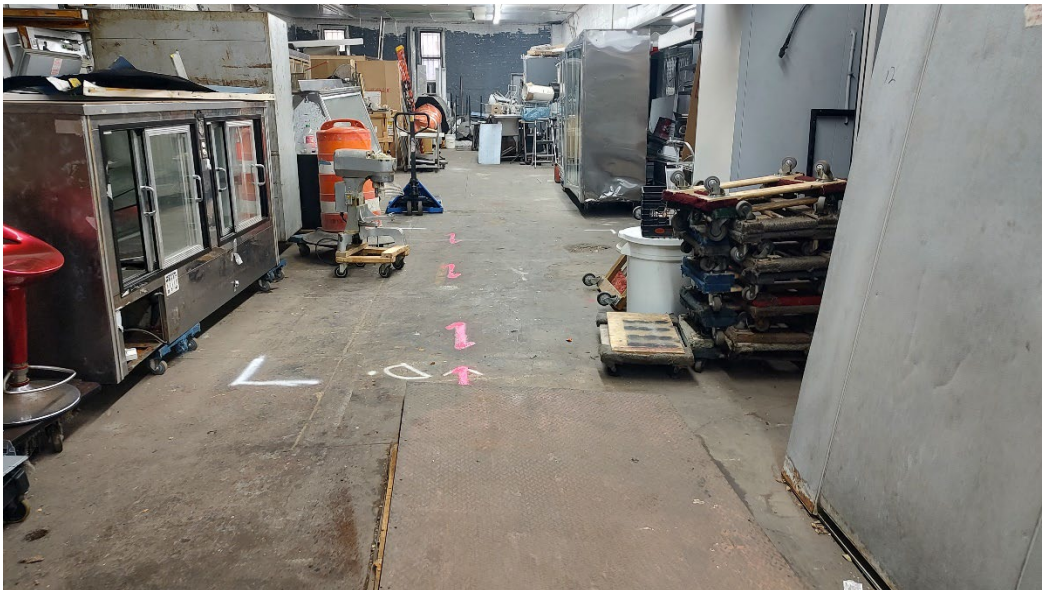
Photo 1 & 2 – View of the area cleared within property #1035 for the collocated locations. the pink marking indicated the detected drainage line leading to the covered cleanout pit seen here.
