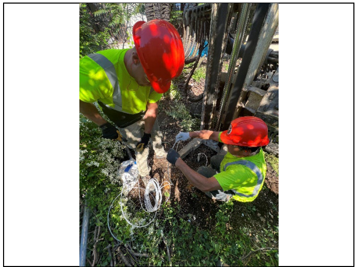
6. Soil Vapor Probe Installation (September 2024)
