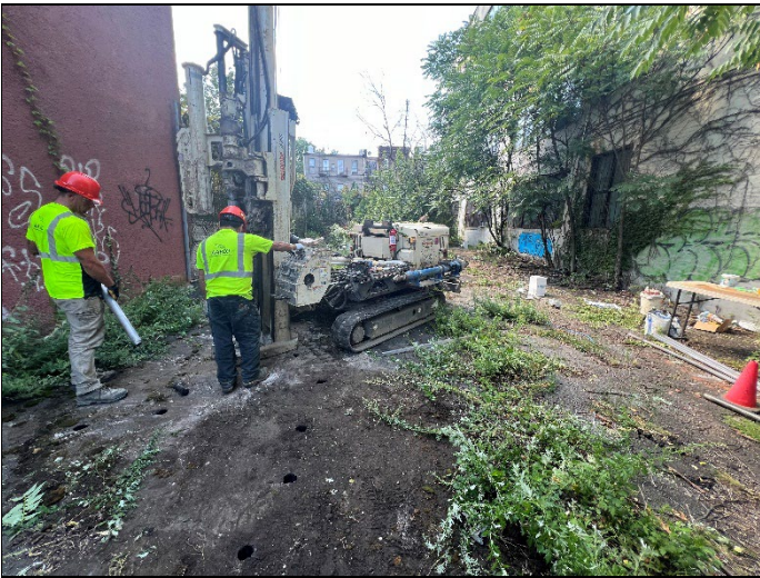
3. Soil Probe Installation (September 2024)
