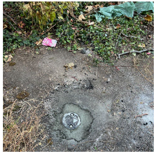
22. Groundwater Monitoring Well
