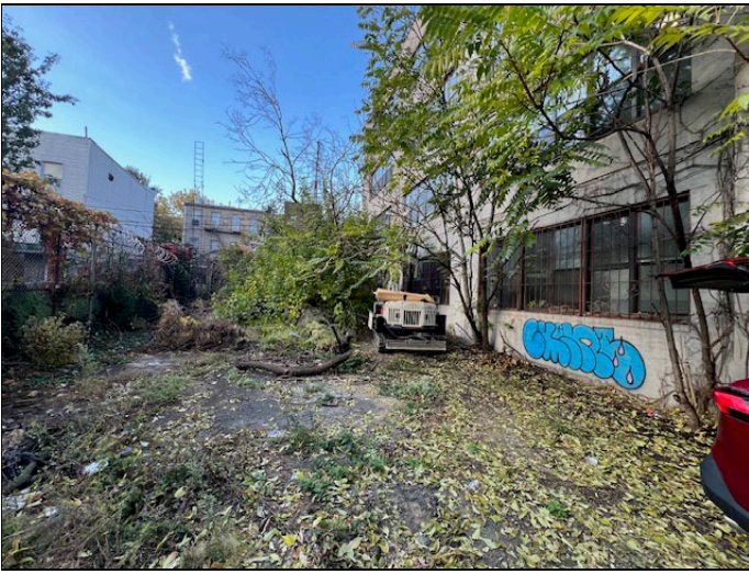
13. Soil Probe Installation (October 2024)
