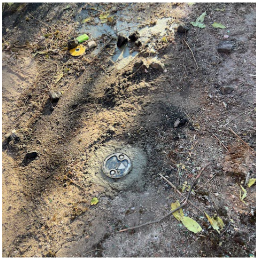
21. Groundwater Monitoring Well
