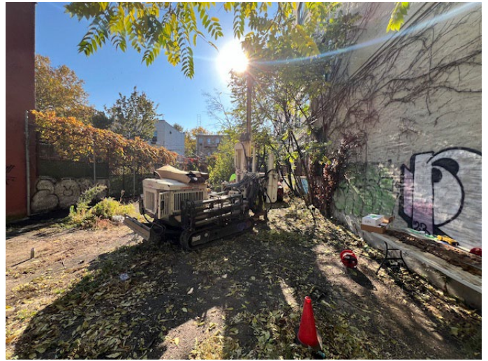
20. Soil Probe Installation (October 2024)
