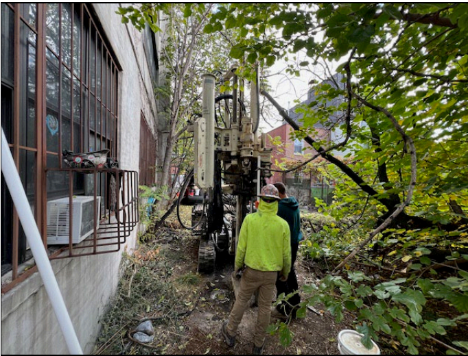
15. Soil Probe Installation (October 2024)
