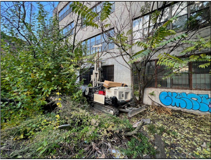
14. Soil Probe Installation (October 2024)
