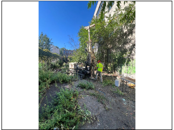
4. Soil Probe Installation (September 2024)
