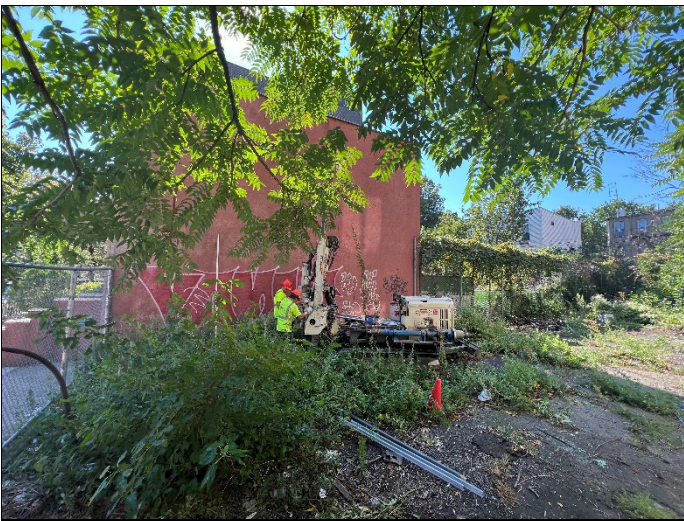
5. Soil Probe Installation (September 2024)
