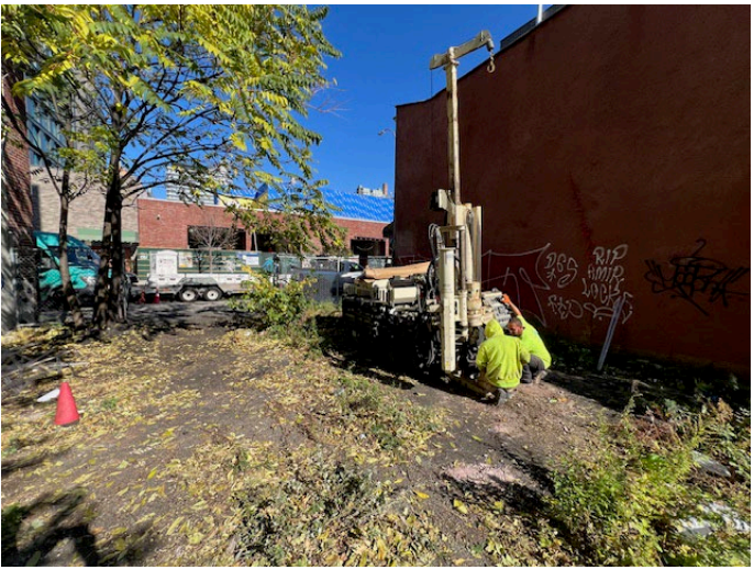
18. Soil Probe Installation (October 2024)
