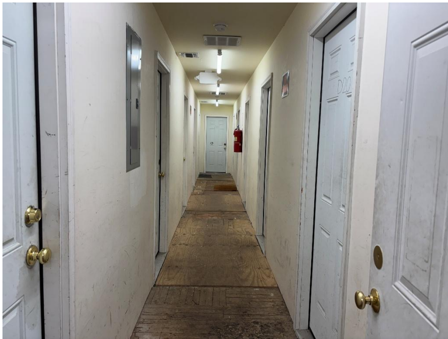
Photo 10: View of internal hallway on Lot 45 of the site, facing east.
