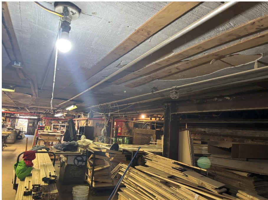
Photo 4: View of the cellar on Lot 48 of the site, facing south.
