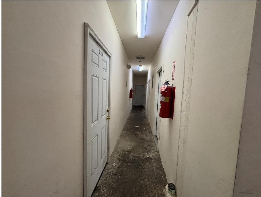
Photo 9: View of internal hallway on Lot 45 of the site, facing east.
