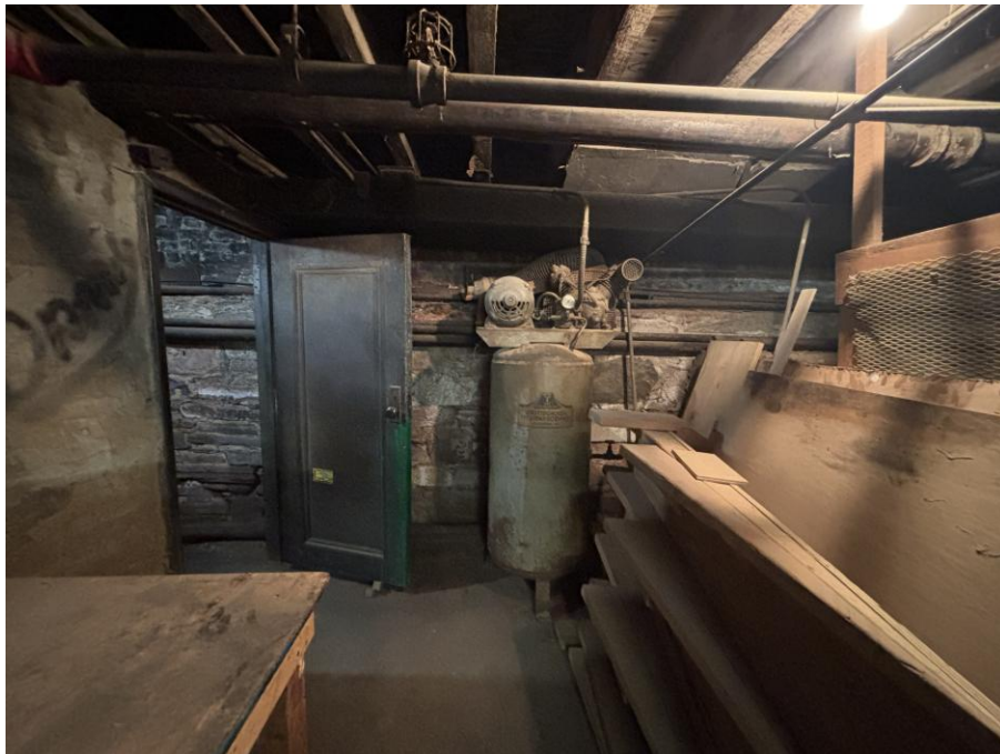
Photo 6: View of the cellar on Lot 48 of the site, facing west.
