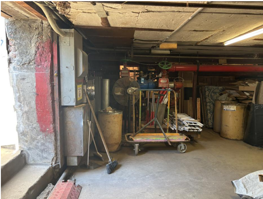
Photo 8: View of the cellar on Lot 48 of the site, facing east.
