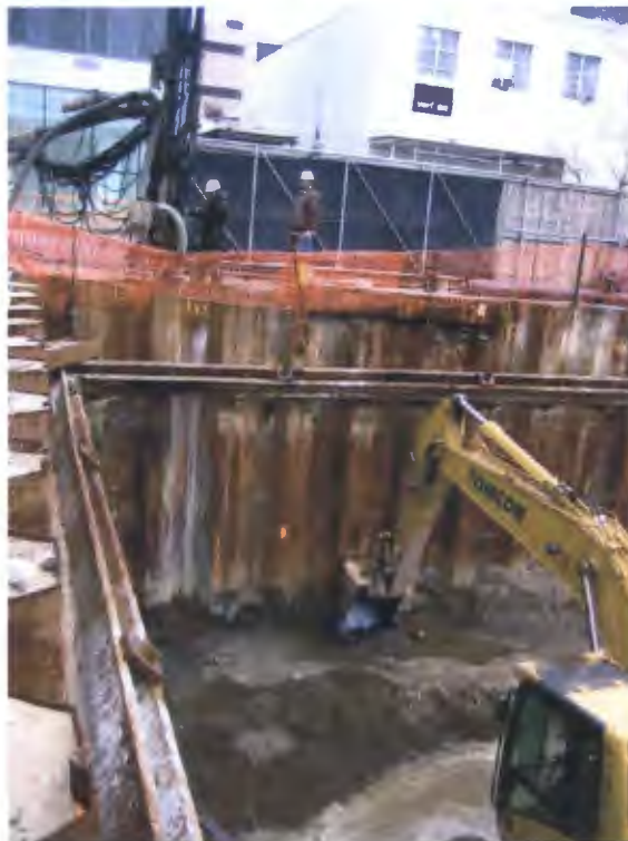
Figure 2. Contractor is drilling additional borings above the seepage area on January 12.
