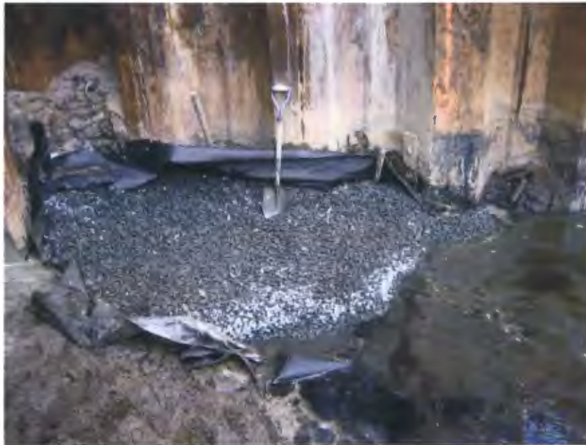
Figure 4. Excavating the cover soil that was contaminated by the groundwater seepage on Jan. 16
