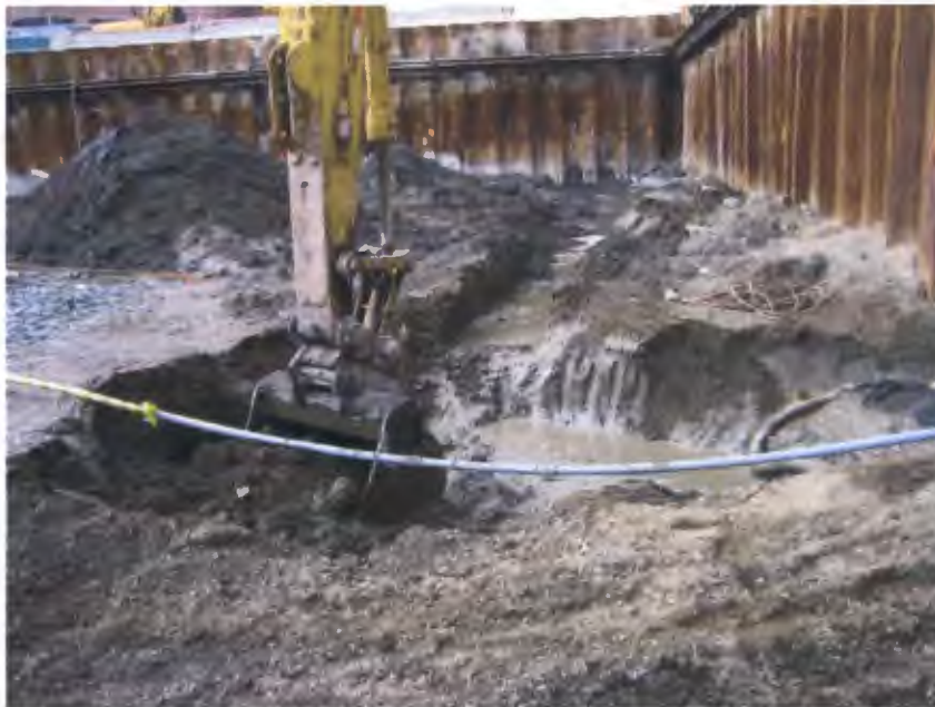
Figure 4. Excavating the cover soil that was contaminated by the groundwater seepage on Jan. 16
