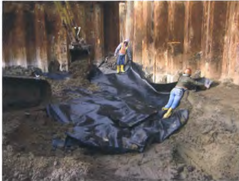
Figure 5. Contractor is backfilling the excavation on January 16. In the northwest corner itself, the original geotextile fabric was destroyed by the repair activities
