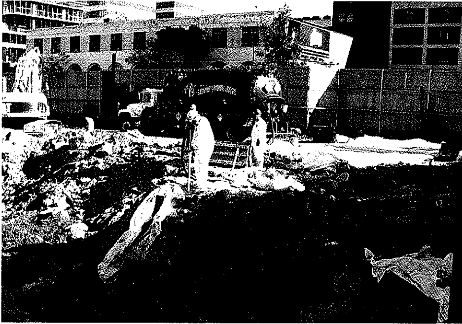
Photo 1: Vacuuming contents of Tank 5
