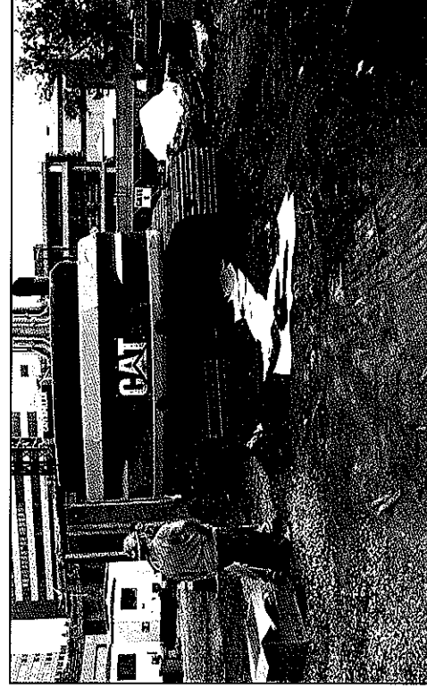
Figure 2 – Hydraulic spill from excavator contained with absorbent pads.
