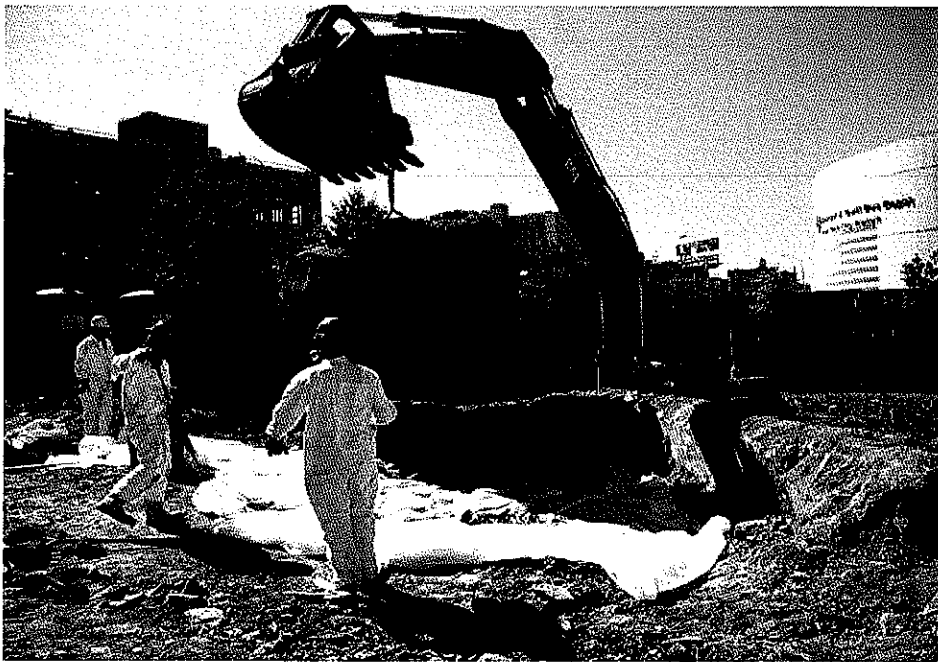
Photo 8: Removal of Tank 5
