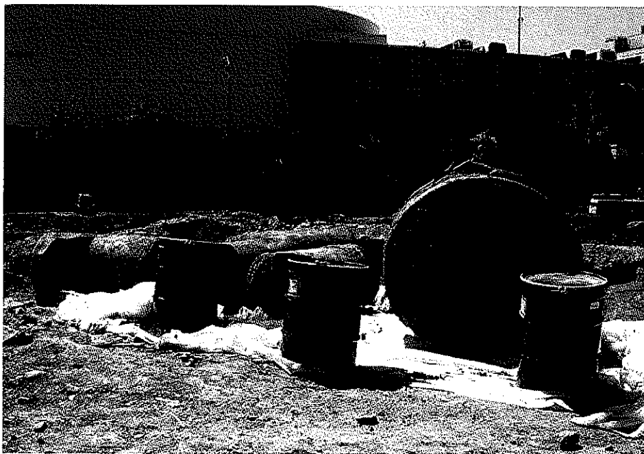
Photo 12: Tanks and drummed waste following removal activities
