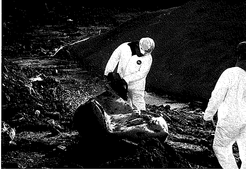
Photo 3: Another shot of UST being cut open.
