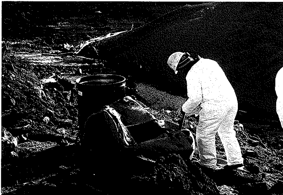
Photo 2: Cutting open UST to clean and inert.
