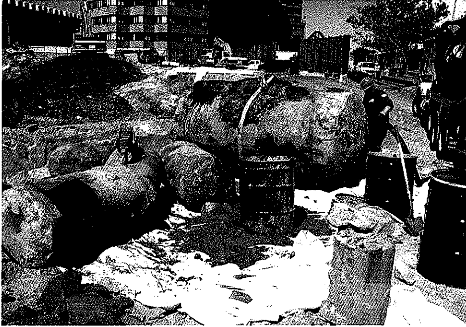
Photo 9: All five tanks and, around drum, soil impacted by spill during Tank 5 removal
