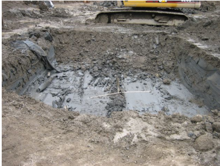
Figure 1. Overview of excavation. The wood stake indicates the approximate location of where the refusal was encountered.
