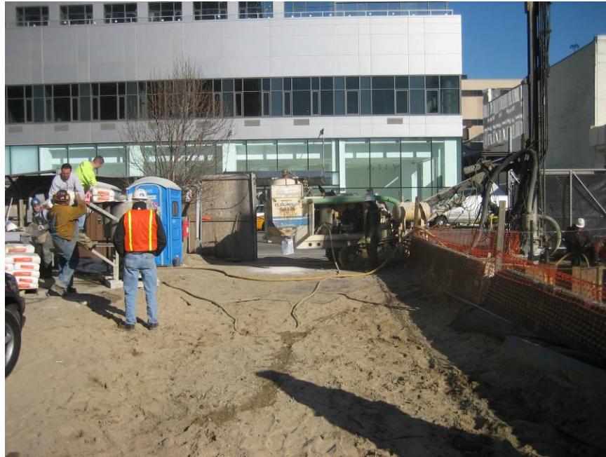
Figure 1. Contractor is mixing grout (left side of photo) with the drill rig standing by to redrill the boring if necessary on January 3 rd , 2007.
