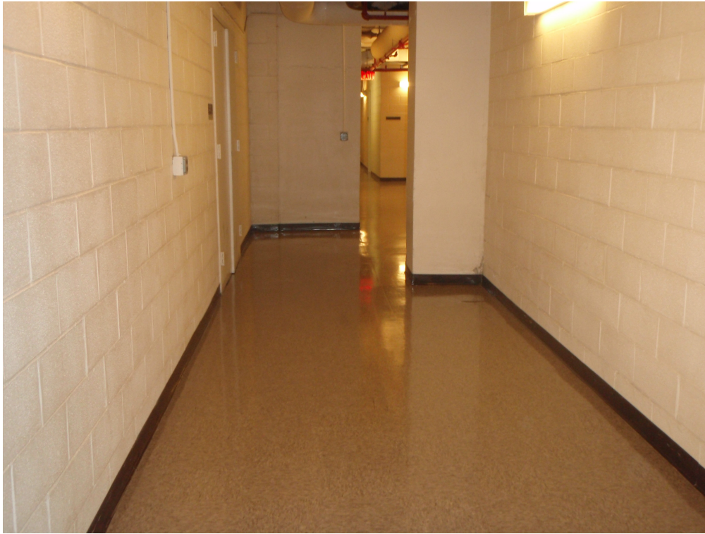
Photograph No. 9: View of hallway floor in lowest level of River Place II.
