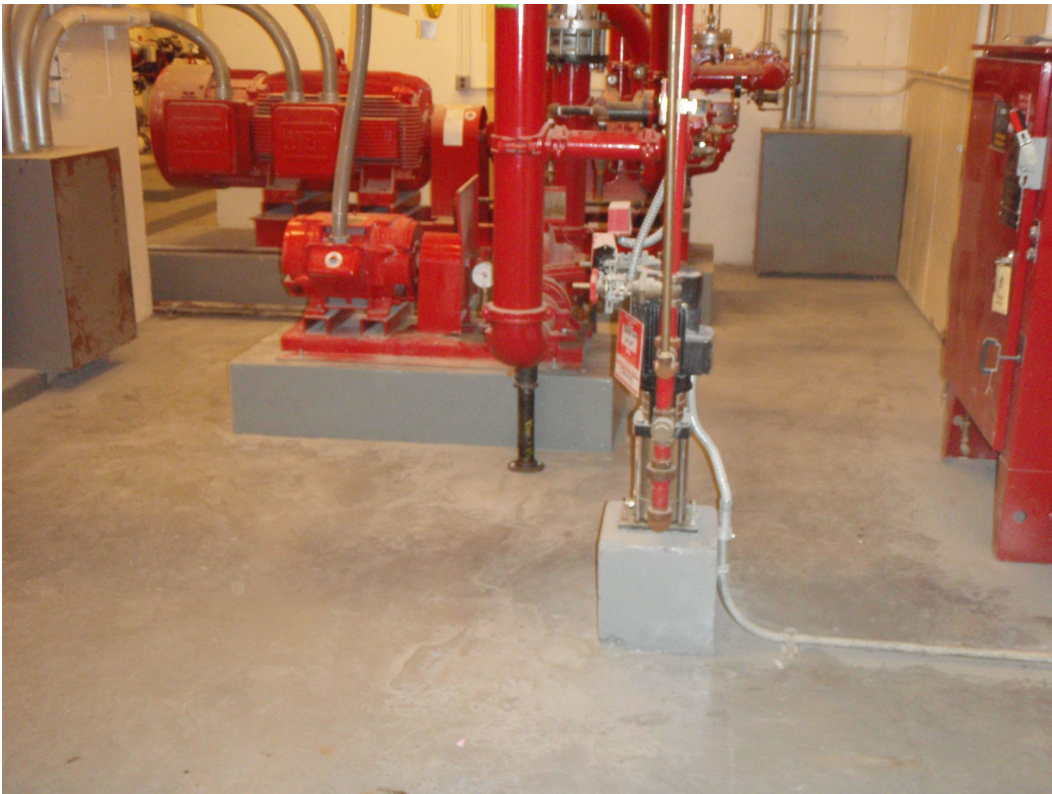
Photograph No. 8: View of cellar floor in lowest level of River Place II
