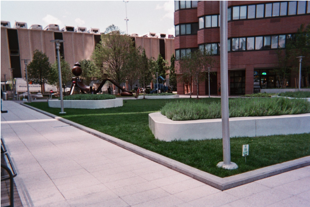
Photograph No. 1: View of paved walkway area located between River Place II building and W. 42 nd Street.
