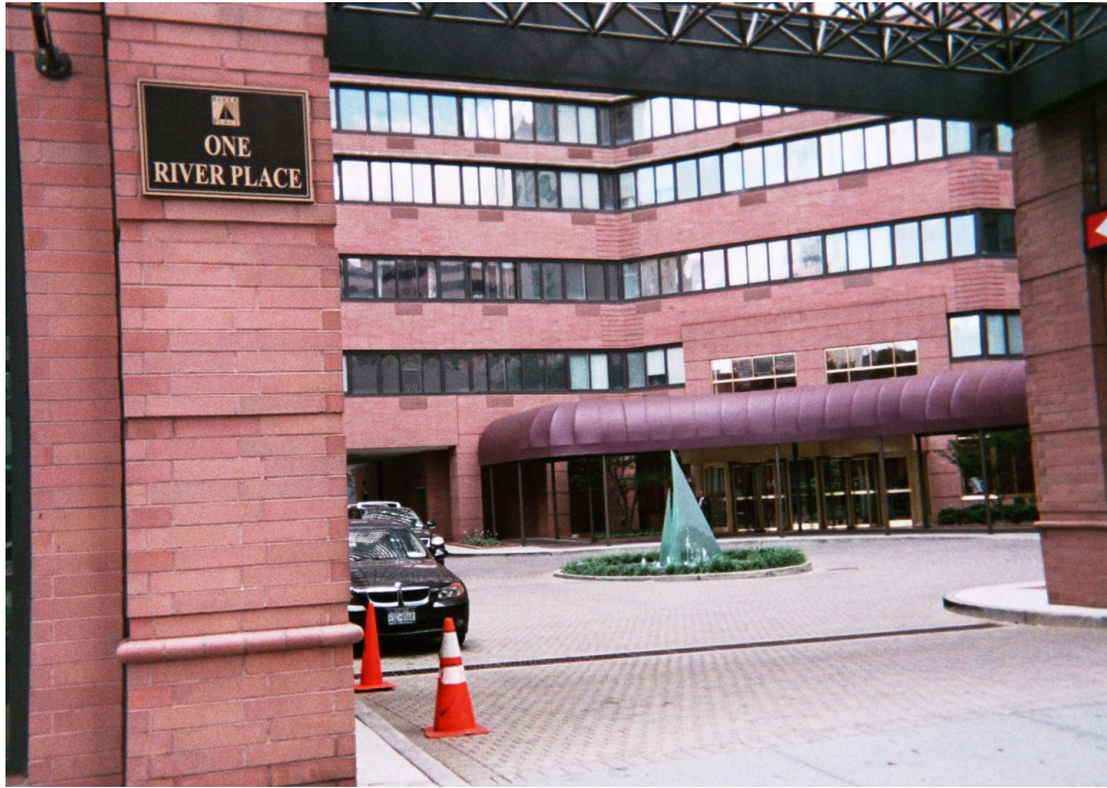
Photograph No. 3: View of capped driveway area for River Place I.
