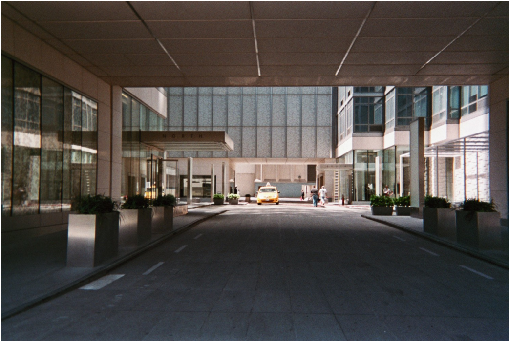
Photograph No. 7: View of capped driveway area for River Place II.
