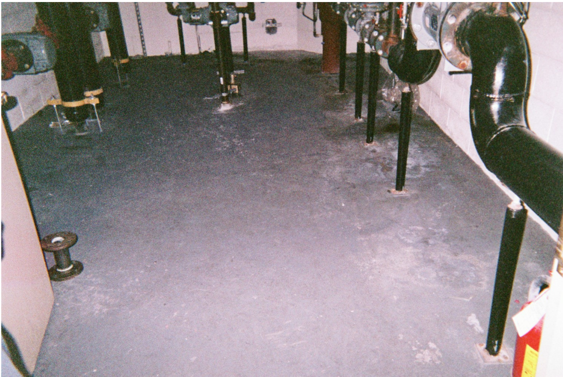
Photograph No. 6: View of concrete floor in lowest level of River Place I.
