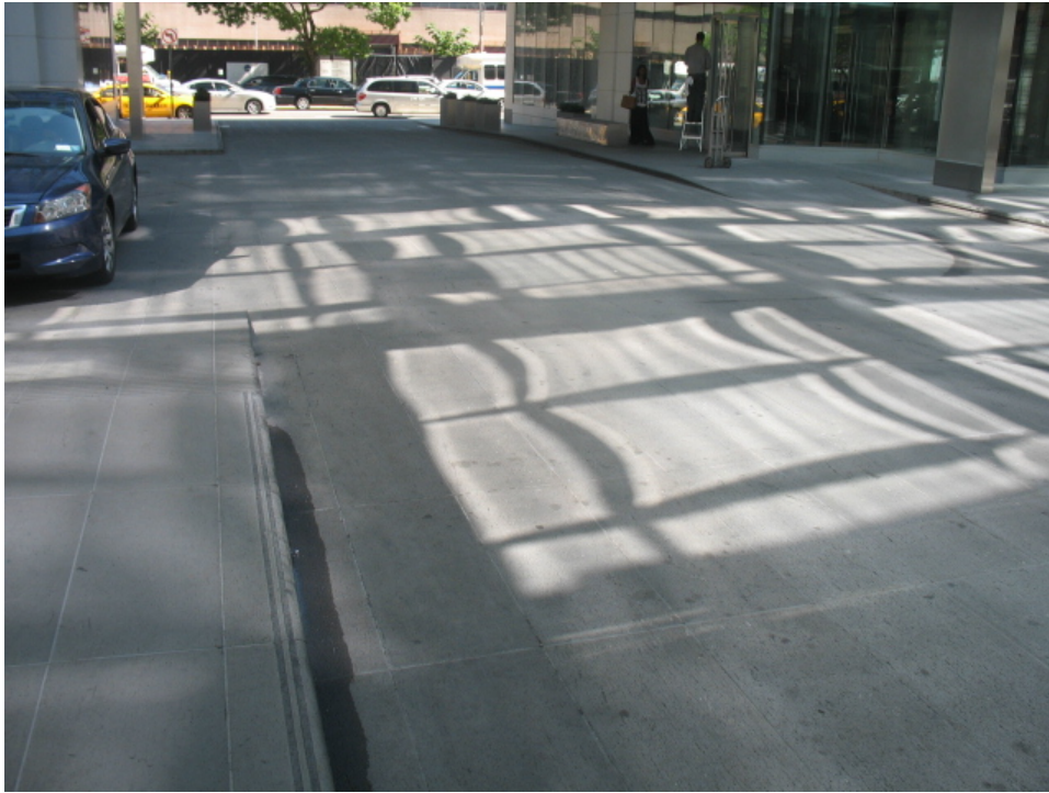
Photograph No. 1: View of paved walkway/driveway area located between River Place II buildings (North and South Towers).
