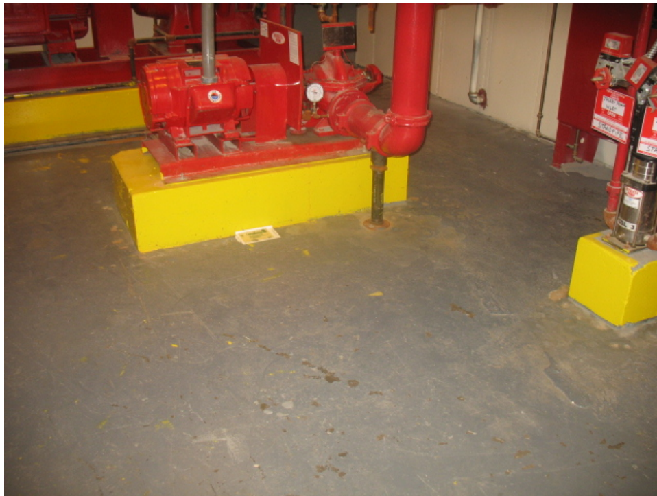
Photograph No. 6: View of cellar floor in the pump room of River Place II.
