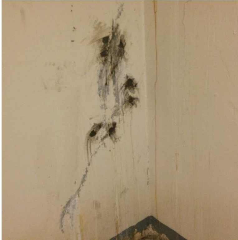
Photograph 7: View of sealed crack in sub cellar (12/2/15).
