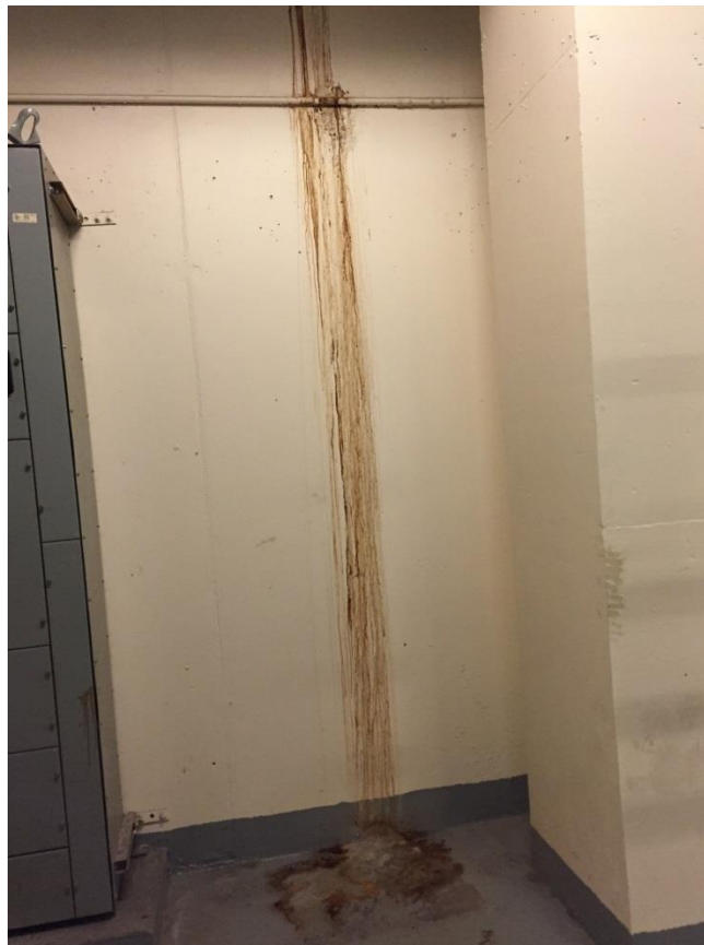
Photograph 4: View of leaks in sub cellar (8/6/15).
