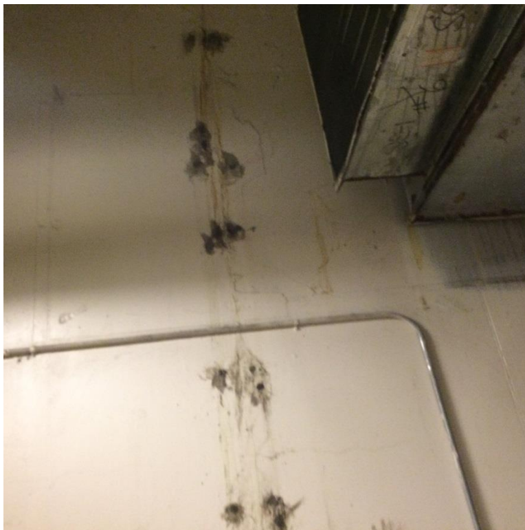
Photograph 10: View of sealed crack in sub cellar.
