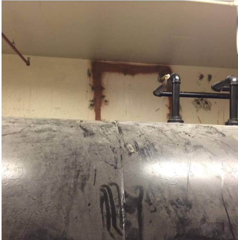
Photograph 5: View of sealed cracks in oil tank room, marked with bronze paint (12/2/15).
