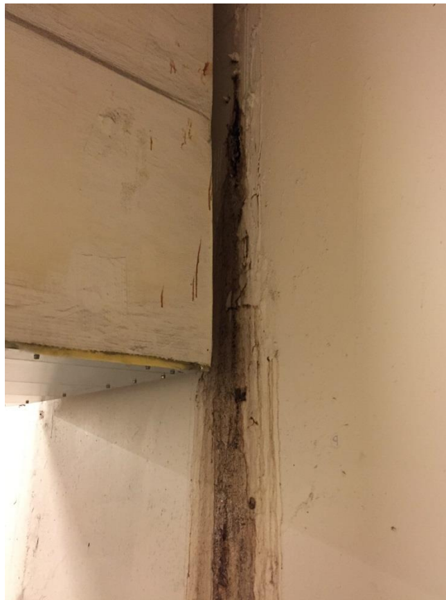
Photograph 2: View of leaks in sub cellar (8/6/15).
