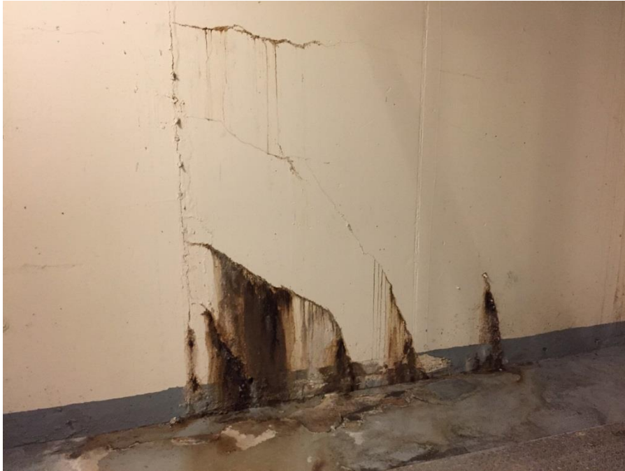
Photograph 3: View of leaks in sub cellar (8/6/15).
