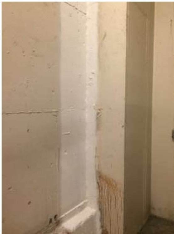
Photo 4: Repaired wall of the sub-cellar level on August 31, 2016.
