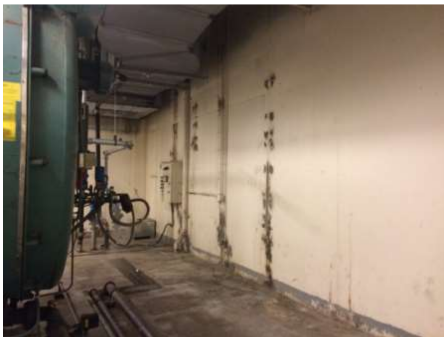
Photo 10: Surface cover and wall grout injections in Site boiler room.
