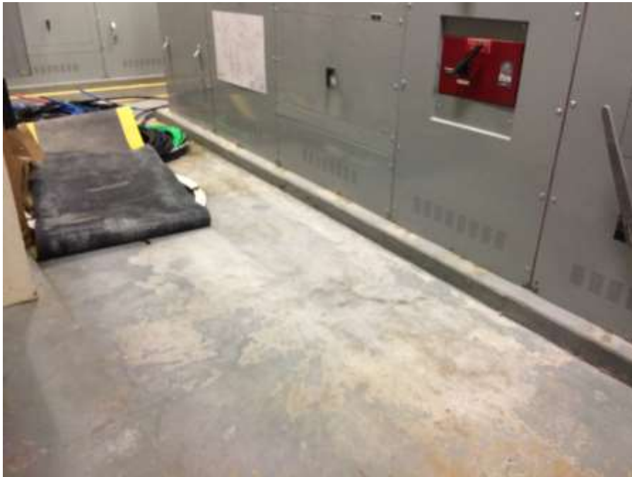
Photo 13: Surface cover in Site mechanical room.
