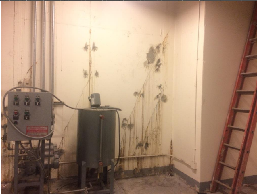
Photo 3: Grout injections on the wall of the sub-cellar level.
