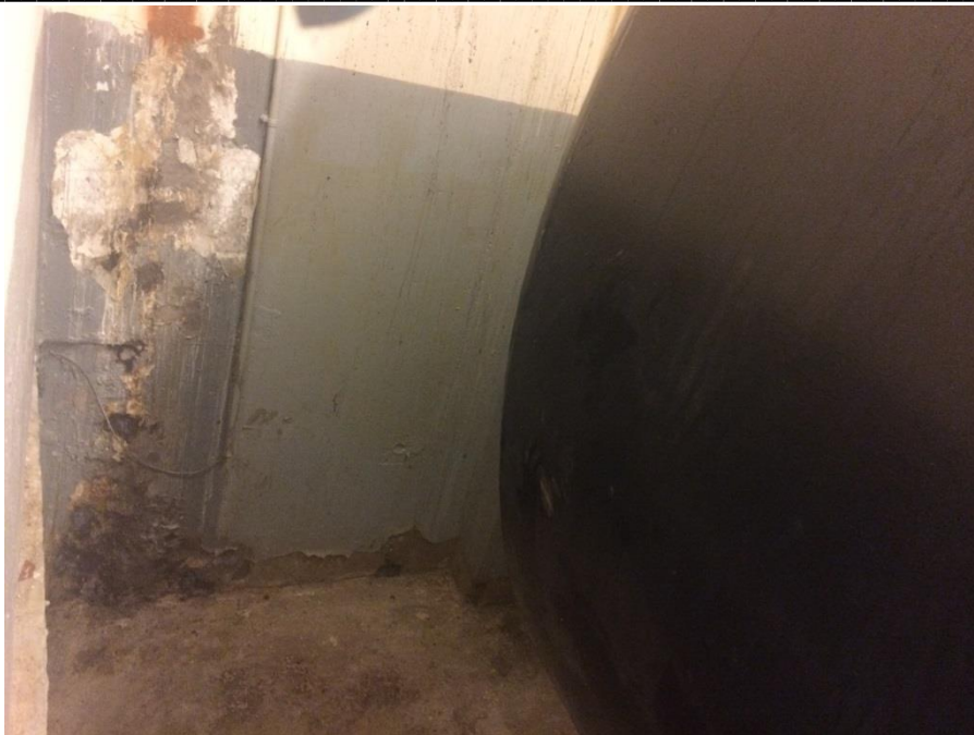
Photo 7: Grout injections and surface cover in Site AST room.
