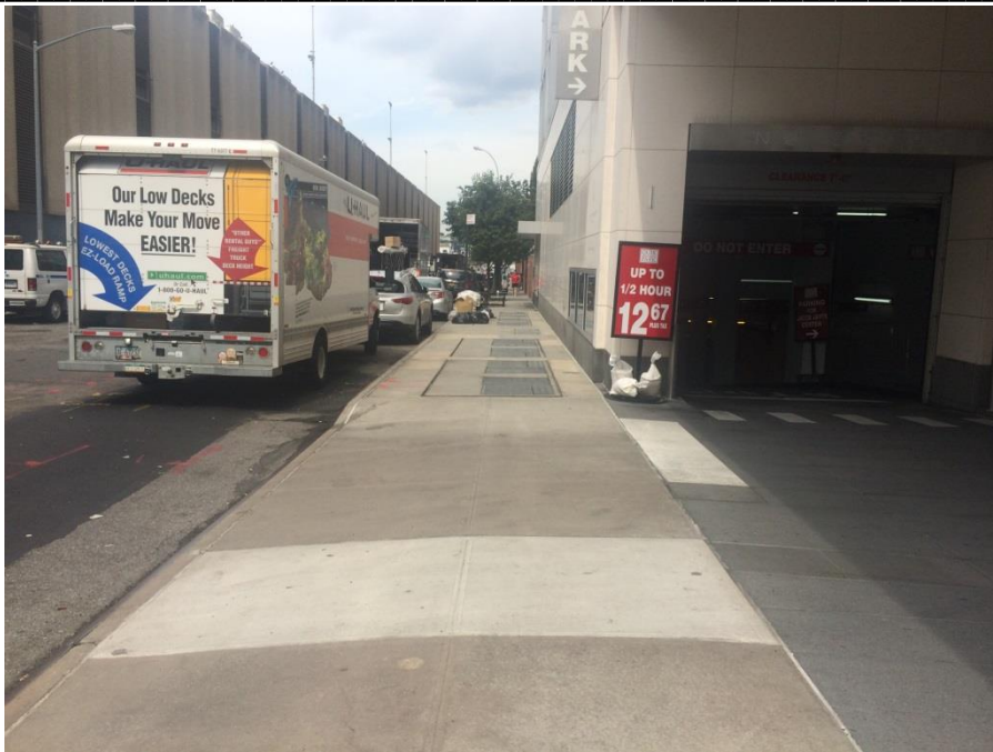
Photo 15: West 41 st Street sidewalk – facing west.
