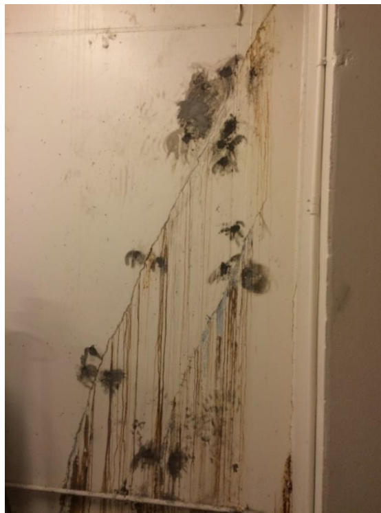
Photo 2: Grout injection locations on the wall of the sub-cellar level.
