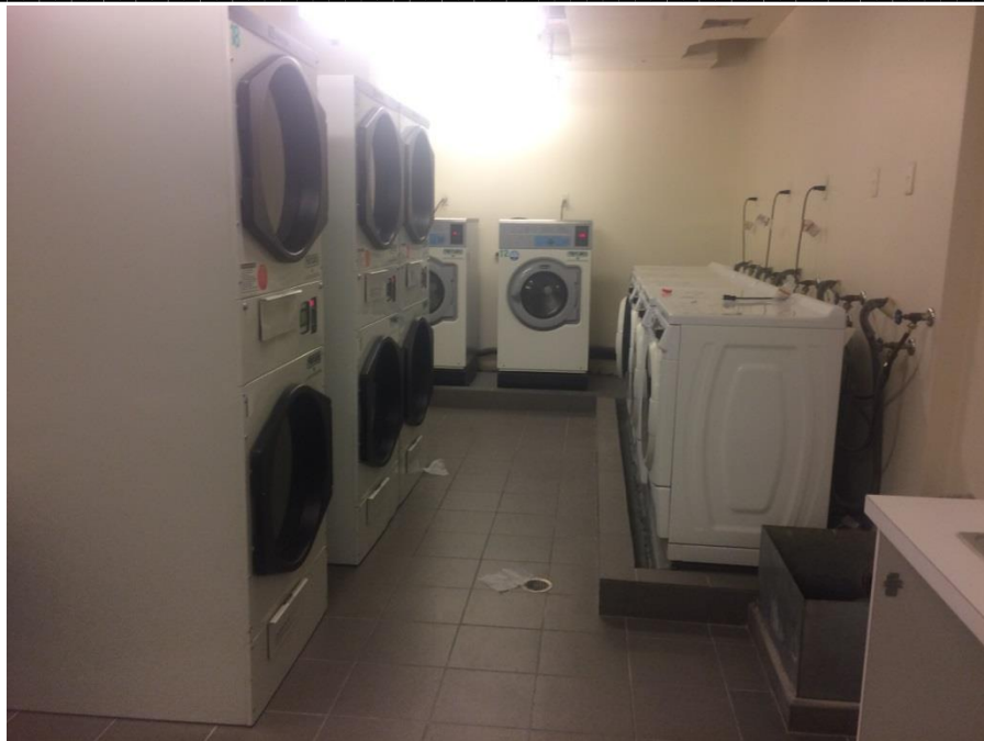
Photo 9: Surface cover in Site laundry room.
