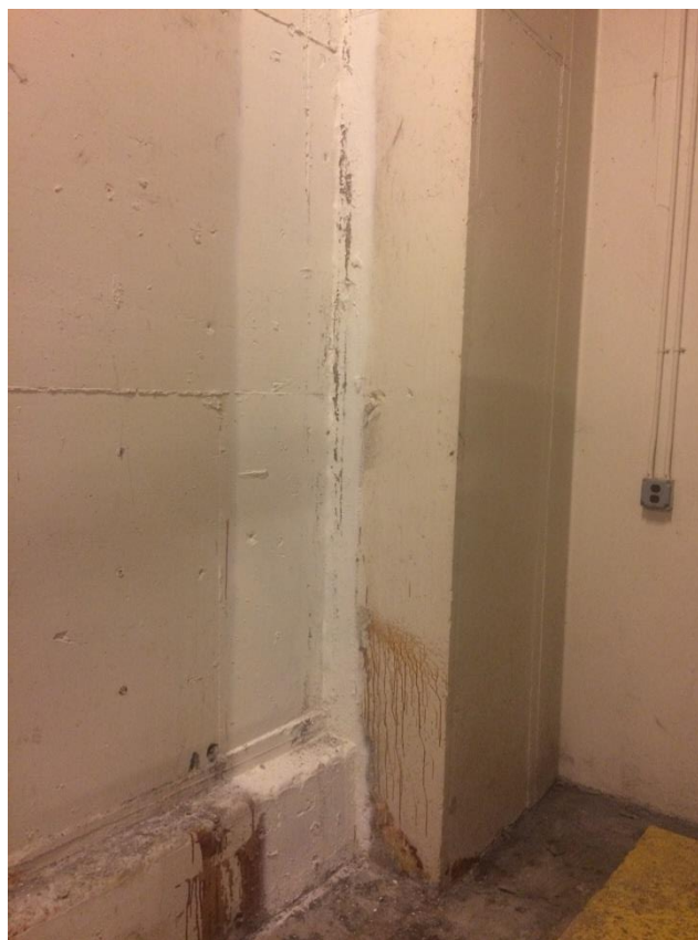
Photo 4: Previously repaired wall of the sub-cellar level.
