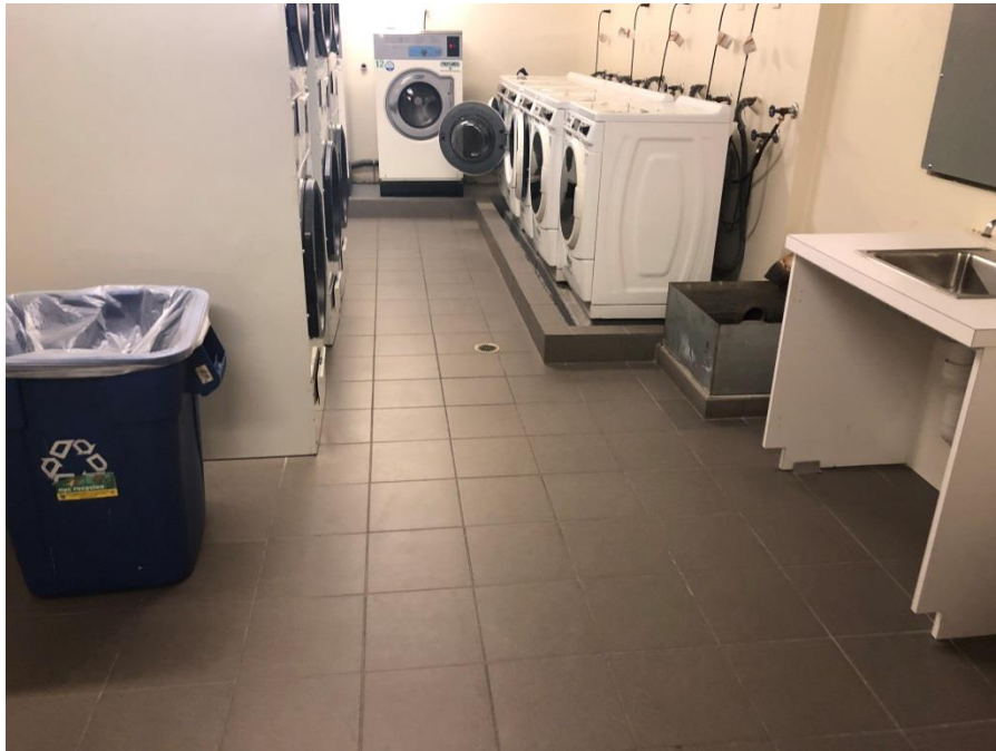
Photo 11: Surface cover in Site laundry room.
