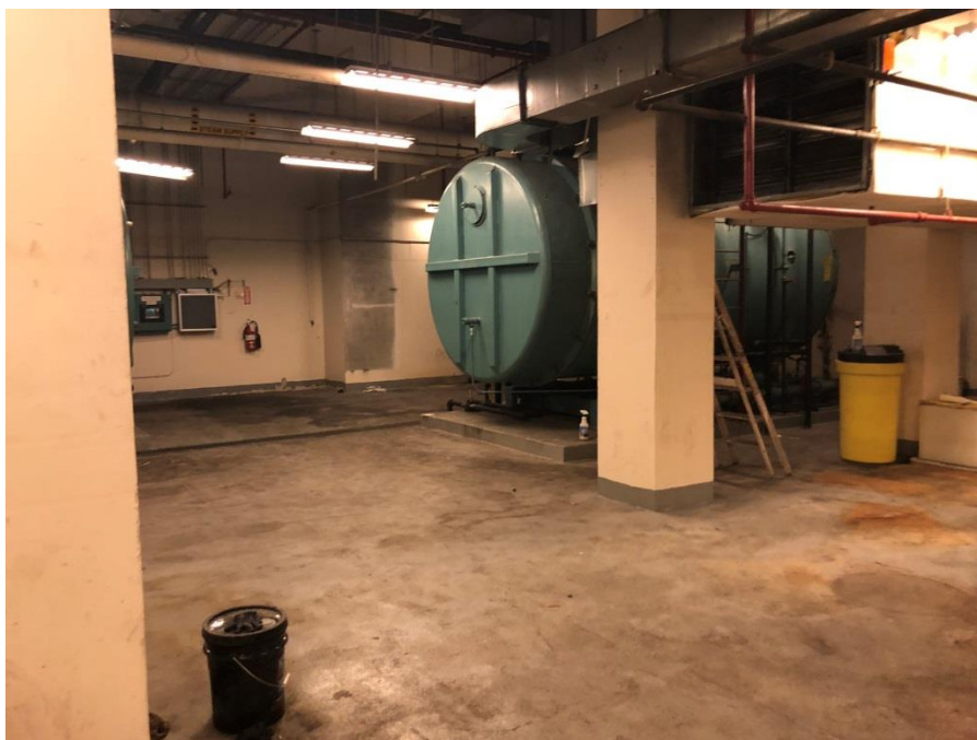
Photo 4: Surface cover in the Site boiler room.
