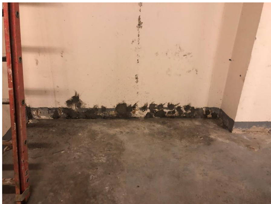
Photo 6: Previously repaired wall of the Site sub-cellar level boiler room.
