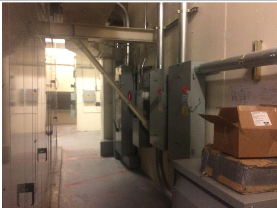
Photo 15: Surface cover in Site mechanical room.
