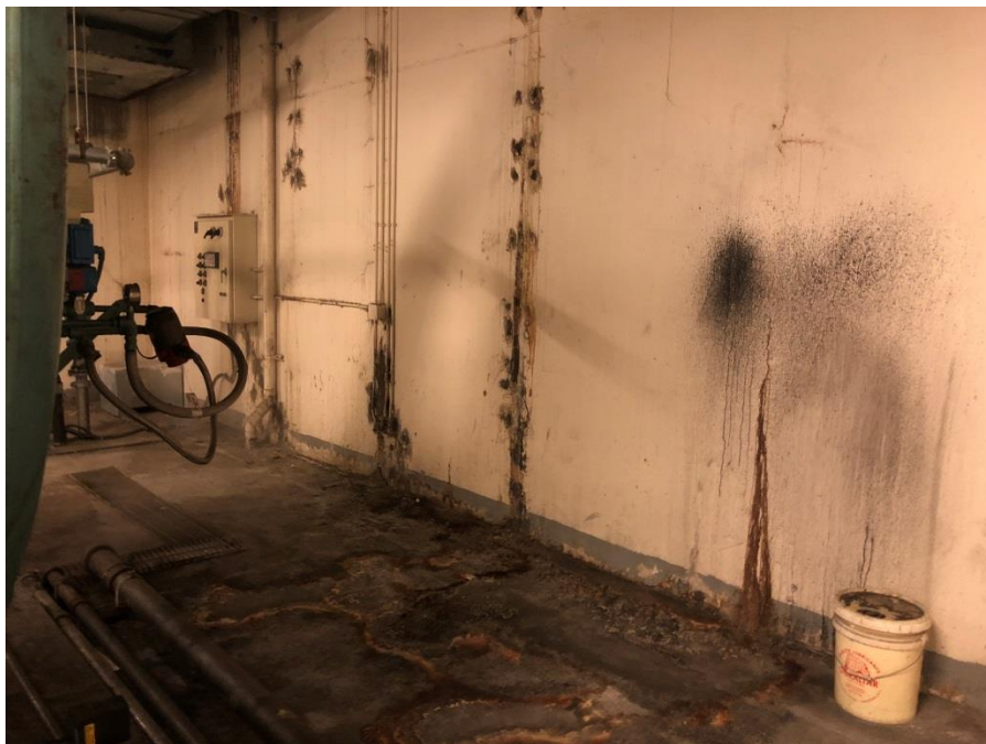
Photo 12: Surface cover and wall grout injections in Site boiler room.
