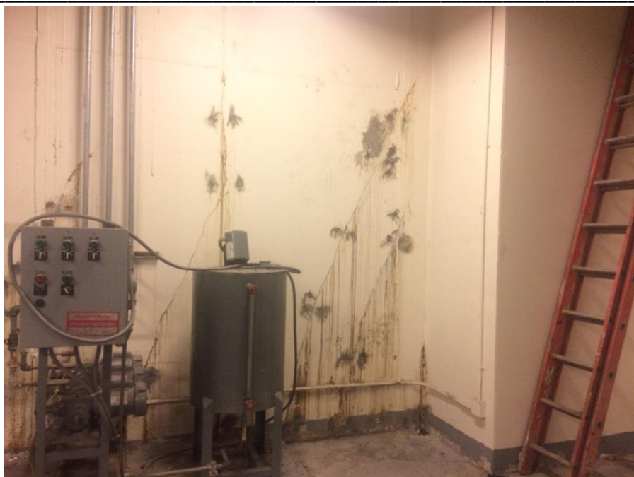
Photo 5: Grout injections on the wall of the sub-cellar level.
