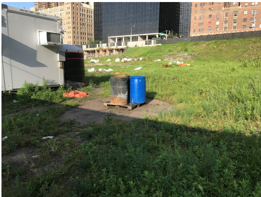
Photograph 3 – View of three 55-gallon drums on a wooden pallet containing diesel fuel for construction trailer generators in the southeast part of the site; no evidence of a spill or staining was observed; facing northeast.
