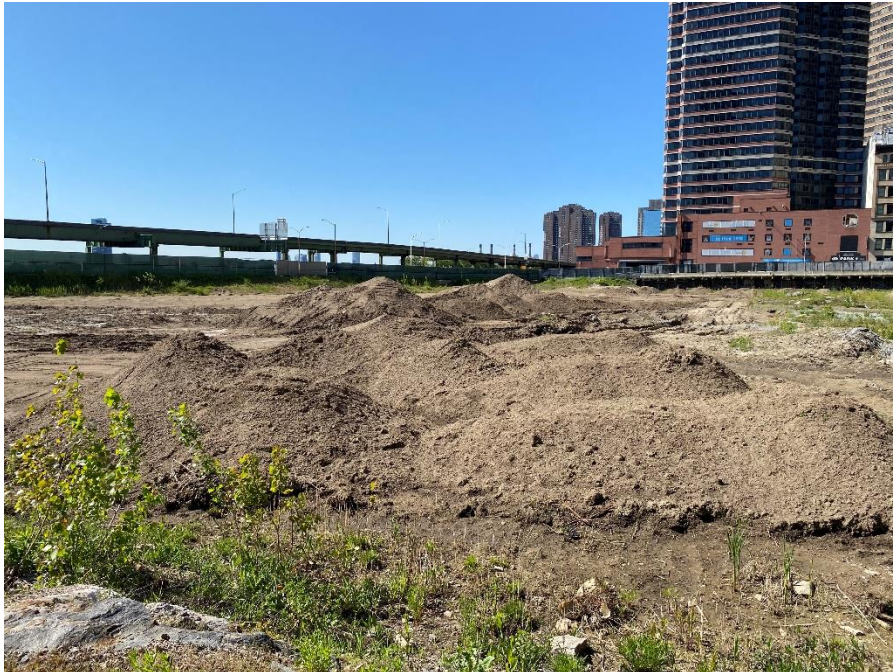
Photograph 6 – View of top soil stockpiled in the central part of the site; facing southeast (photograph dated 5/13/2020).
