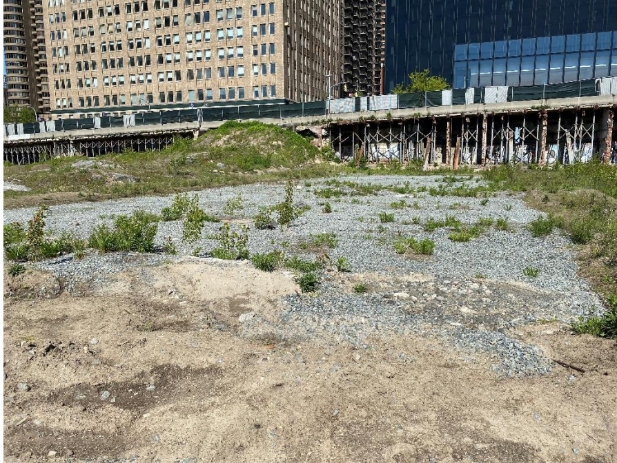
Photograph 7 – View of gravel area in the central west part of the site; facing west (photograph dated 5/13/2020).
