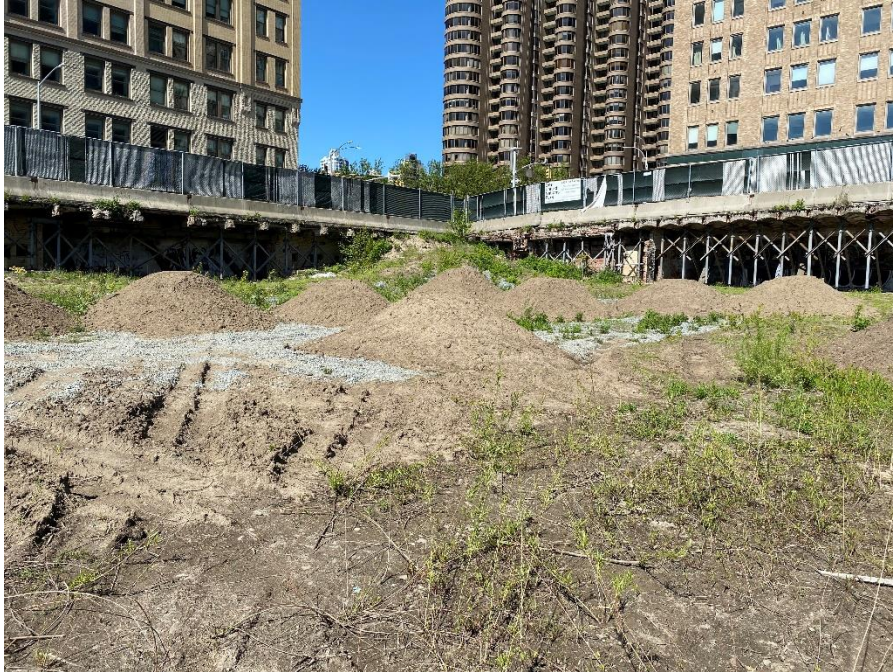
Photograph 9 – View of top soil stockpiled in the southwest corner of the site; facing southwest (photograph dated 5/13/2020).
