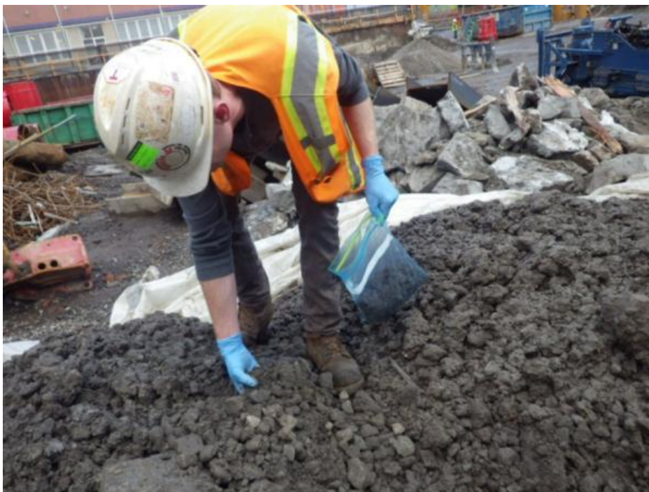
Photograph 11 – View of soil sampling from an impacted stockpile. 11/18/2013
