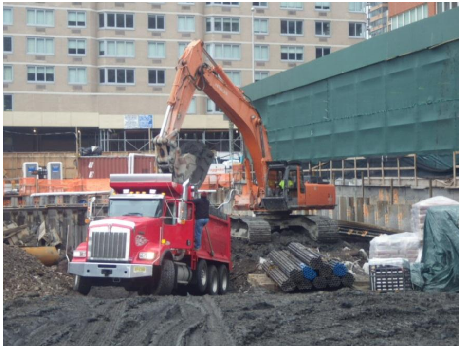
Photograph 18 – View of soil excavation and direct loading into tri-axel dump trucks. 4/4/2014
