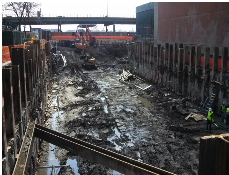
Photograph 20 – Facing east. View of excavated area to approximately 12 feet below grade surface. 4/26/2014
