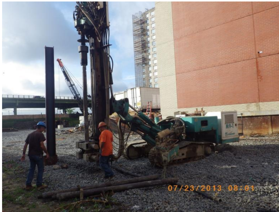
Photograph 3 – Facing east. View of predrilling at a caisson location with an auger rig. 7/23/2013
