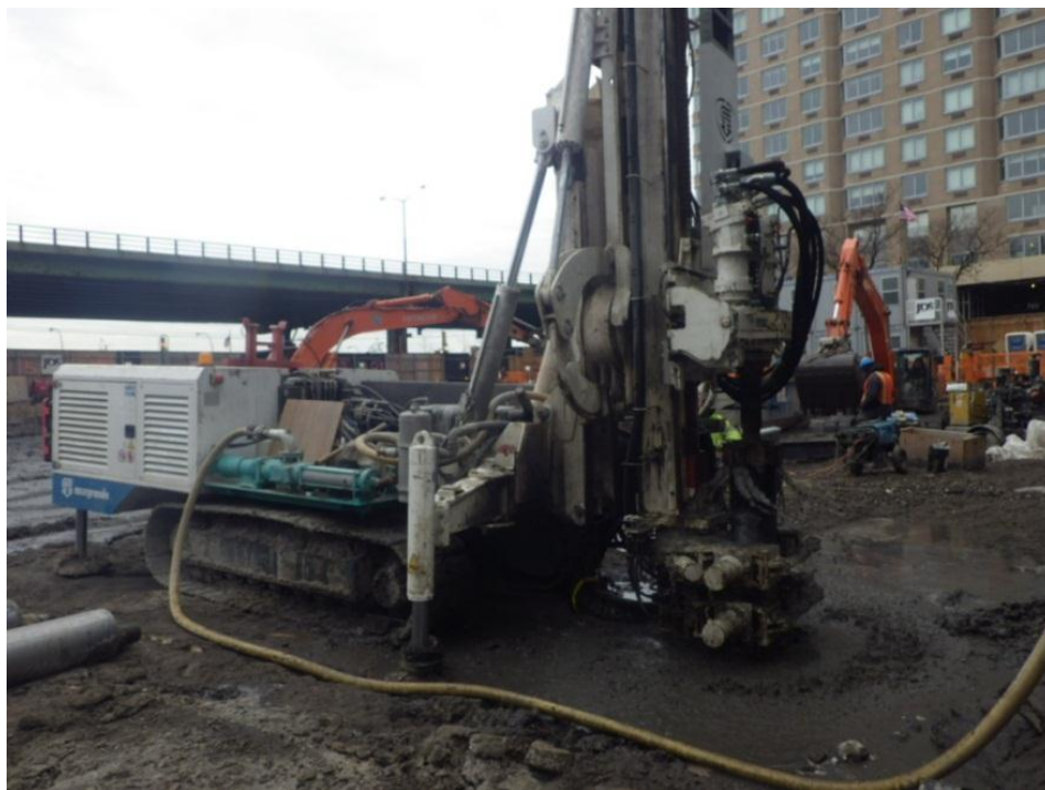
Photograph 16 – View of dewatering well installation. 3/14/2014
