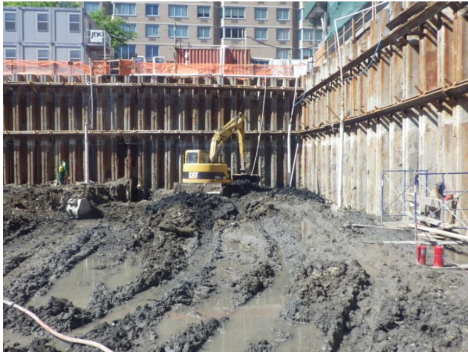
Photograph 25 – View of soil excavation at depths of approximately 22 feet below grade surface. 5/31/2014
