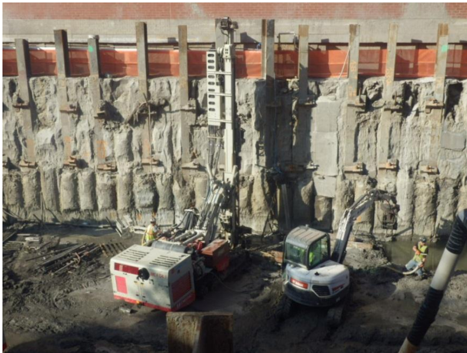
Photograph 24 – View of dewatering well installation. 5/30/2014
