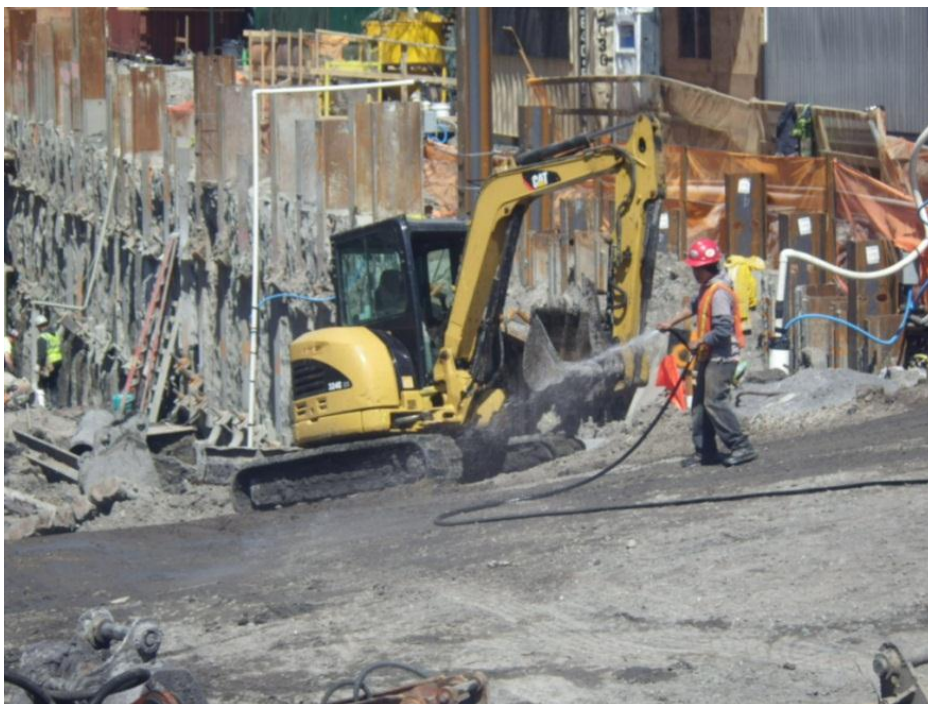
Photograph 21 – View of contractor implementing dust suppression. 5/7/2014
