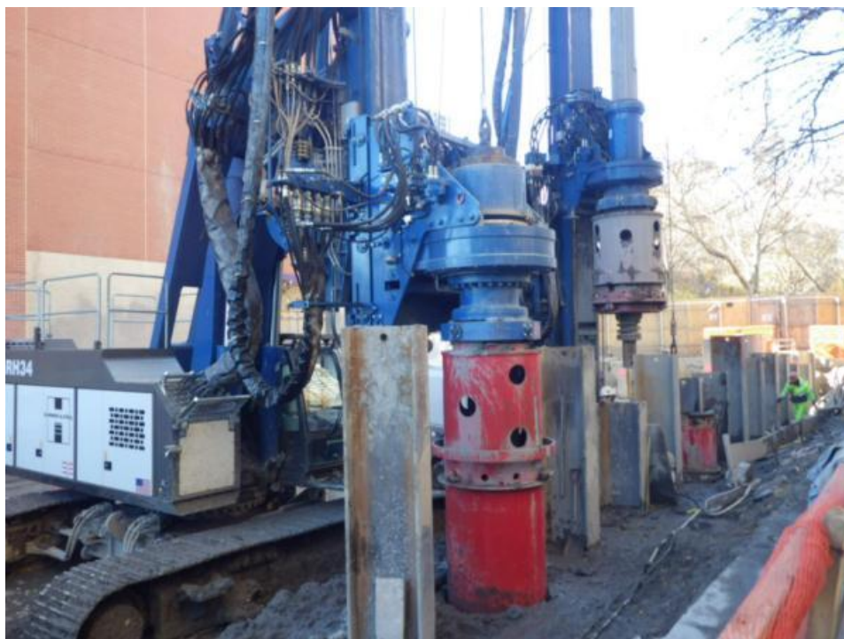
Photograph 10 – View of secant pile installation. 11/18/2013
