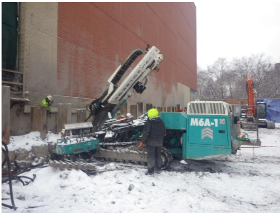
Photograph 13 – View of tieback installation. 2/18/2014
