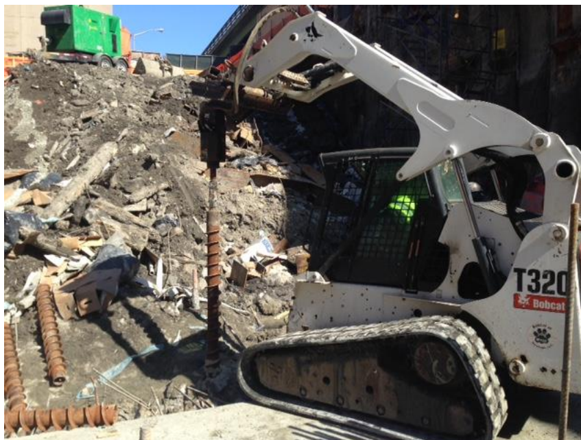
Photograph 22 – Drilling of on-site monitoring well using hollow-stem augers. 02/27/2015
