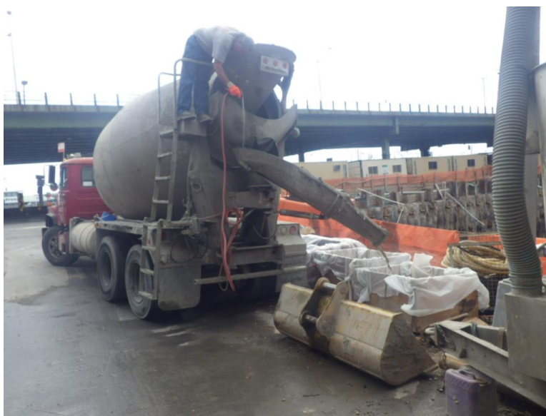
Photograph 4 –View of a concrete truck washing-out into a designated bin on 36 th street. 9/22/2014
