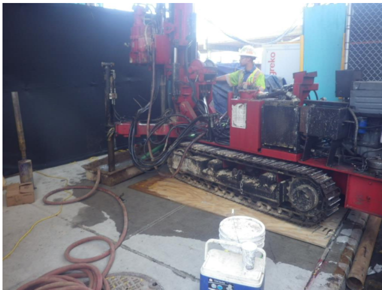
Photograph 5 – View of a piezometer well being drilled on 35 th street. 10/06/2014
