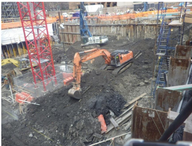
Photograph 17 – ECD moves material for ramp construction. 01/14/2015
