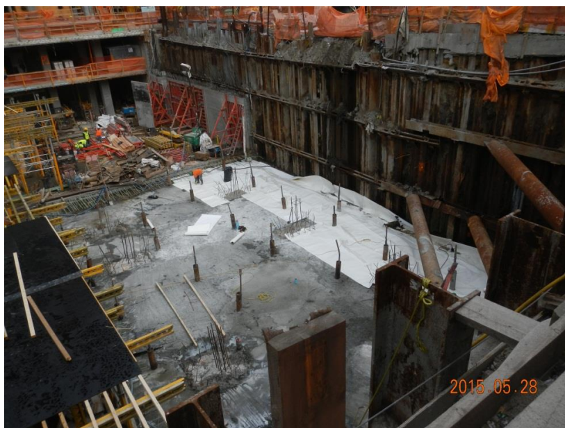
Photograph 34 – View of concrete mud slab installed at the base of Grids 5 and 6. SSC installs waterproofing membrane above the mud slab. 05/28/2015
