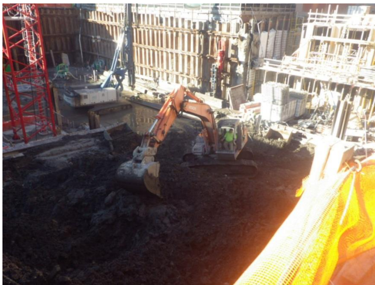
Photograph 13 – Stockpiled material in Grid 5 is moved for trucking off-site. 12/13/2014
