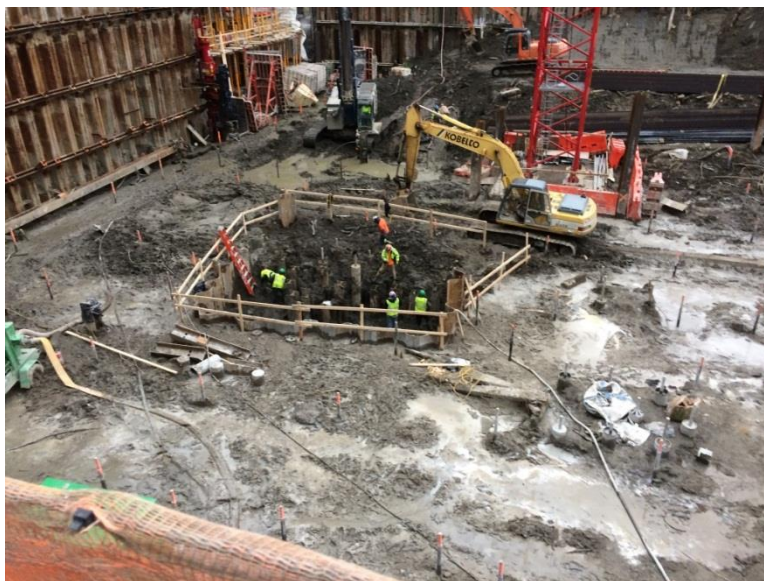
Photograph 15 – Excavation of the elevator shaft in Grids 16 and 17. 12/22/2014
