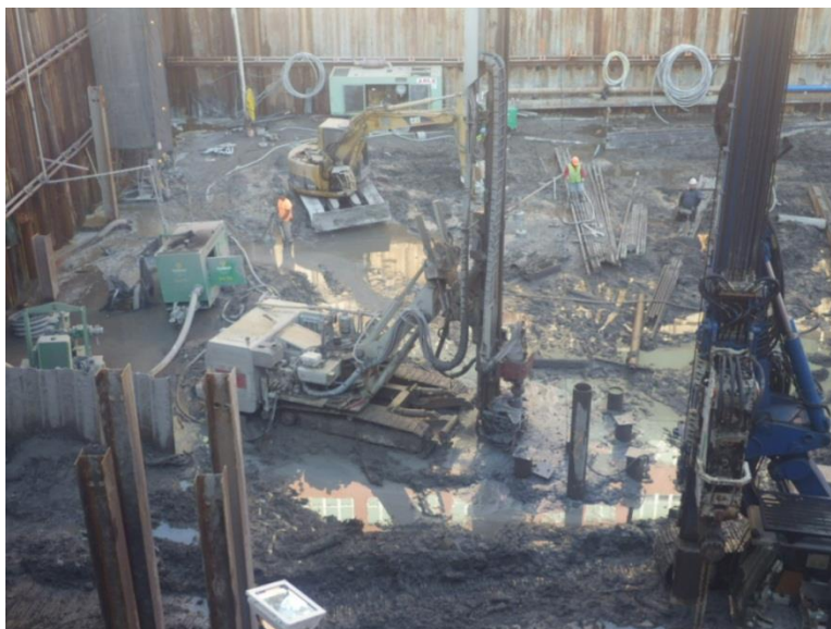
Photograph 9 – Structural caisson drilling. 11/10/2014
