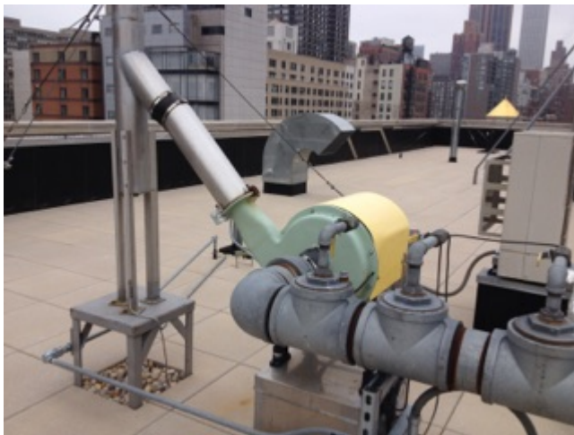
Photo 3: View of operational SSDS fan unit on the roof.
