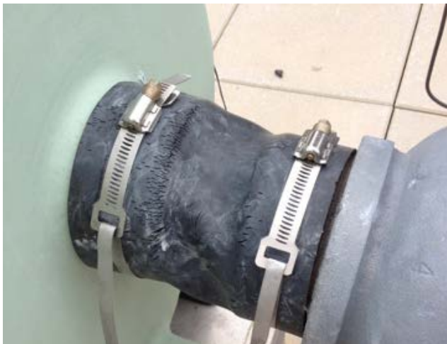
Photo 5: View of cracked flexible connector on the SSDS fan stack.
