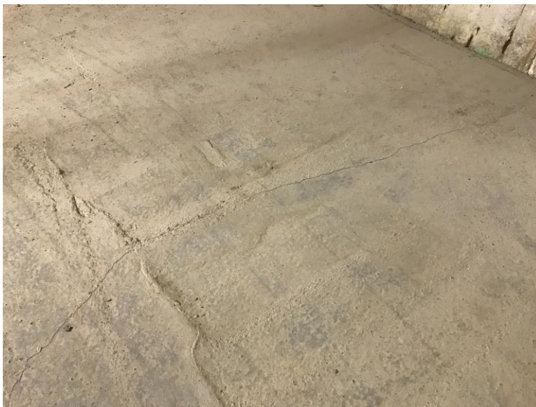
Photograph 13 – View of the superficial crack in concrete floor of the cellar in the East Tower; facing west. Dated 12/19/2017.
