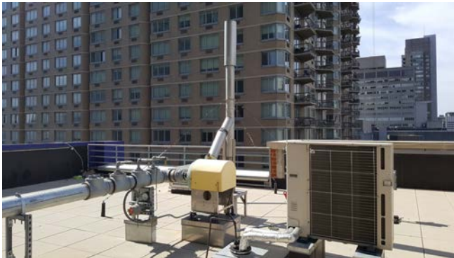
Photo 3: View of operational SSDS fan unit on the roof.
