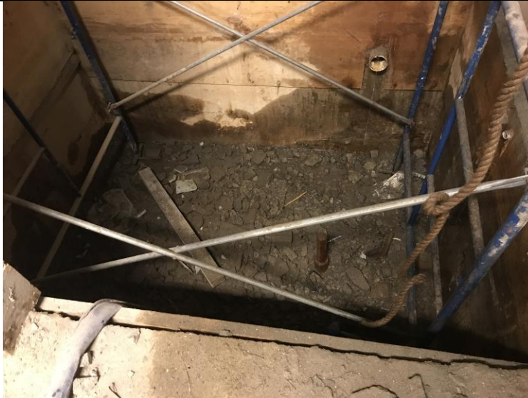
Photograph 9 – View of exposed tie down and concrete floor in the northwest cellar of the East Tower; facing west. Dated 12/19/2017.
