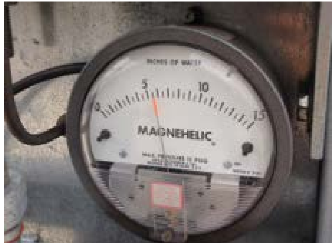
Photo 4: View of vacuum gauge associated with SSDS fan unit.
