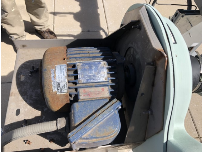
Photo 1: View of SSDS fan unit direct drive motor.
