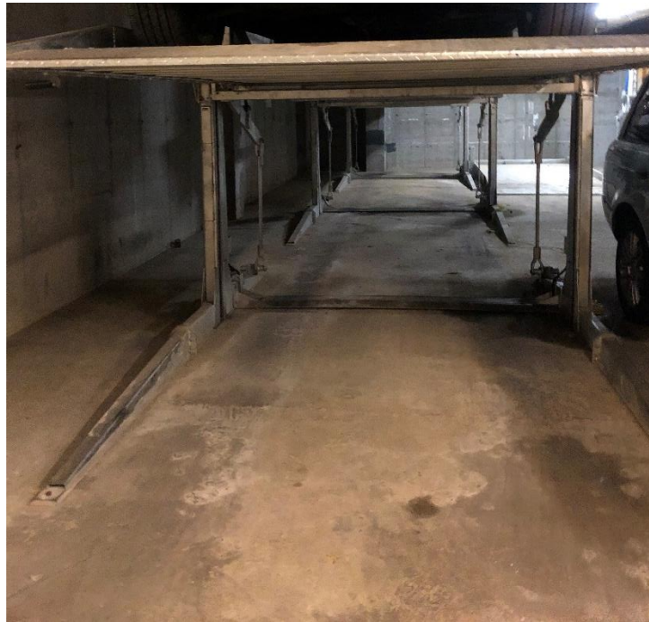
Photograph 6 - View of car lift in the cellar parking garage fastened with 3-inch bolts and sealed with epoxy; facing north. Dated 12/20/2019.
