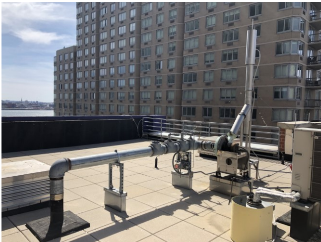
Photo 3: View of SSDS fan unit on the roof.
