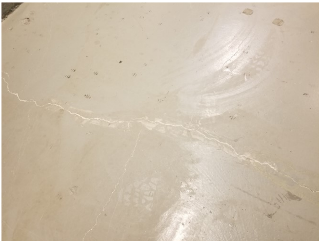
Photo 5: View of typical sealed hairline crack in Room 110.
