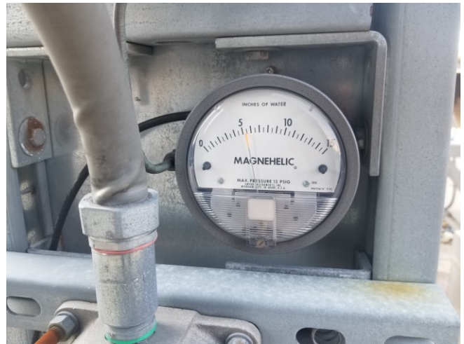
Photo 4: View of vacuum gauge for the SSDS fan unit.
