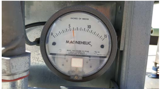
Photo 4: View of vacuum gauge associated with SSDS fan unit.
