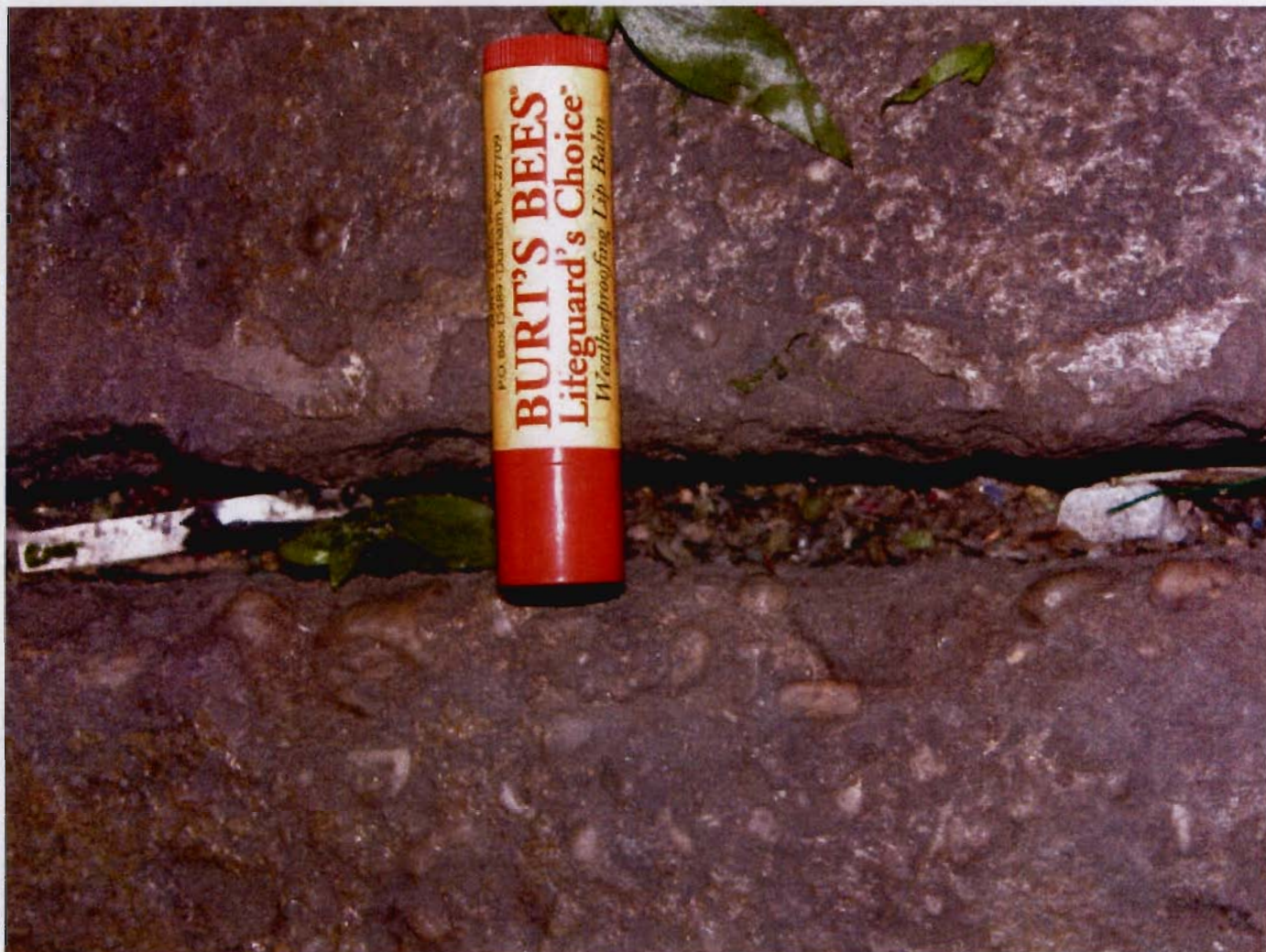
Floor crack near the florist work area in the first floor florist shop.
