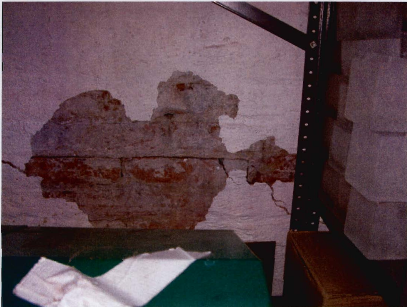
Wall cracks observed in the first floor florist space on the western wall of the Gasser Building.
