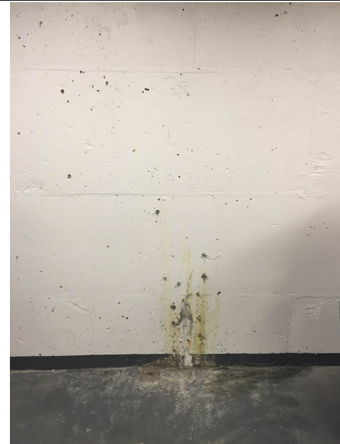
Location 1 – After repair.
