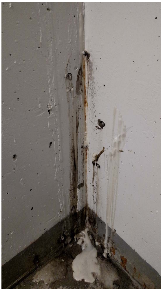
Photograph 1. Grout Repair in Stained Area (Northeast Corner of Fan Room)
