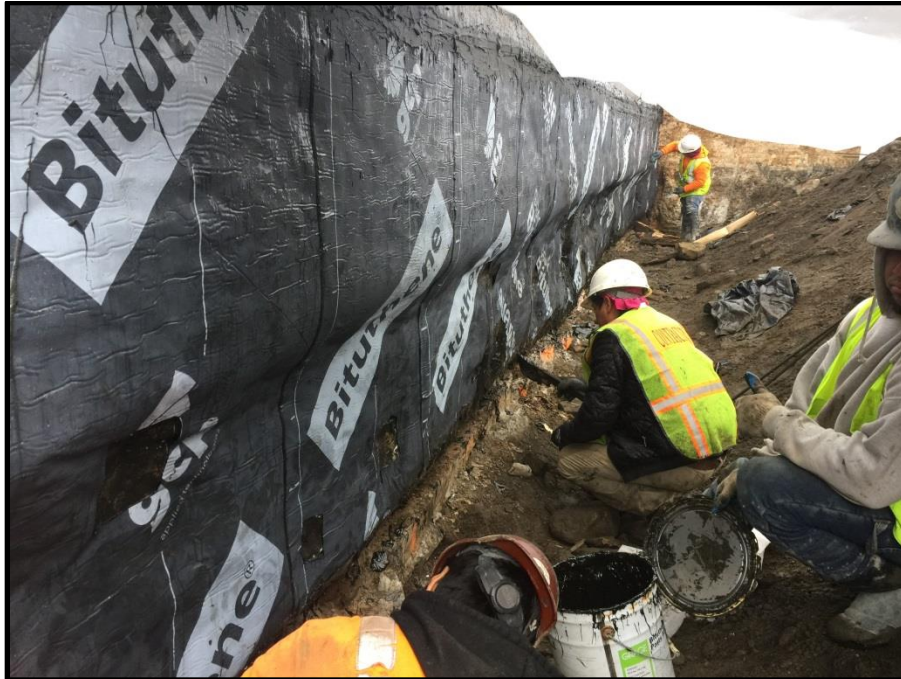
Photo 1: Contractor repairing the Bituthene membrane along the west wall (facing north)
