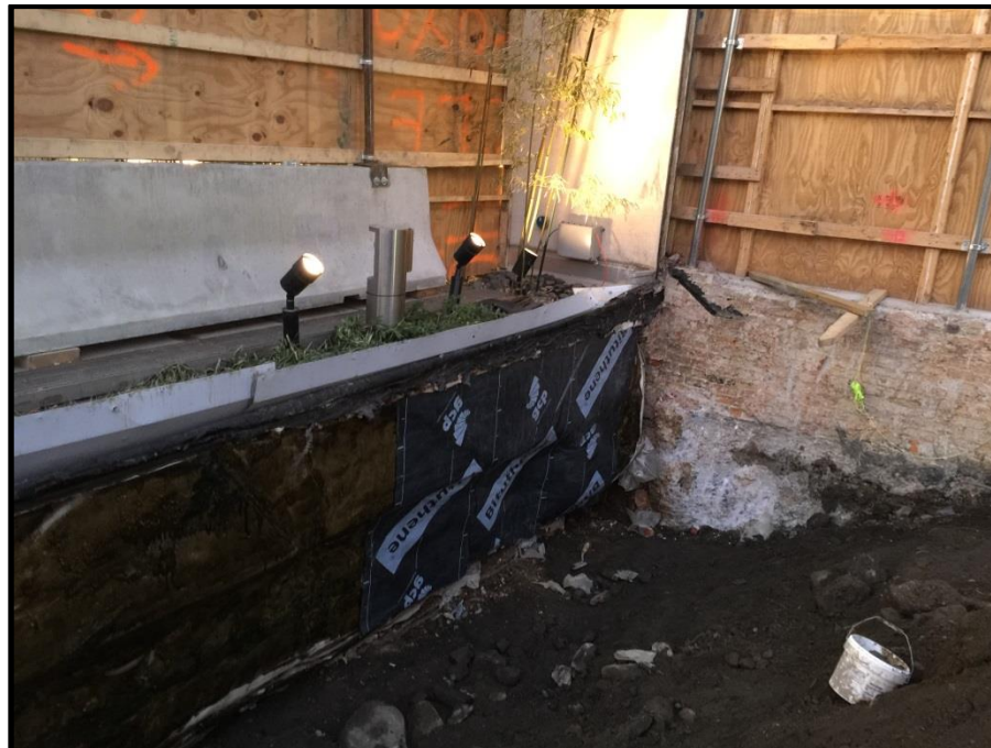
Photo 2: End of waterproofing work for the day (facing northwest).
