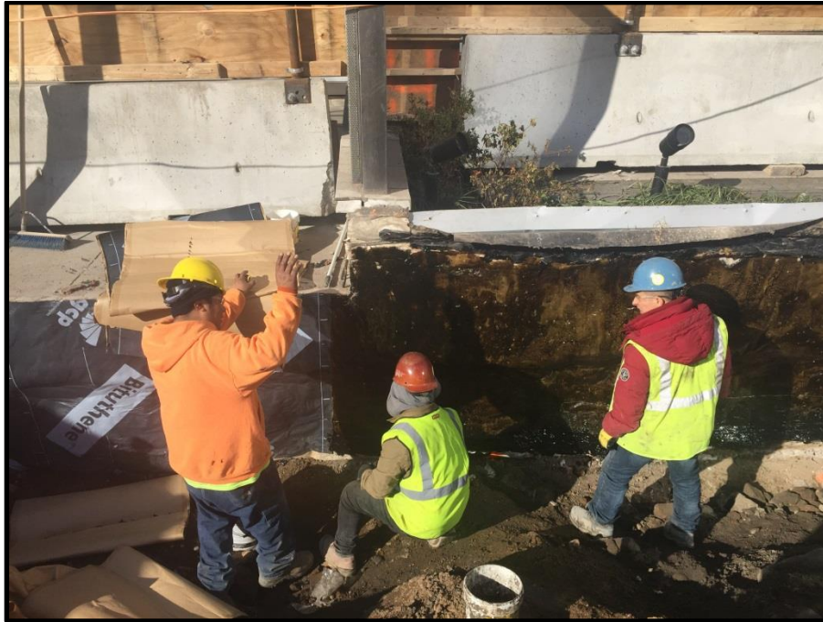
Photo 1: Contractor installing Bituthene membrane over the west wall (facing west)
