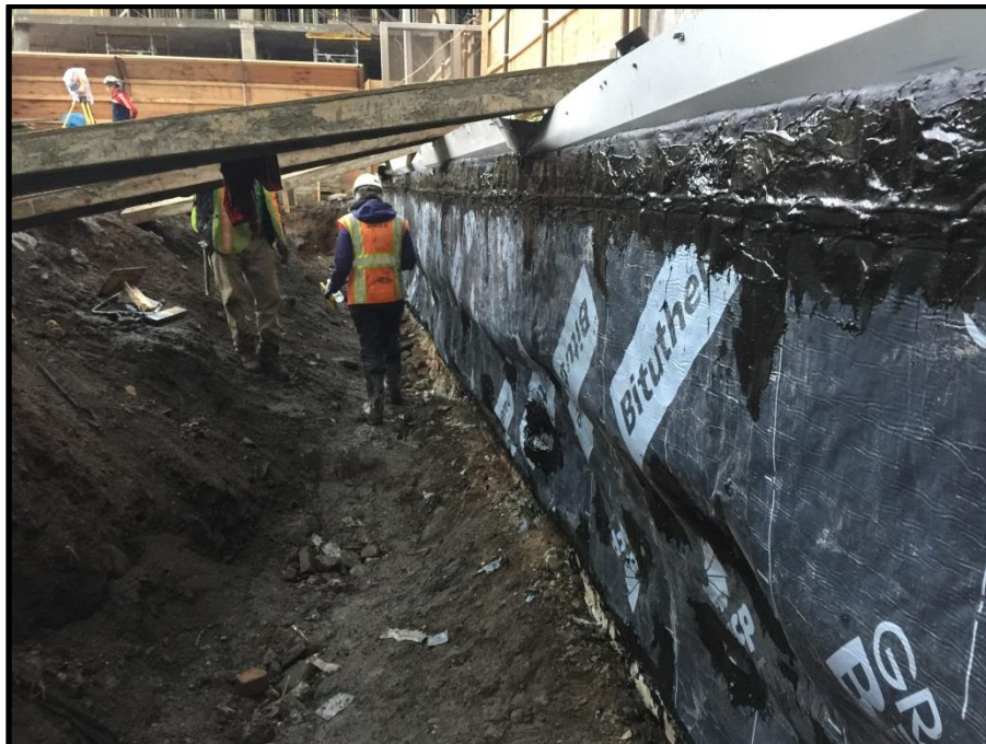
Photo 2: MRCE engineer inspecting completed waterproofing (facing south)
