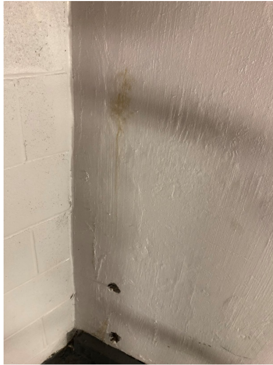
Photograph 1. New Evidence of Active Water Infiltration on Foundation Wall in Northwest Stairwell (February 7, 2019)
