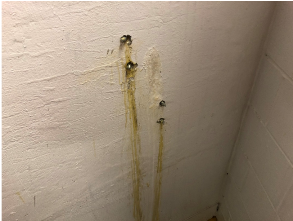
Photograph 2. 2018 Grout Injection Location (February 7, 2019)
