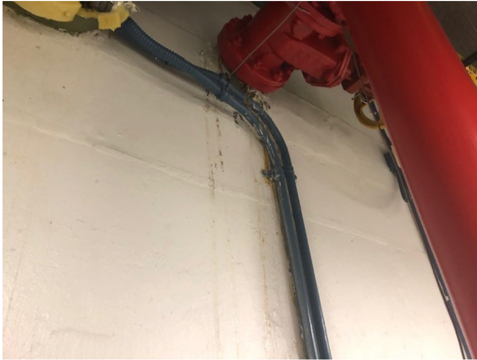
Photograph 7. Fire Main Pipe Penetration in Foundation Wall after Grout Injection (February 21, 2019)
