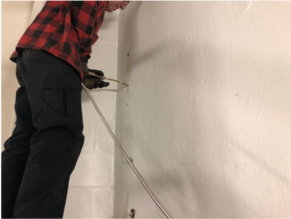
Photograph 5. Grout Injection around Water Infiltration Stain in Northwest Stairwell (February 21, 2019)
