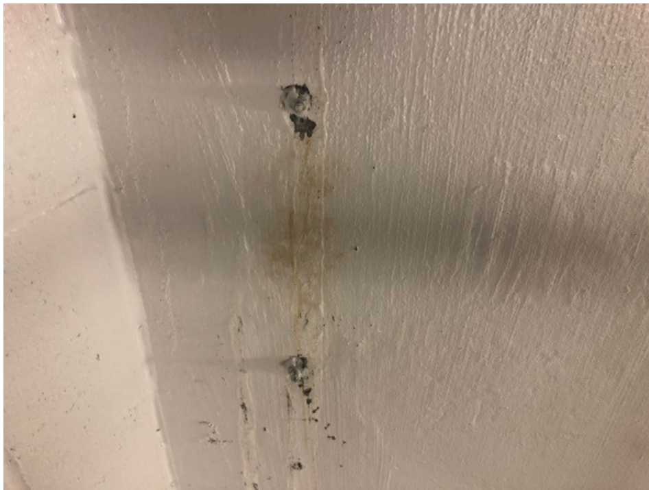
Photograph 8. Water Infiltration Stain in Northwest Stairwell after Grout Injection (February 21, 2019)
