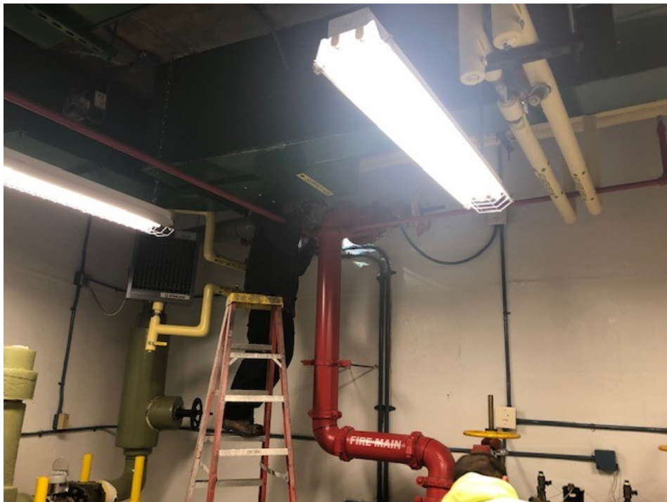
Photograph 6. Starbrite Drilling Holes for Grout Injection around Fire Main Pipe Penetration in Foundation (February 21, 2019)
