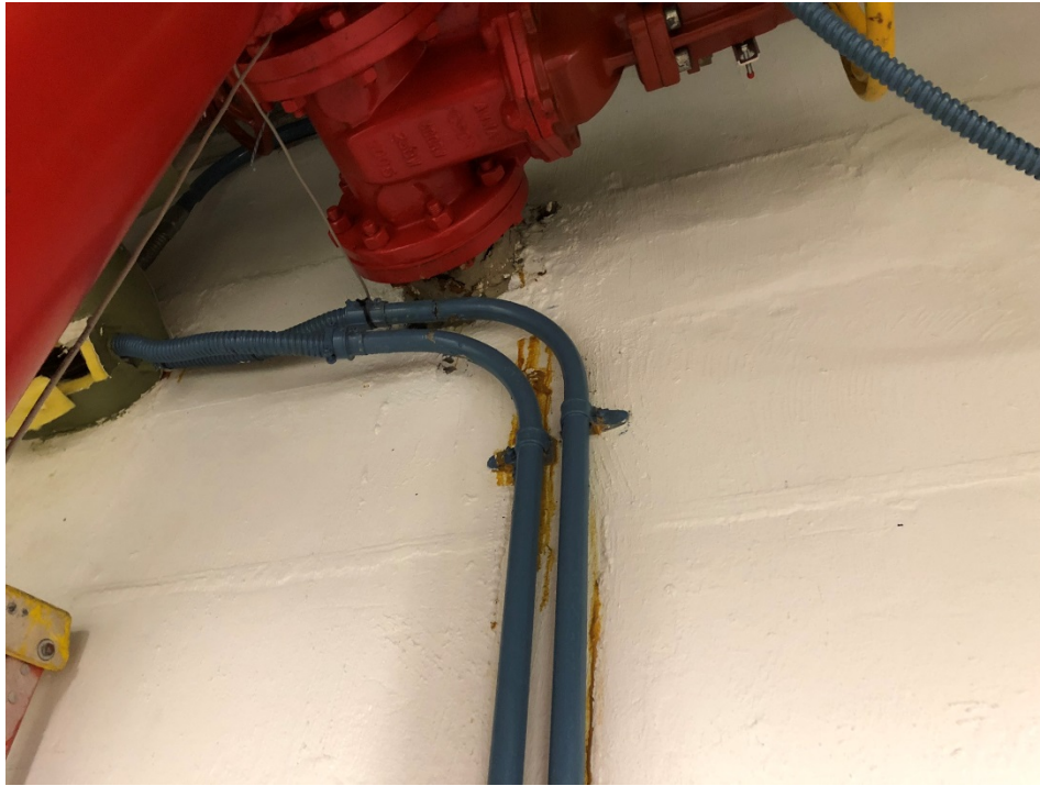
Photograph 3. Leaking Fire Main Pipe Penetration (February 7, 2019)
