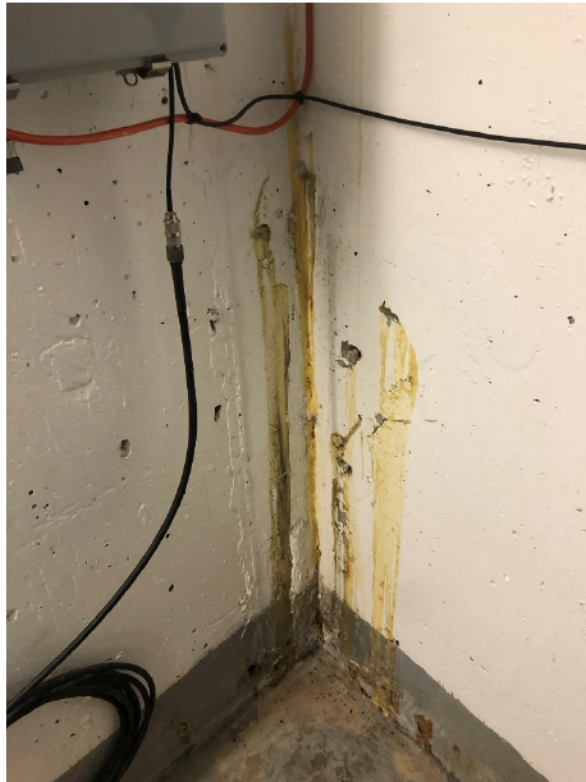
Photograph 1. Previous Grout Injection from 2020 in South Lobby AC Room (January 19, 2021)
