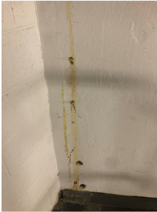
Photograph 3. Previous Grout Injection from 2019 in Northwest Stairwell (January 19, 2021)
