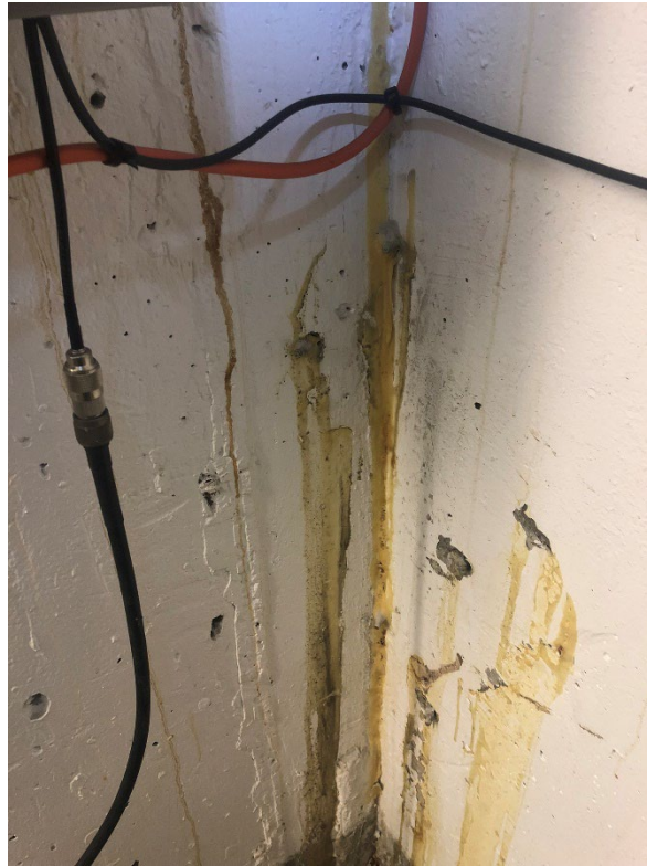
Photograph 1. Previous Grout Injection from 2020 in South Lobby AC Room (February 9, 2022).
