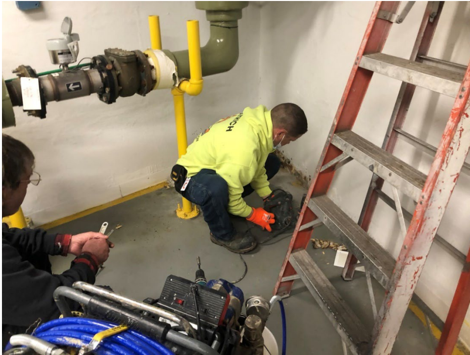
Photograph 3. Grout Injection in Corner of North Water Meter Room (March 10, 2022).
