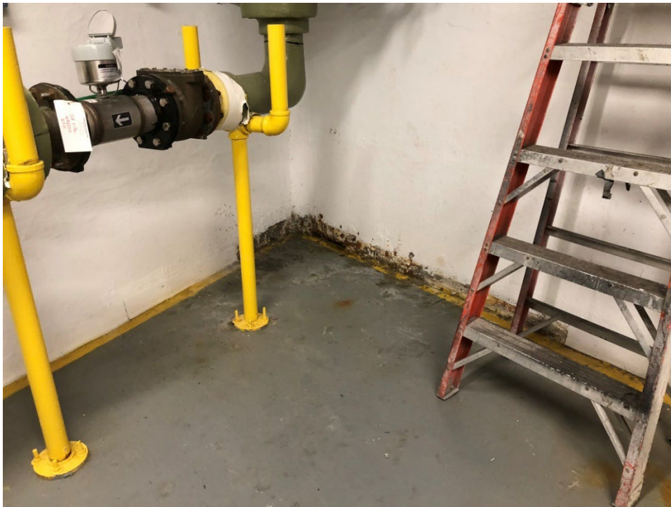
Photograph 4. Completed and Cleaned Grout Injection Location in North Water Meter Room (March 10, 2022).
