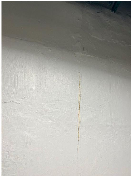
Photograph 2. Staining Evidence of Water Infiltration in North Water Meter Room (January 25, 2023).
