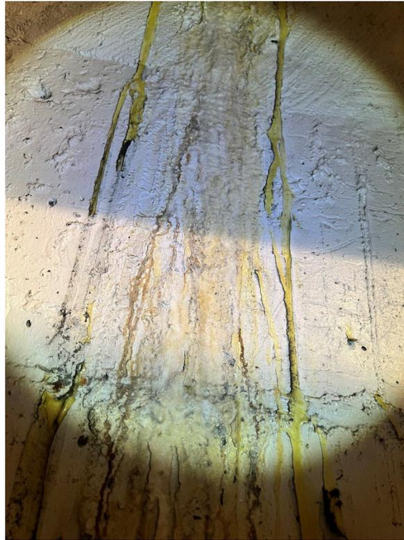
Photograph 3. Evidence of Water Infiltration and Efflorescence in South Lobby AC Unit Room (January 25, 2023).
