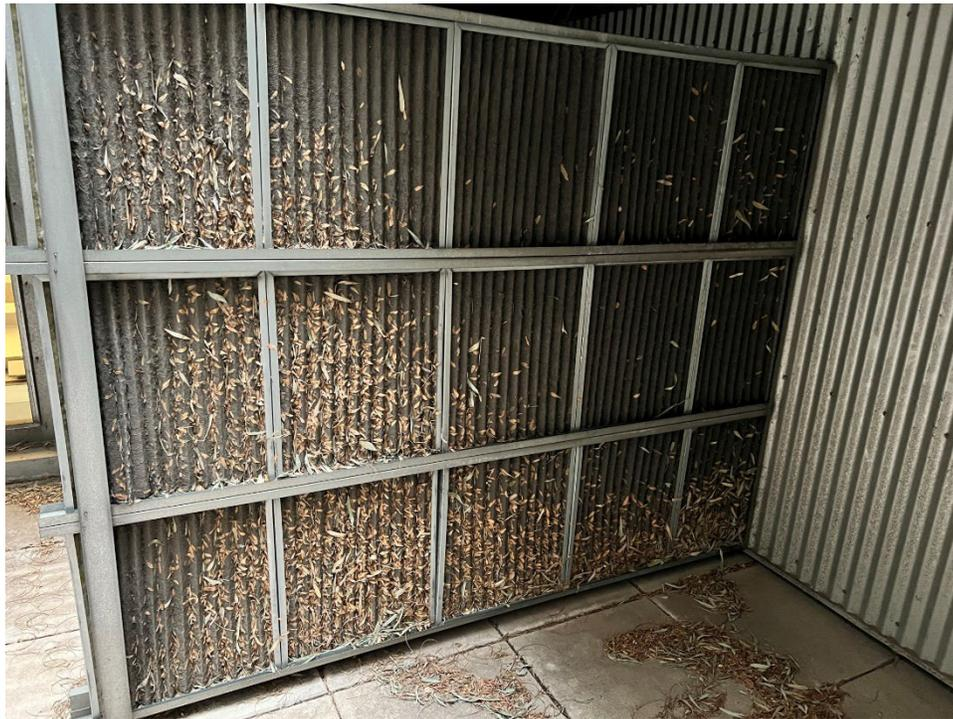
Photograph 4. GSF-C-1 Intake Filters Clogged with Debris and Dust (January 25, 2023).
