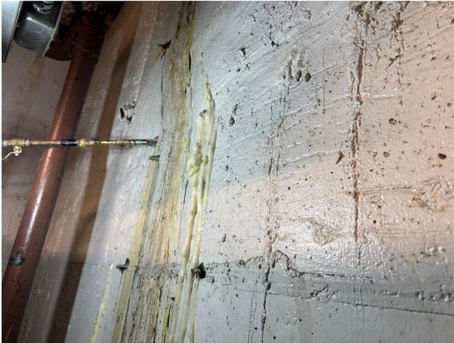
Photograph 5. Grout Injection in South Lobby AC Unit Room Wall (February 17, 2023).
