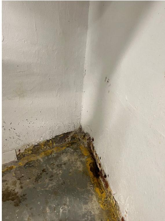
Photograph 1. Previous Grout Injection from 2022 in Corner of North Water Meter Room (January 25, 2023).
