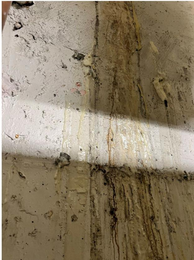
Photograph 6. Completed Grout Injection in South Lobby AC Unit Room Wall (February 17, 2023).
