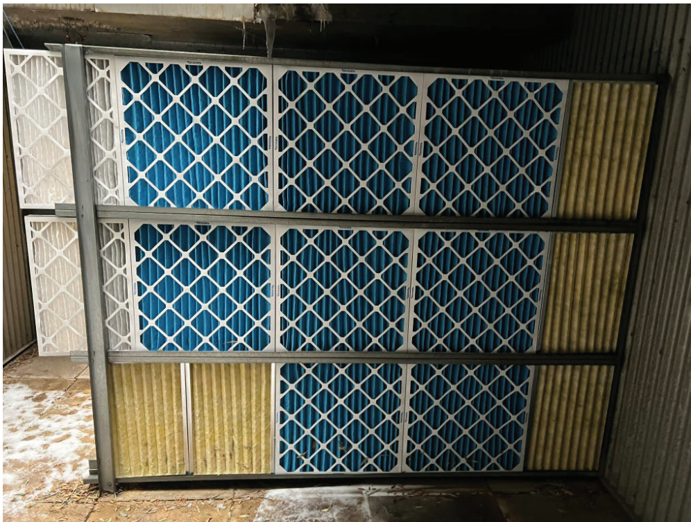
Photograph 4. GSF-C-1 New Intake Filters Replaced Before Inspection (January 19, 2024).
