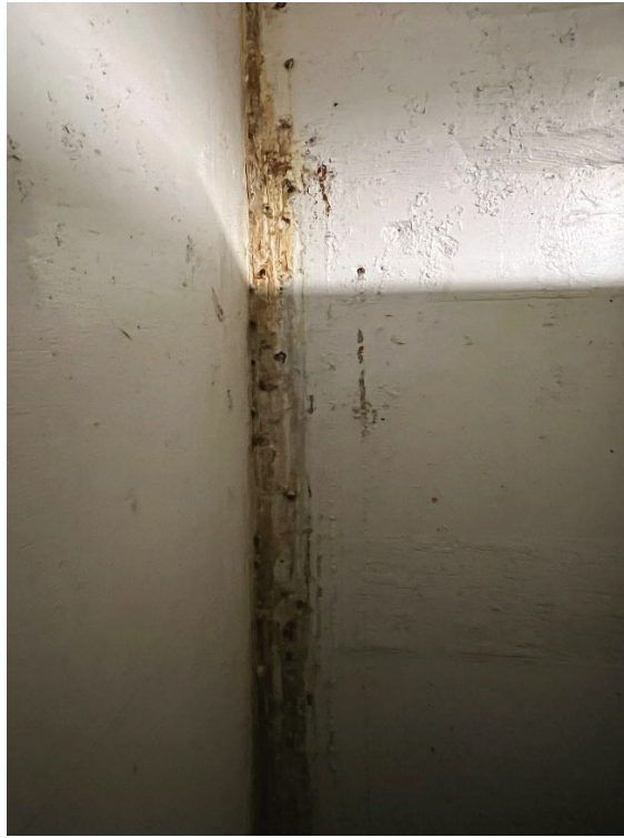
Photograph 5. Completed 2024 Grout Injection in Corner of South Lobby AC Unit Room Wall (February 21, 2024).
