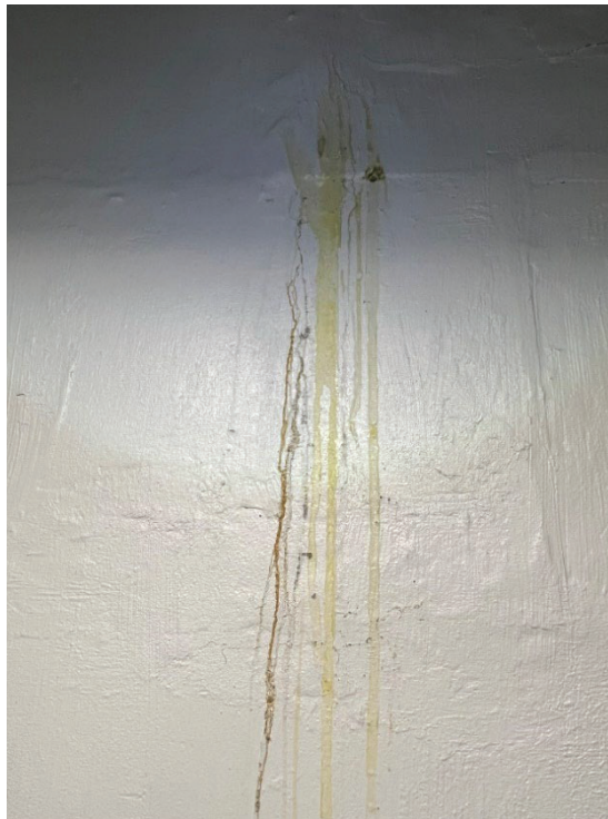
Photograph 2. Previous Grout Injection from 2023 in West Wall of North Water Meter Room (January 19, 2024).
