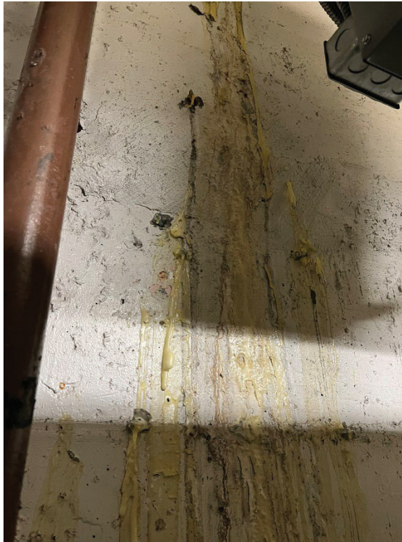
Photograph 1. Previous Grout Injection from 2023 in South Lobby AC Unit Room (February 21, 2024).
