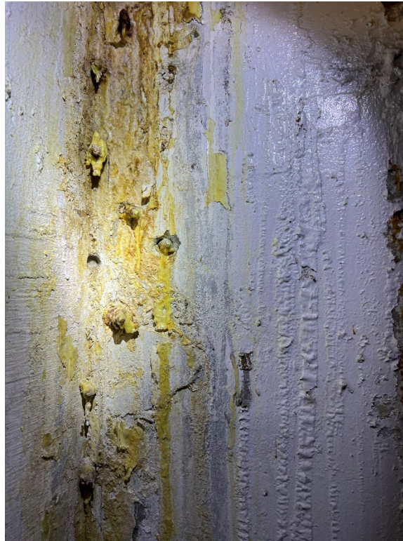
Photograph 1. Closeup of Previous Grout Injection from 2024 in South Lobby AC Unit Room (January 24, 2025).
