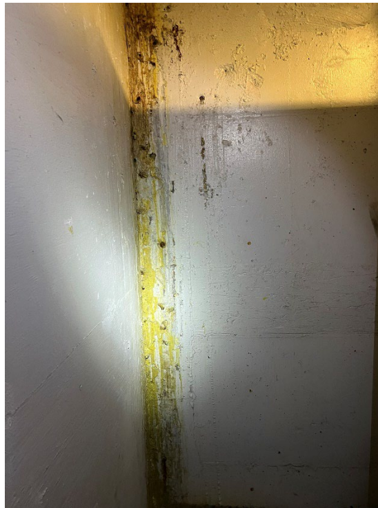
Photograph 2. Previous Grout Injection from 2024 in South Lobby AC Unit Room (January 24, 2025).
