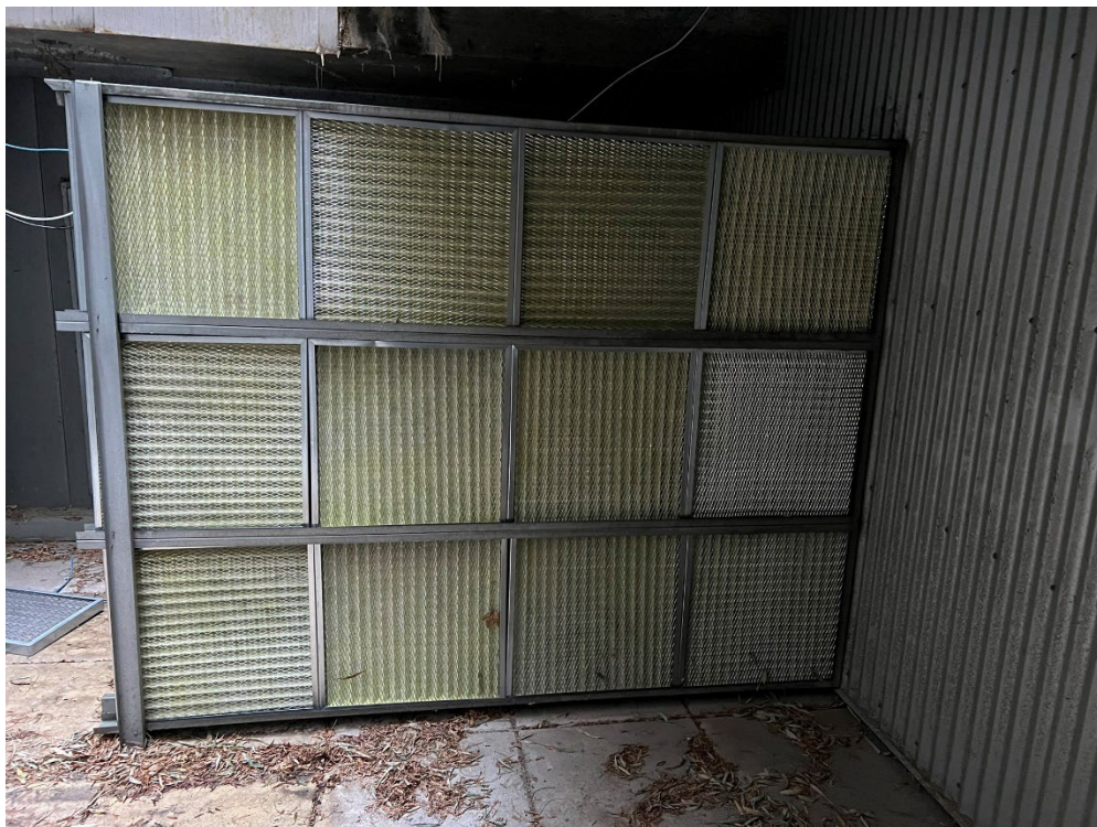
Photograph 4. GSF-C-1 New Intake Filters (January 24, 2025).
