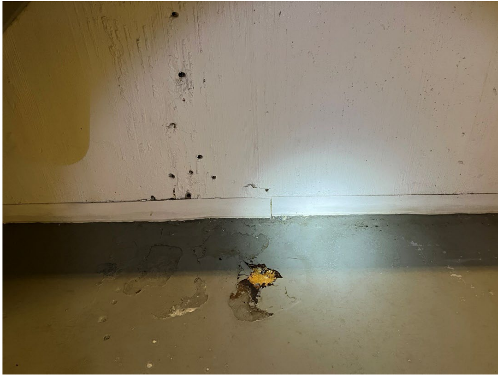
Photograph 7. Cracking in Floor Paint in North Hallway due to Grout Injection in Foundation Wall Above. (January 24, 2025).
