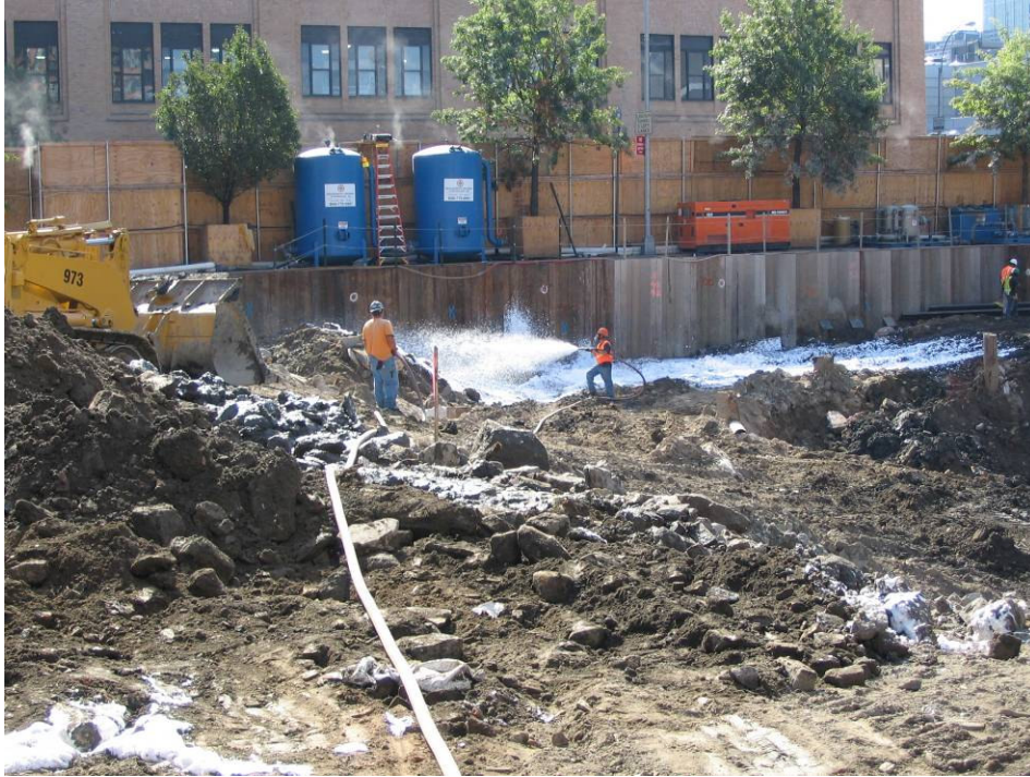
Photograph No. 41: September 12, 2005 - Workers keeping area along eastern end of Site covered with foam (area where USTs were discovered).
