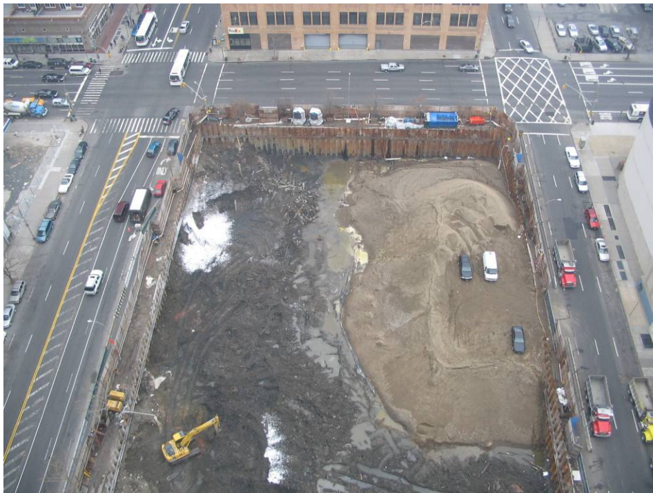
Photograph No. 90: January 11, 2006 - Aerial view of site (view east) from RiverPlace I 32 nd floor observation deck. Note RCA stockpile along southern perimeter.
