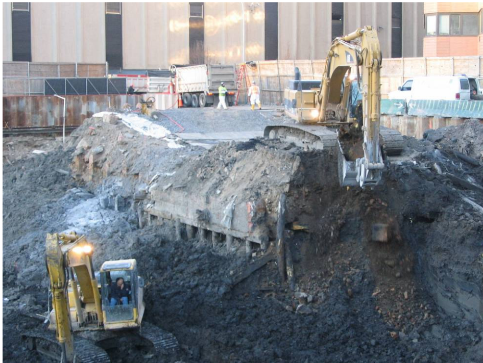
Photograph No. 102: January 27, 2006 – Excavating the former Purifying House foundation (view south-southwest).
