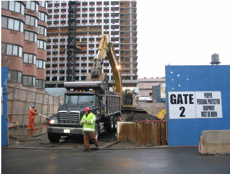
Photograph No. 105: January 31, 2006 - Washing truck down at Gate 2 before exiting Site.
