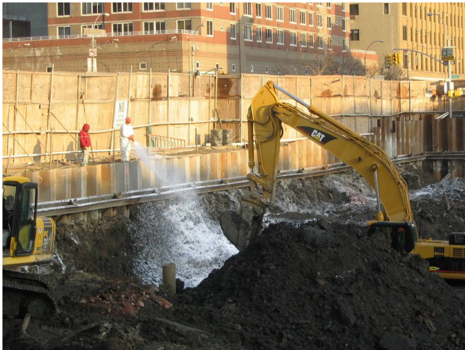
Photograph No. 86: January 9, 2006 - Foaming during excavation along northern sheeting line.
