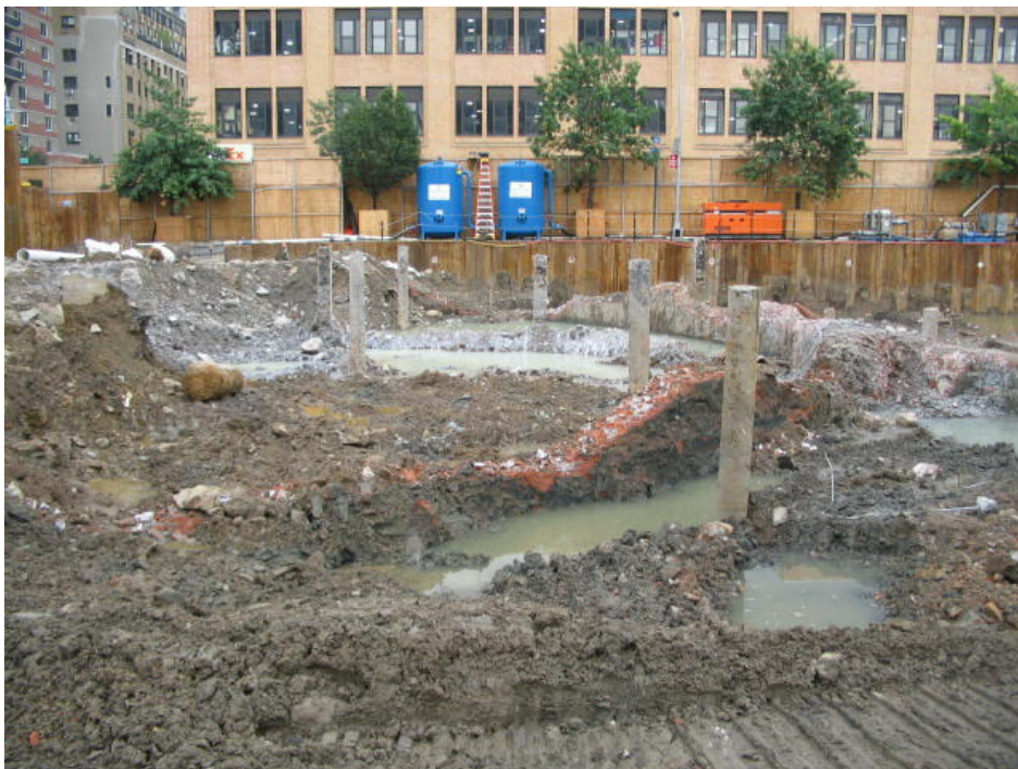
Photograph No. 23: August 16, 2005 - No. 2 filter sand being placed around screened interval of dewatering well during well installation.
