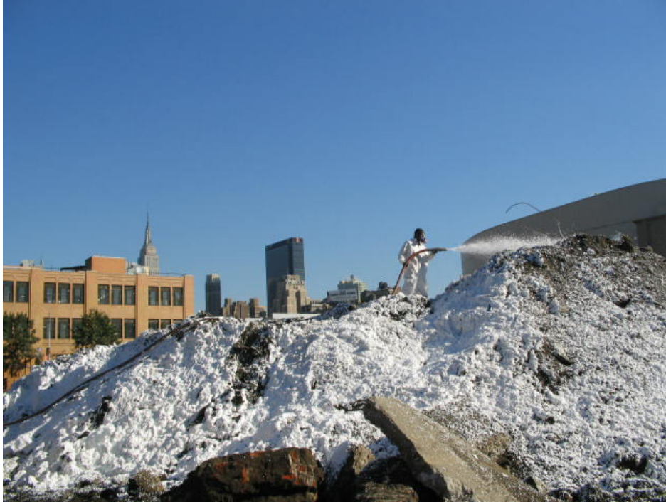
Photograph No. 37: September 7, 2005 - Worker covering material stockpile with foam.
