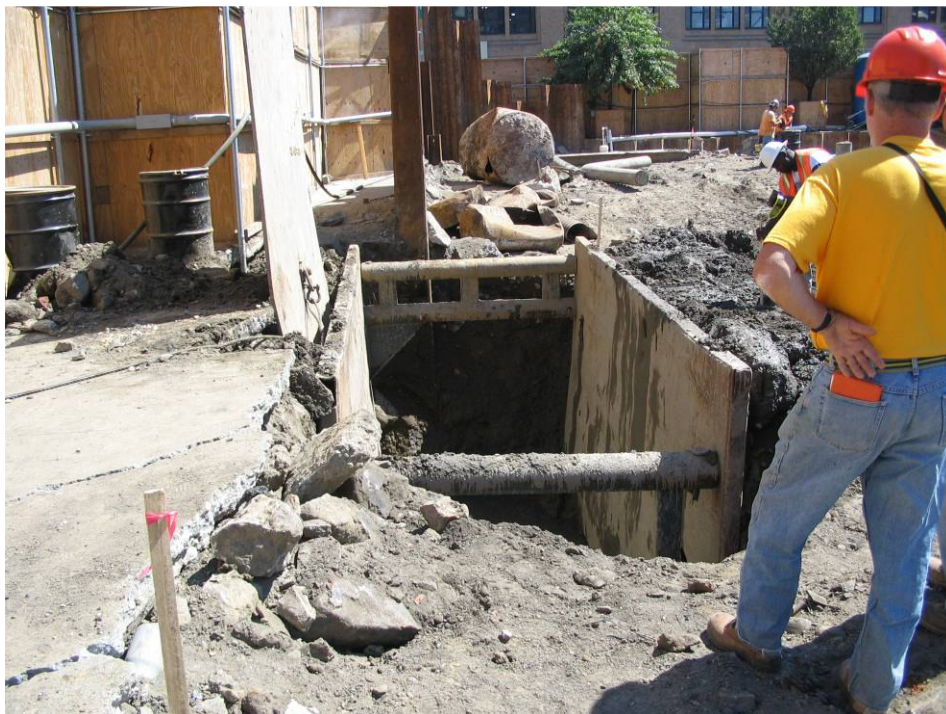
Photograph No. 40: September 10, 2005 - Another view of the trench box excavation.
