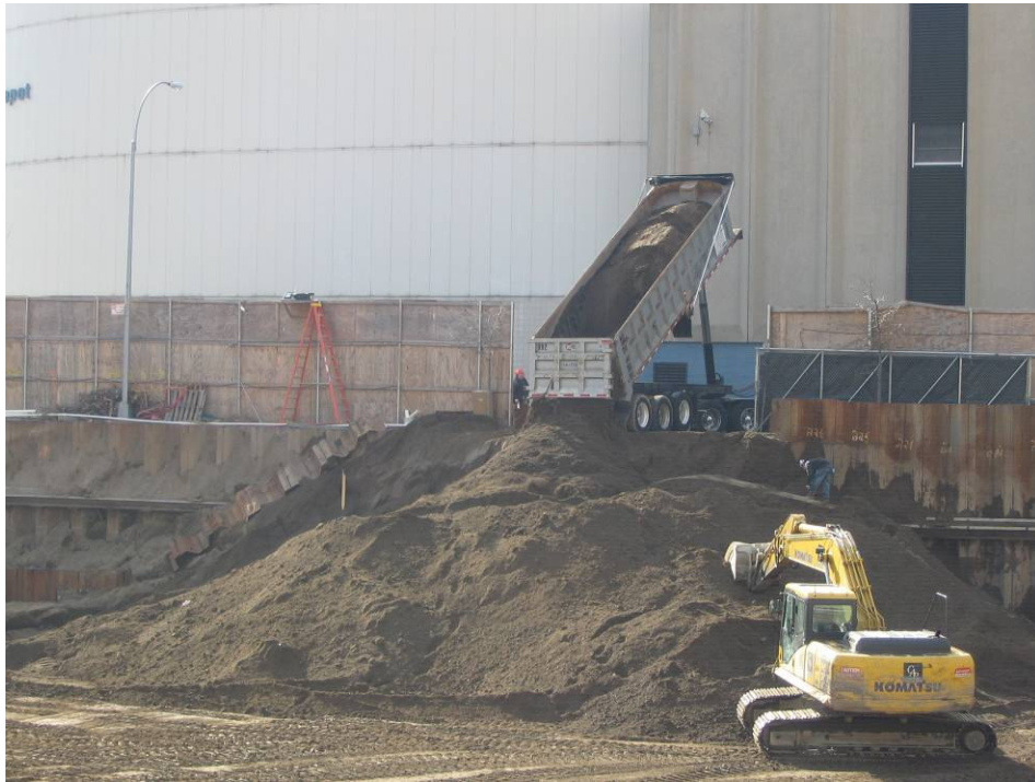
Photograph No. 109: February 8, 2006 – View of RCA delivery through Gate 4 (view south).
