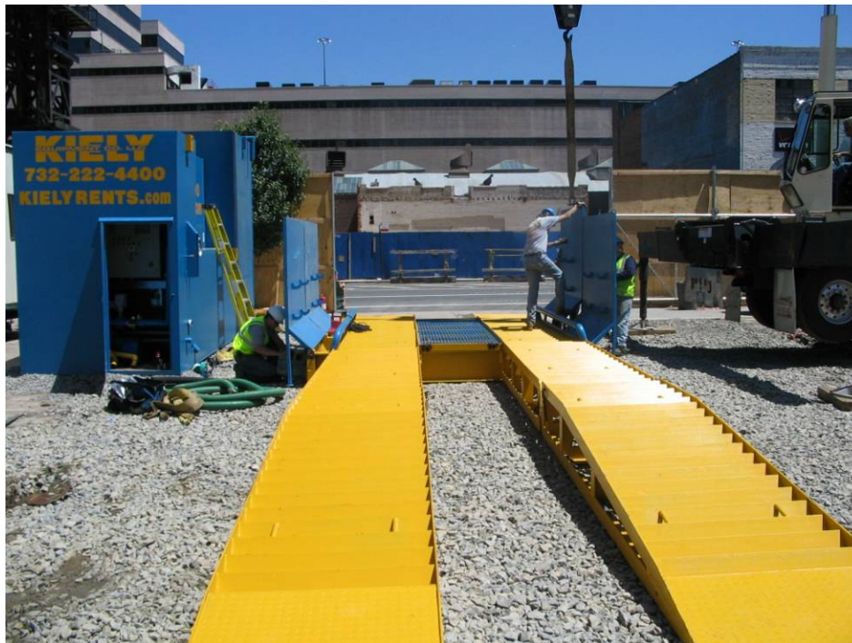
Photograph No. 8: June 2005 - Assembling the truck wash (view north onto West 42 nd Street).
