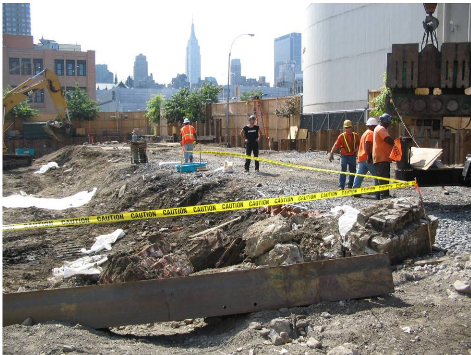
Photograph No. 18: August 10, 2005 - An early version of zone demarcation using caution tape (view towards southeast). Note decontamination pools present at zone boundary.
