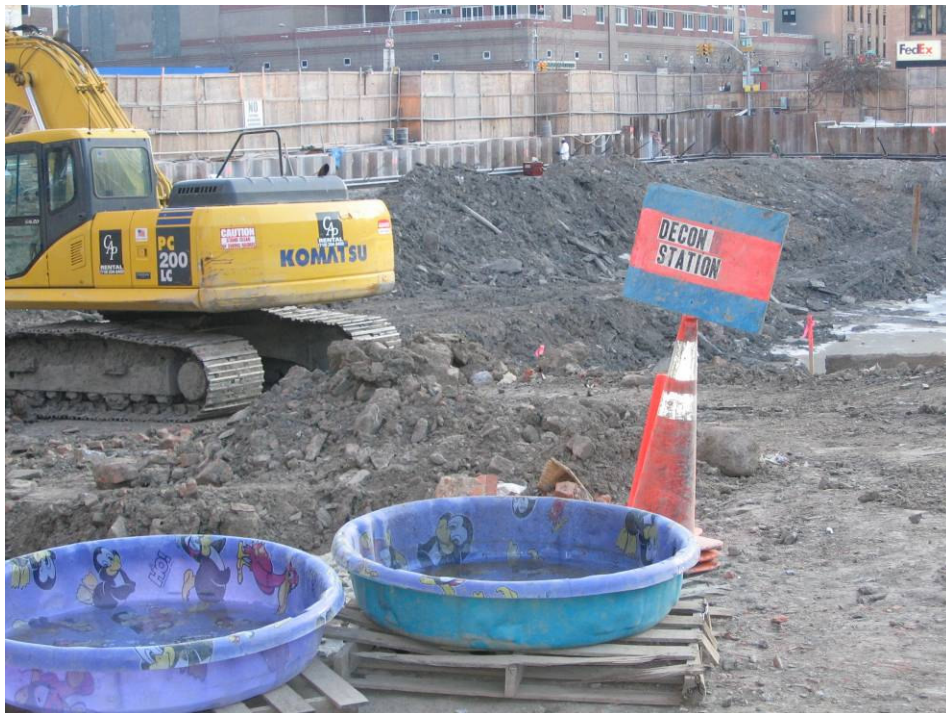
Photograph No. 84: View of the decontamination station at the exit of the Site exclusion zone.
