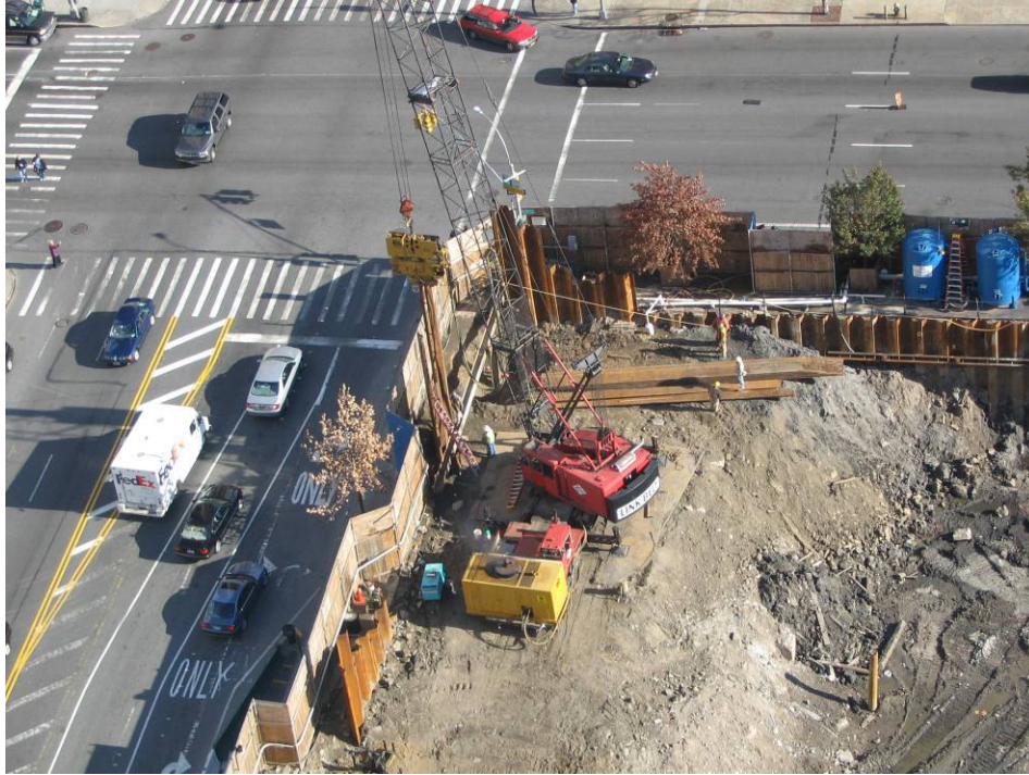
Photograph No. 79: November 11, 2005 - Close-up aerial view of site (view east) from RiverPlace I 32 nd floor observation deck. View is of sheeting installation occurring along northern perimeter.
