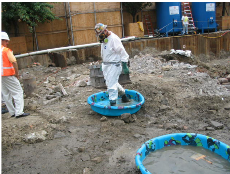
Photograph No. 30: August 31, 2005 - Workers decontaminating PPE (boots) in decon pools.
