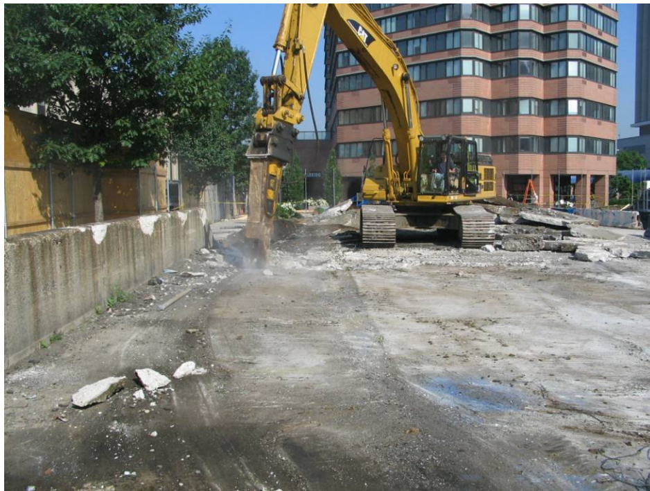
Photograph No. 4: June 2005 - Working to remove existing surface materials (view west).
