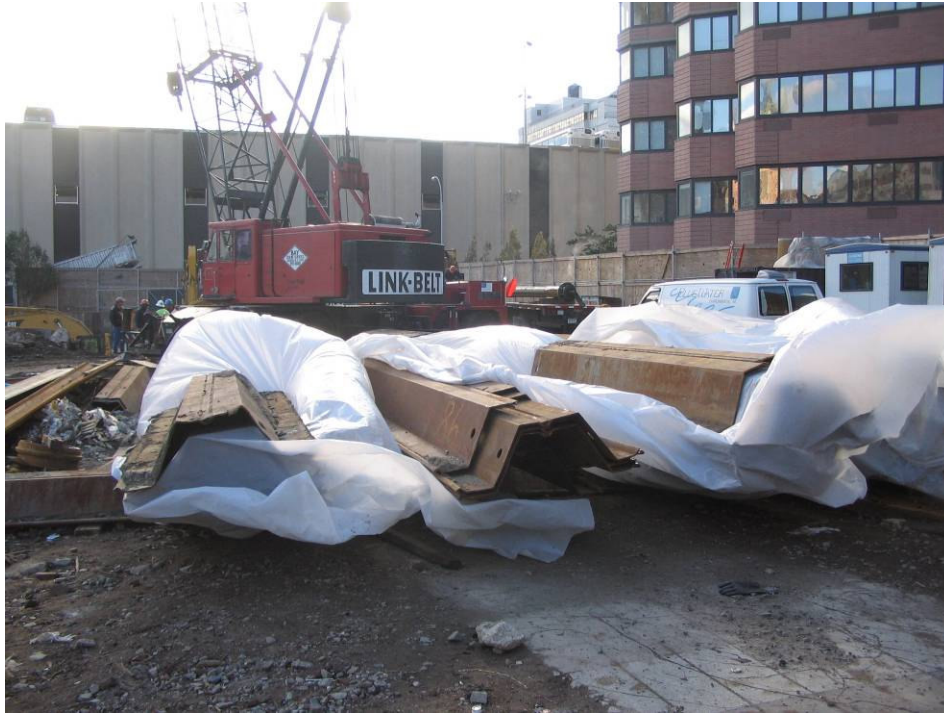
Photograph No. 77: November 10, 2005 - Sheeting sections (pieces to be installed along northern perimeter) staged for use with plastic sheeting to keep them dry.
