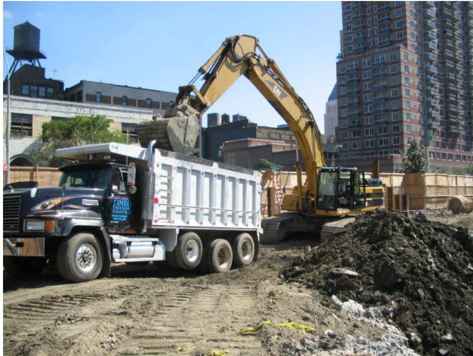
Photograph No. 35: September 6, 2005 - View of material load-out in progress.
