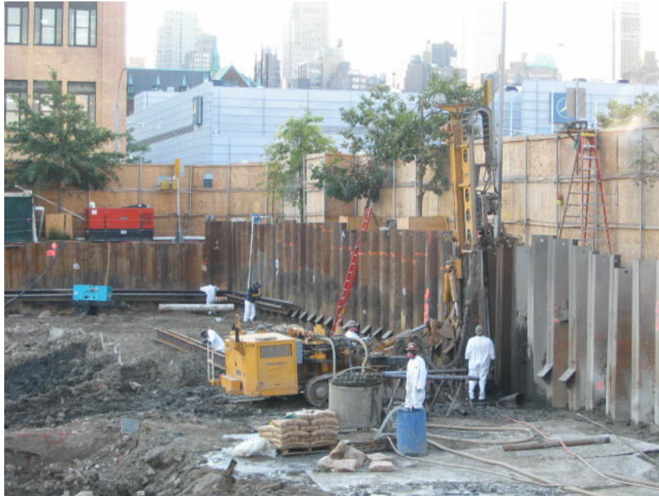
Photograph No. 53: September 25, 2005 - View of Moretrench performing toe pin installation.
