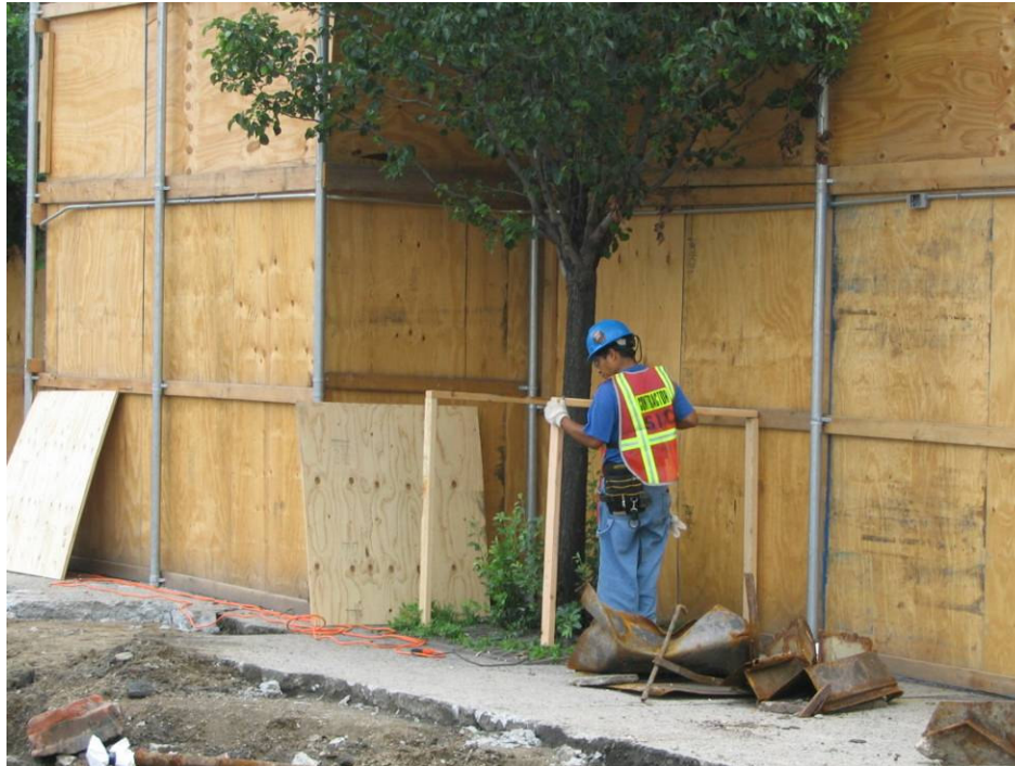
Photograph No. 7: June 2005 - Assembling plywood barriers around on-site tree trunks.
