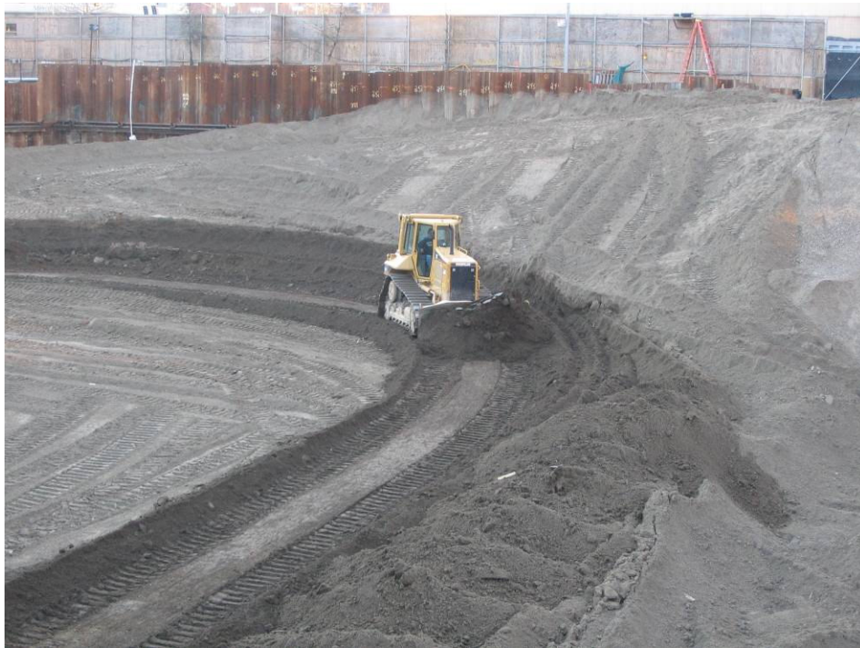
Photograph No. 100: January 26, 2006 – The bulldozer in action spreading out RCA.
