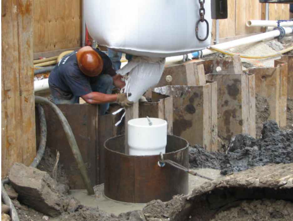
Photograph No. 23: August 16, 2005 - No. 2 filter sand being placed around screened interval of dewatering well during well installation.
