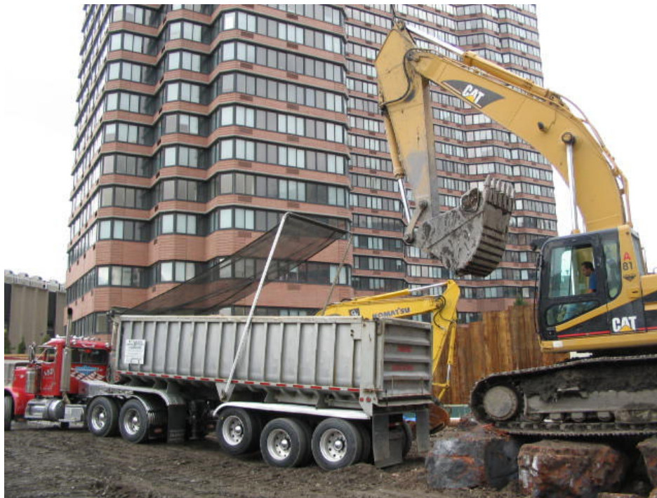
Photograph No. 46: September 16, 2005 - View showing mesh tarp being installed over top of material load within truck bed. A solid tarp is subsequently installed over the top of the mesh tarp.
