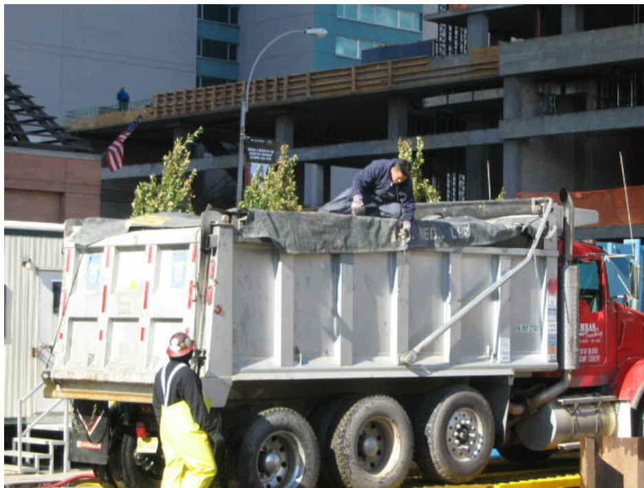
Photograph No. 70: October 28, 2005 - Trucker installing solid tarp over material load before departing from Site.
