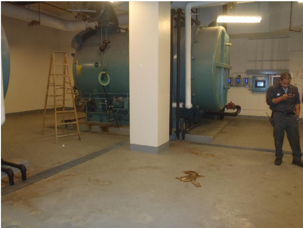
Photograph No. 4: View of surface cover inside the boiler room of River Place II.
