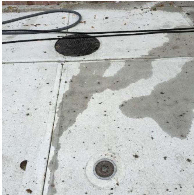
Photo 21: Fill port on 41 st Street sidewalk.
