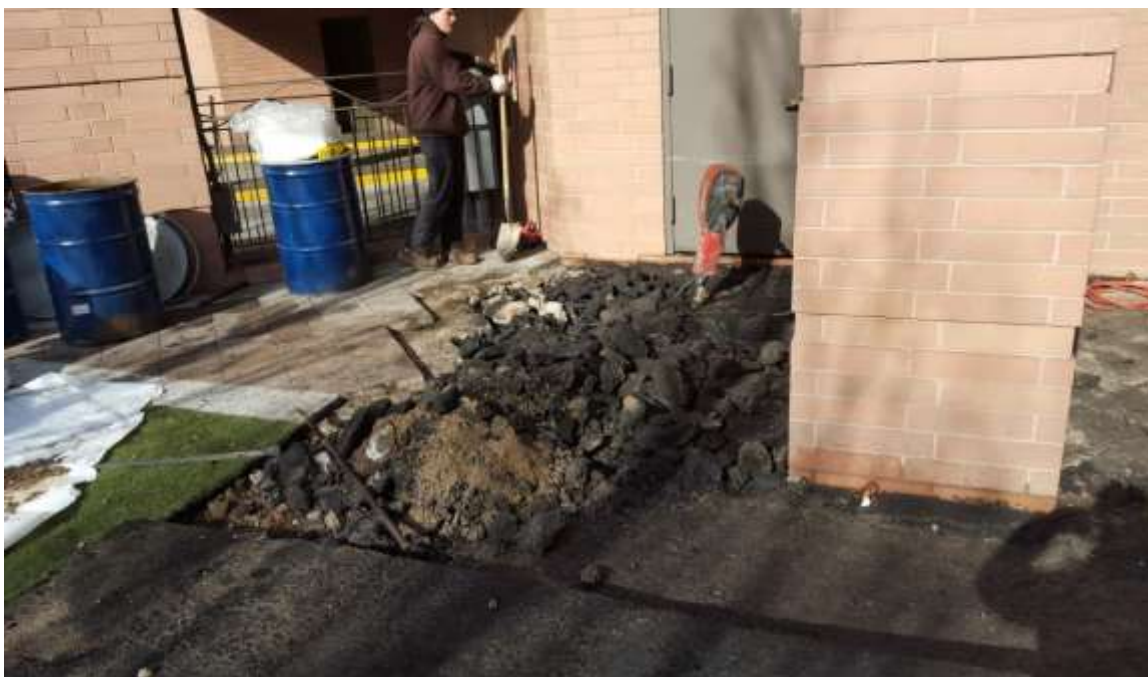
Photograph 4: View of impacted material removal
