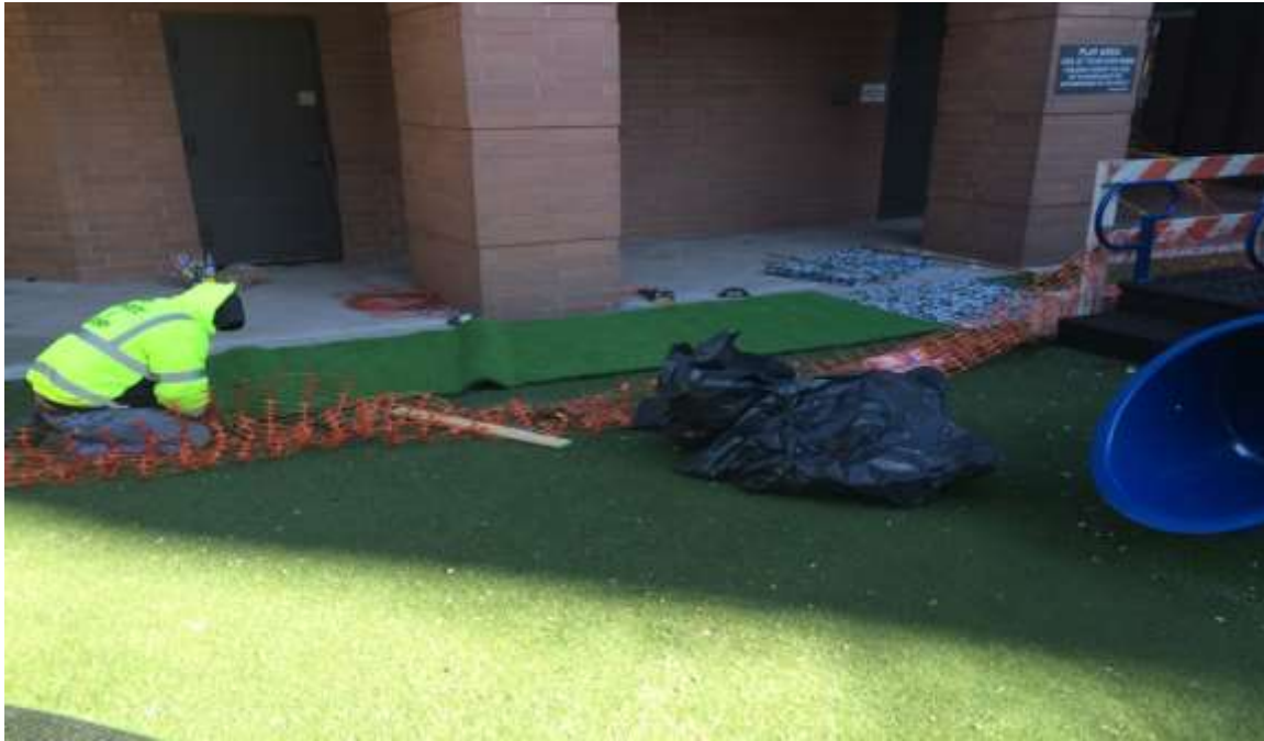
Photograph 9: View of restored paver stone walkway.
