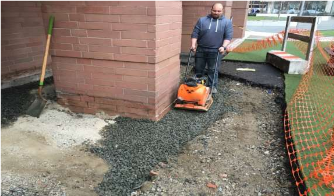
Photograph 7: View of backfill (i.e. ¾-inch quarry stone) compaction.
