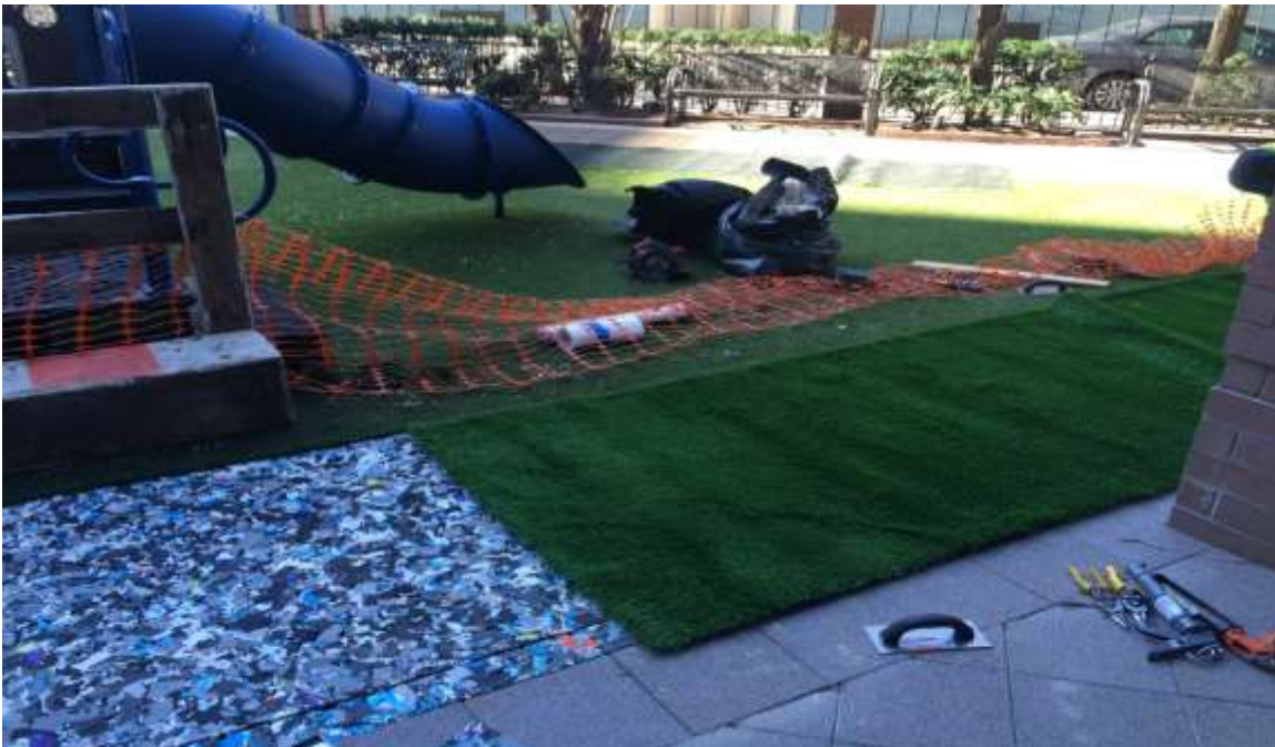
Photograph 8: View of new composite foam and turf in playground area.
