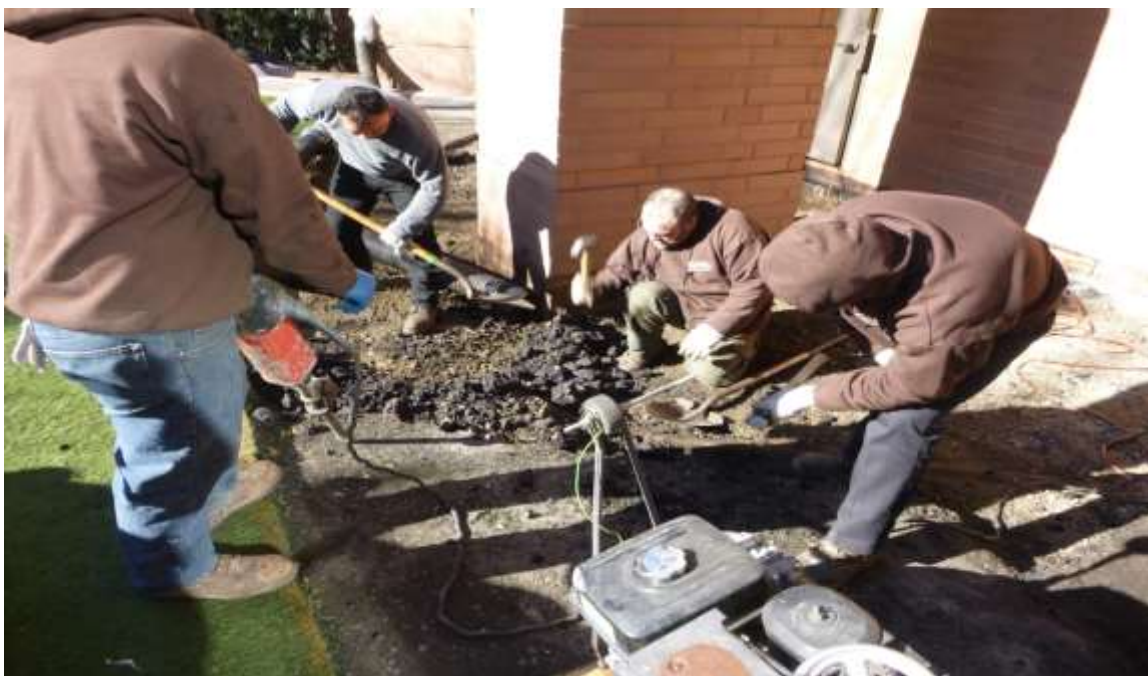
Photograph 6: View of impacted material removal.
