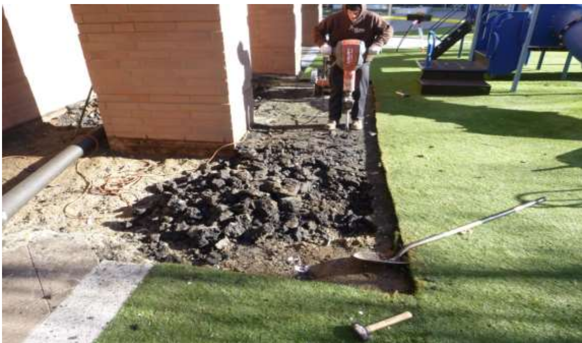
Photograph 5: View of impacted material removal.
