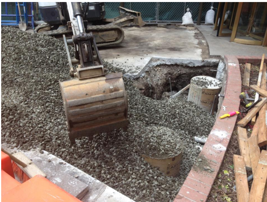
Photo 8: View of backfilling activity using 3/4-inch stone; facing southeast. (04/25/2016)
