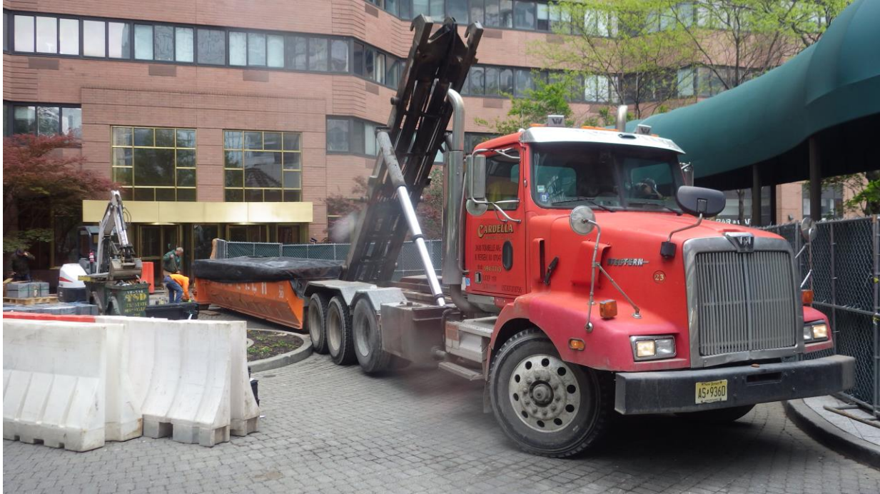
Photo 13: View of material removal activity; facing north. (05/05/2016)
