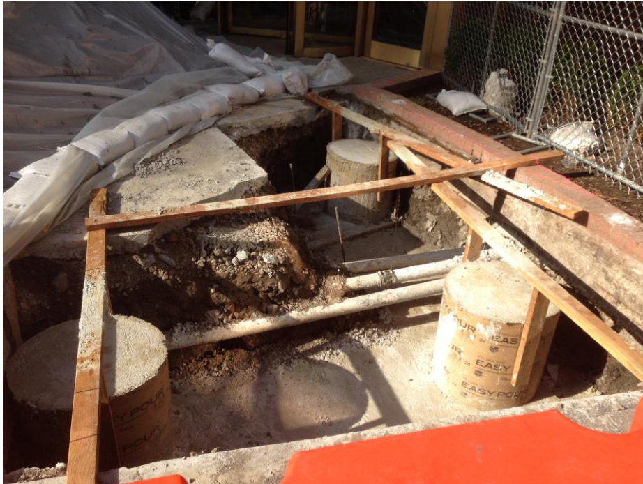
Photo 5: View of concrete backfill in the western excavation area; facing southeast. (04/25/2016)
