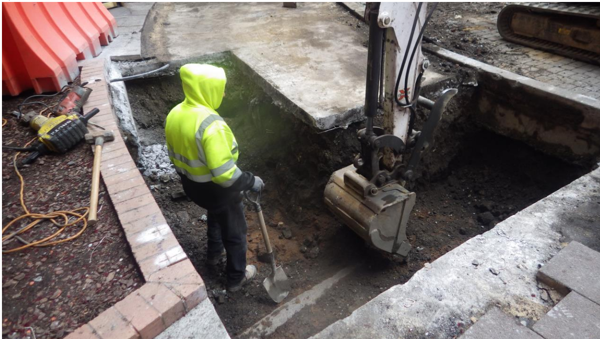
Photo 11: Excavation activity on the eastern portion of the Site; facing northwest. (05/05/2016)
