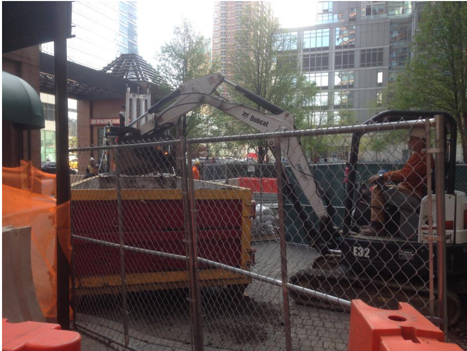
Photo 7: View of material loading and disposal activity; facing east. (04/25/2016)
