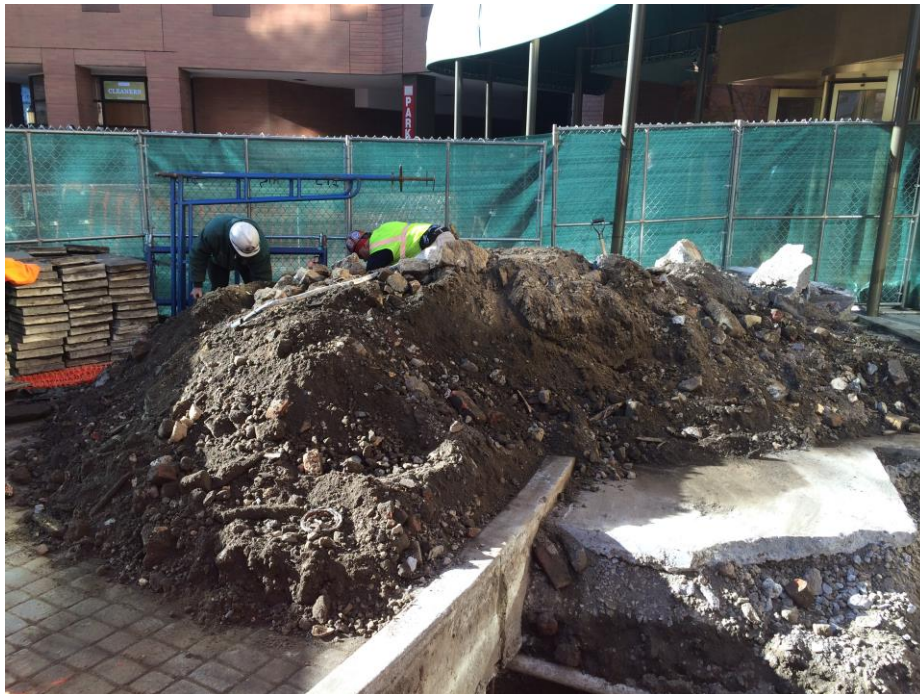
Photo 3: View of stockpiled material adjacent to the western excavation area; facing southeast. (4/21/2016)
