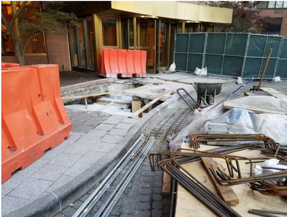
Photo 15: View of eastern excavation area backfilled with concrete, facing southwest. (05/12/2016)
