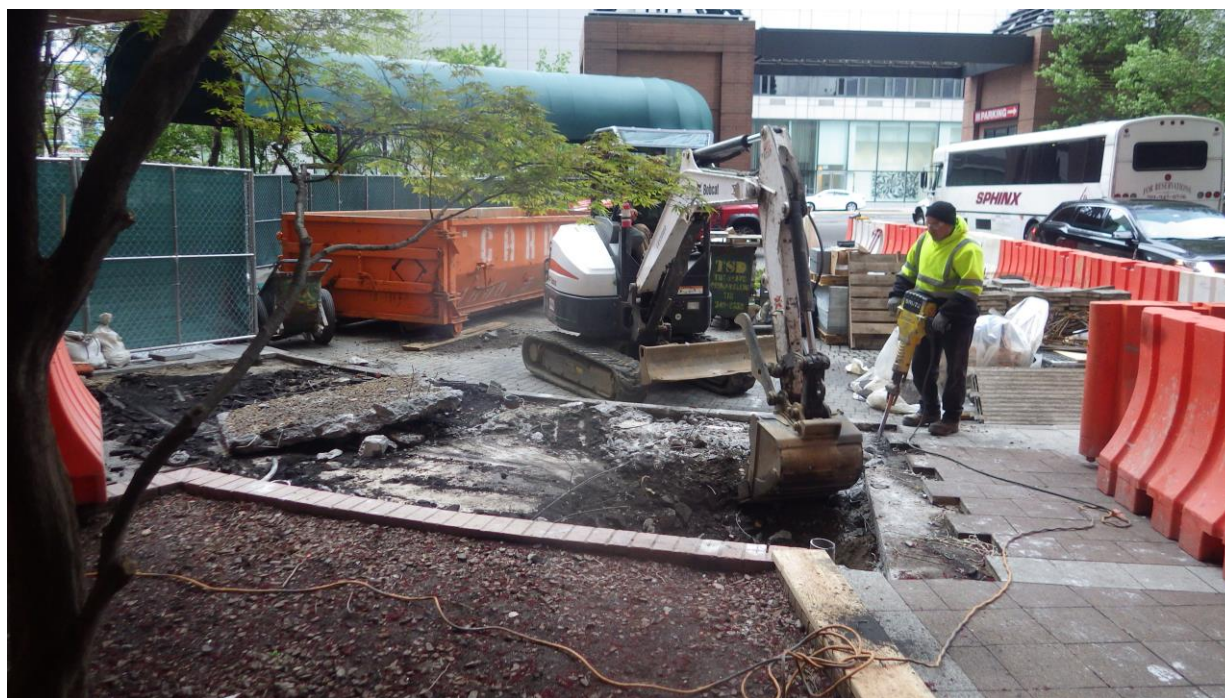
Photo 10: Excavation activity on the eastern portion of the Site; facing north. (05/05/2016)
