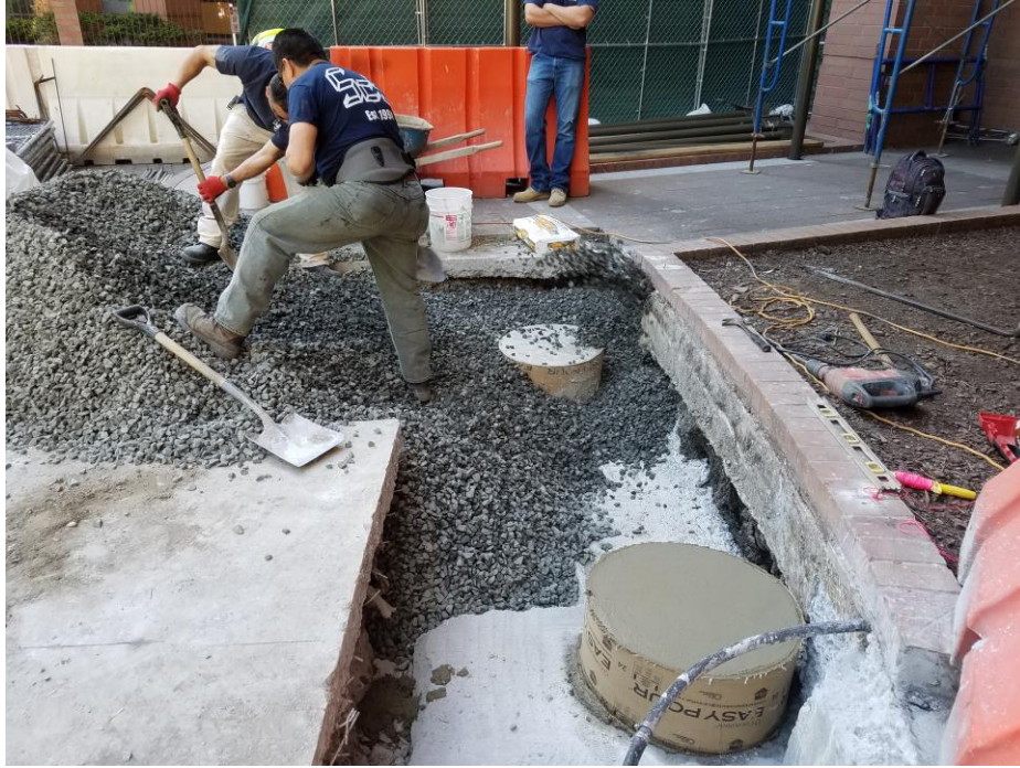
Photo 17: View of stone backfill in the eastern excavation area, facing southeast. (05/12/2016)
