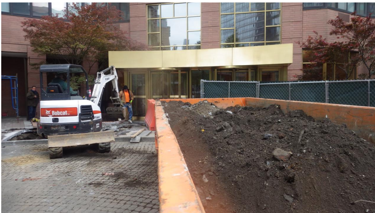
Photo 12: View of excavated material placed in a roll-off container for disposal; facing north. (05/05/2016)
