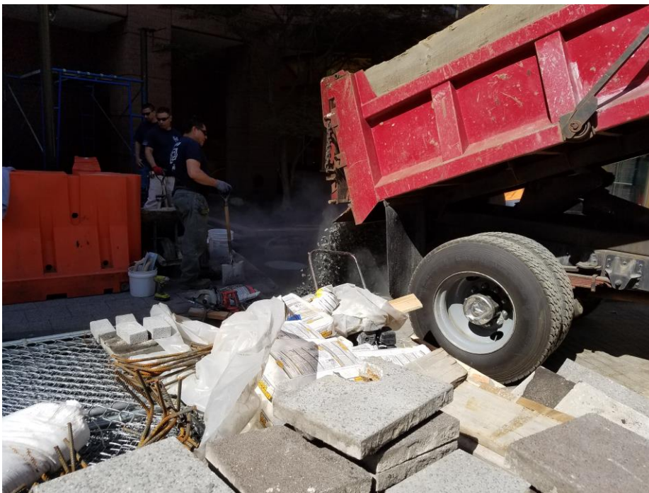
Photo 16: View backfill stone placement, facing south. (05/12/2016)
