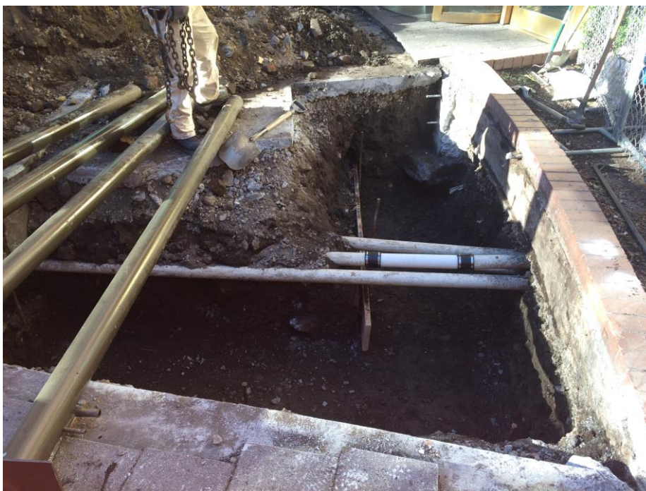
Photo 2: View of western excavation area; facing southeast. (4/21/2016)
