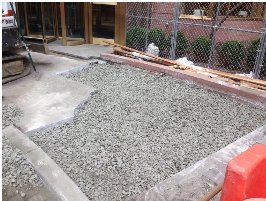
Photo 9: View of backfilled area on the western portion of the Site; facing south. (04/25/2016)
