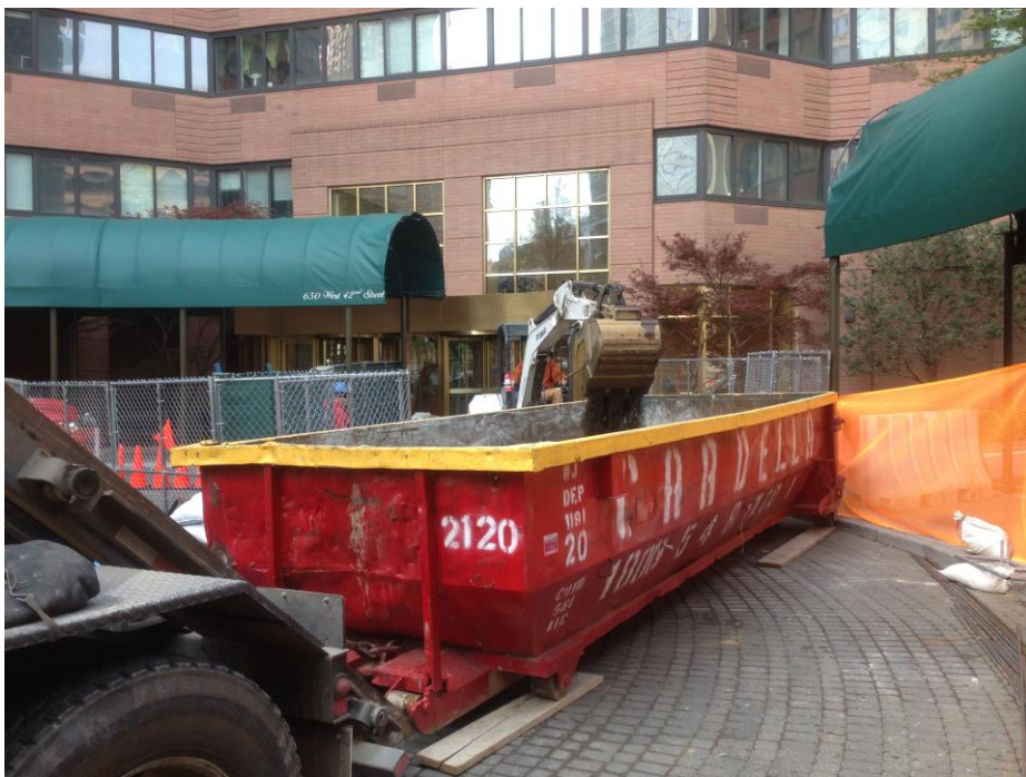
Photo 6: View of material loading and disposal activity; facing south. (04/25/2016)
