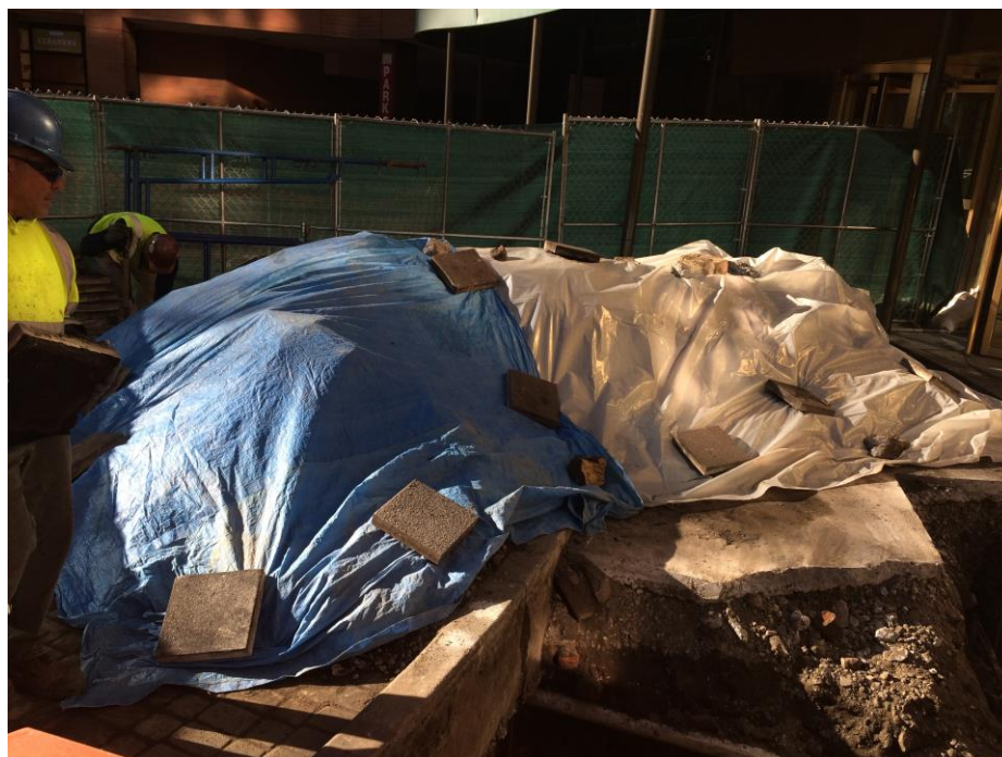
Photo 4: View of covered stockpile at end of work day; facing southeast. (4/21/2016)
