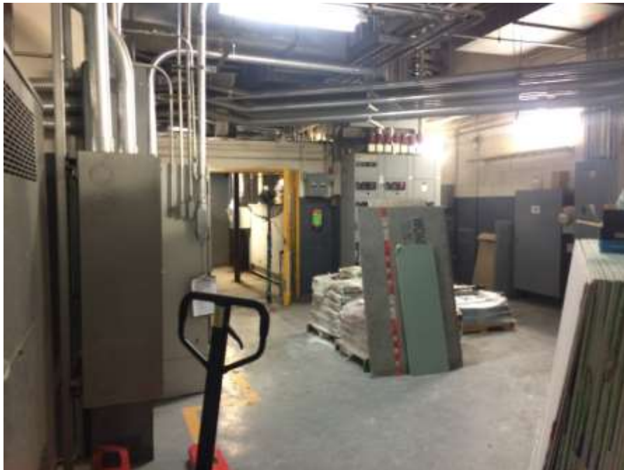
Photo 8: Surface cover in Site mechanical room
