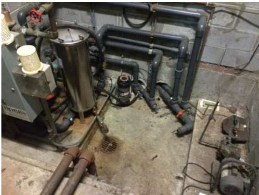
Photo 12: Surface cover in oil pump room
