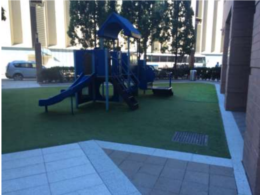
Photo 18: Location of repaired pavers and surface cover.
