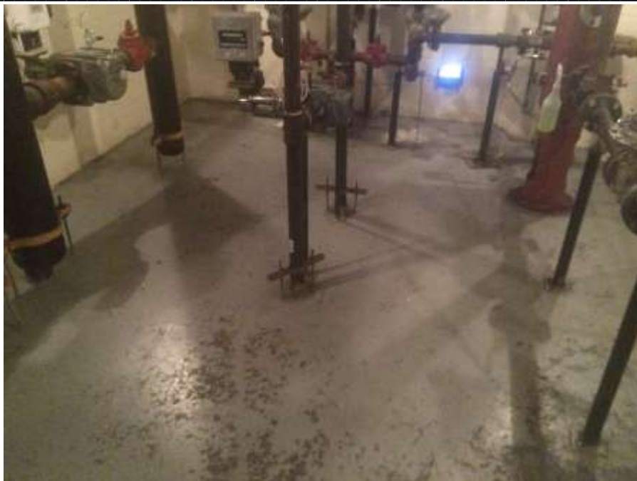
Photo 11: Surface cover in Site gas meter room.
