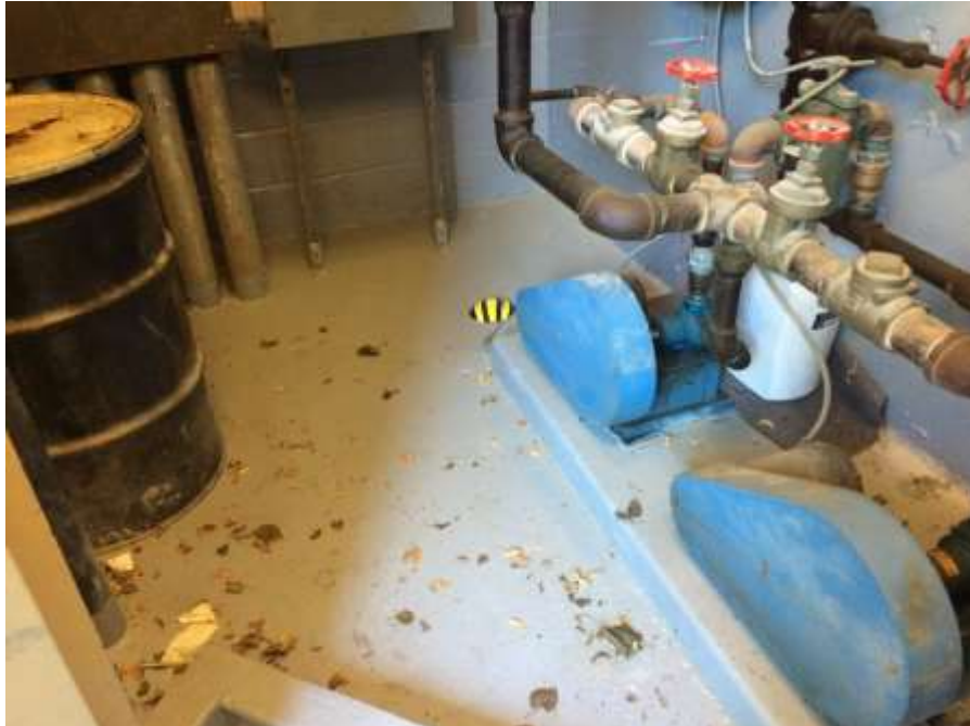
Photo 14: Surface cover in the Site oil pump room.
