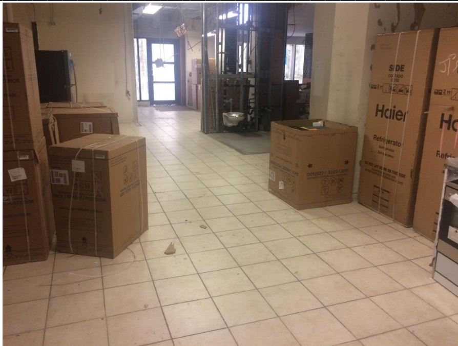
Photo 17: Surface cover at vacant commercial space within Site.
