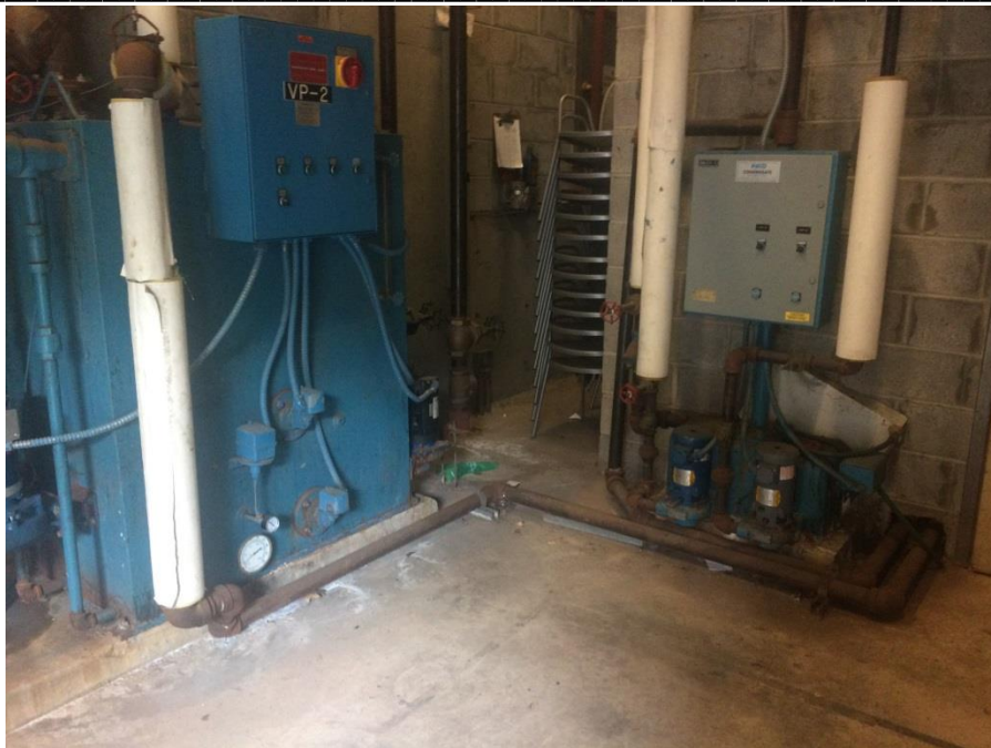
Photo 15: Surface cover in the Site oil pump room.
