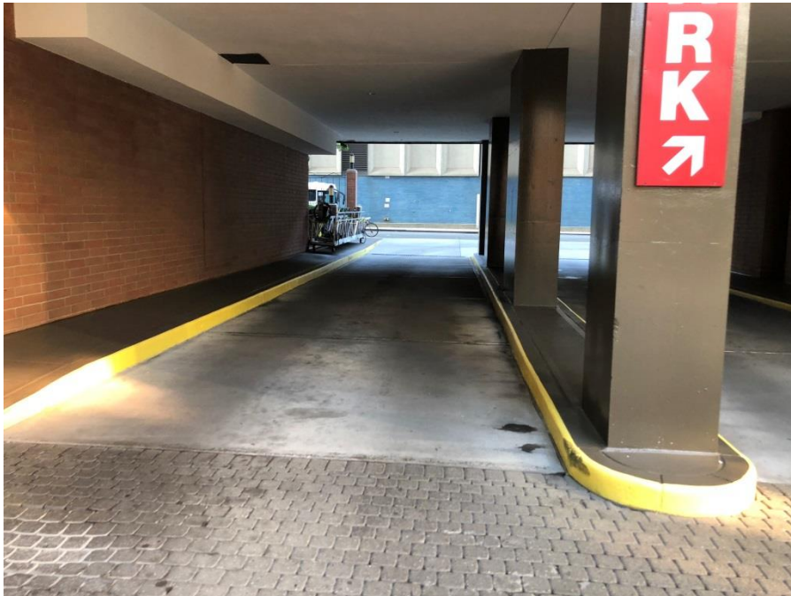
Photo 3: View of ground cover and roadway at the Site.
