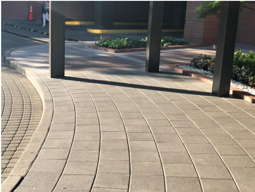
Photo 1: View of walkway at the Site.
