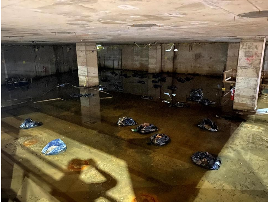
Photograph 3: Standing water from precipitation runoff in the central part of the cellar (facing northwest)
