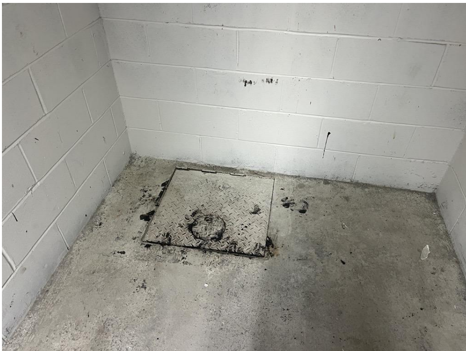
Photograph 8: Typical recovery well vault (RW-E, facing east).
