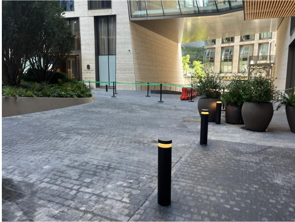
Photograph 9: Eastern building exterior (facing north).
